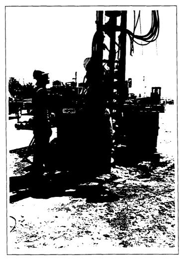
Photo 5: View to the southeast of L. Fluk at monitor well 3. She is driving out the pin from hollow flight extension in preparation to removing an auger flight from the drill stem. Photographer: Cora Halasan
