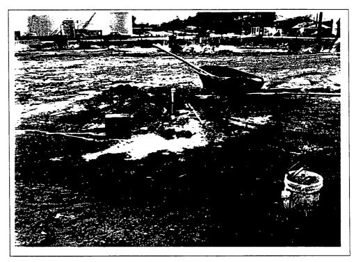
Photo 8: View east. Monitor well 3 is shown before final well completion. The thick clayey sediments and dark brown soils to the left of the PVC well casing are drill cuttings. This photo also shows the compacted contaminated surface sediments at this location. The active Giant Refining tank farm is in the left background, across Fifth Street. Photographer: Cora Halasan
