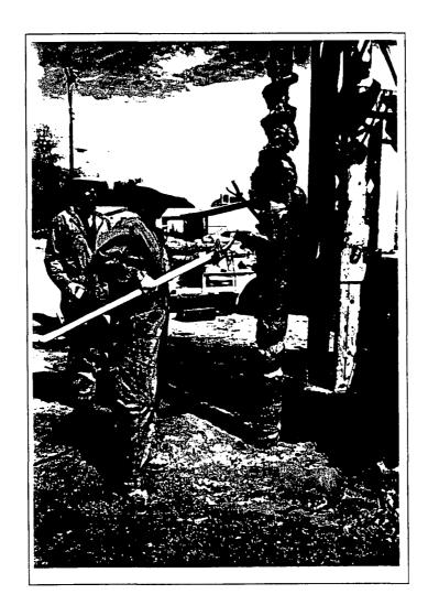
Photo 6: View west. L. Fluk & M. Sanders, at monitor well 3, removing thick wet clay from auger flights during the final withdrawal of the drill stem from the borehole. Note the contaminated sediments and oily water around the hole. Photographer: Cora Halasan
