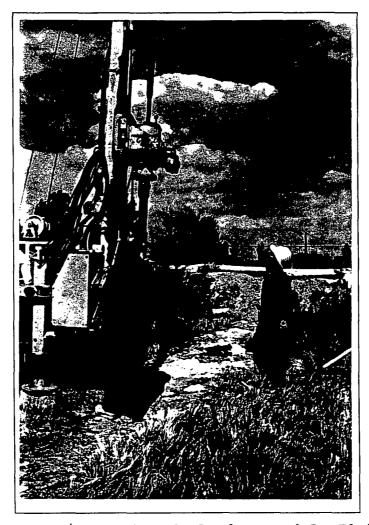
Photo 3: View west. M. Sanders and L. Fluk, at monitor well 2, are lowering the split spoon sampler down the hollow-stem auger. The raised concrete slab in the right background is one of the building foundations located at the south end of the property. Photographer: Cora Halasan
