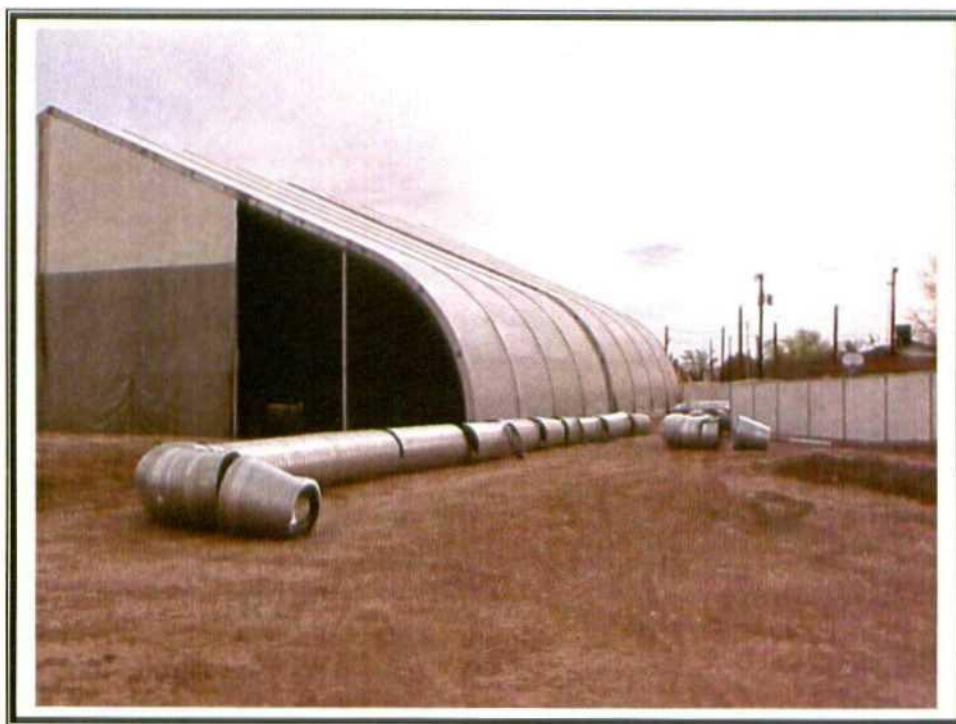
13. One structure panel left to be installed. Duct work for carbon filtration system is being assembled.
