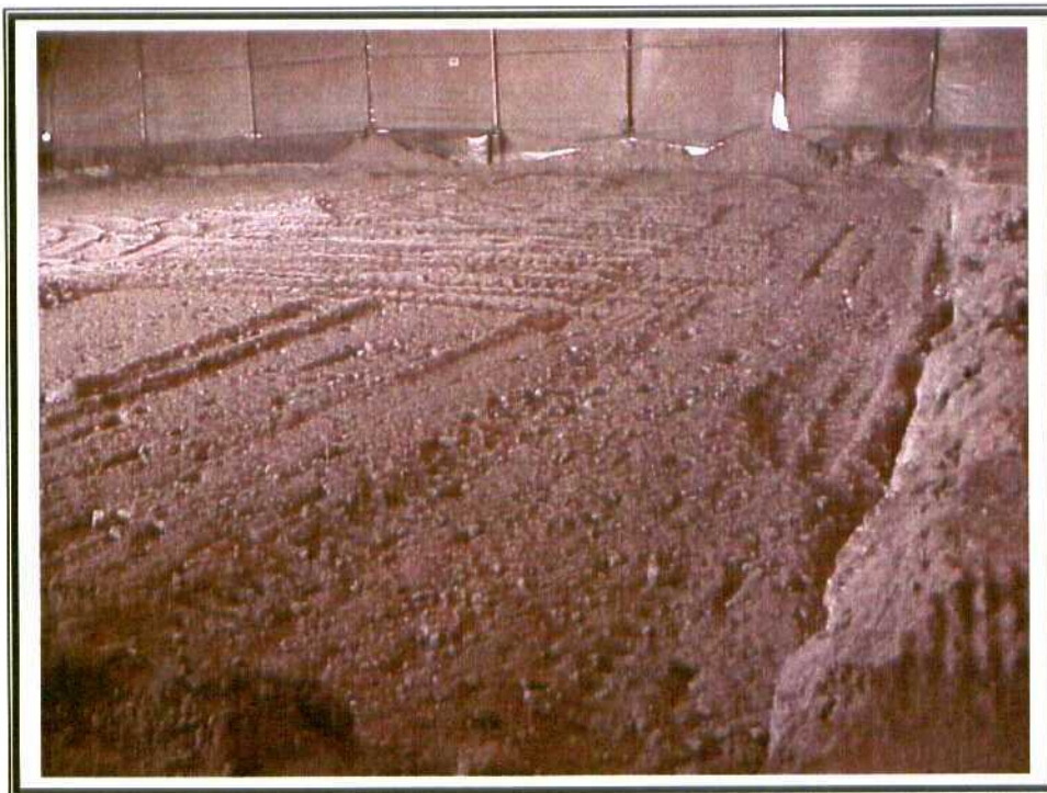
32. Phase III – Backfill caliche near surface.
