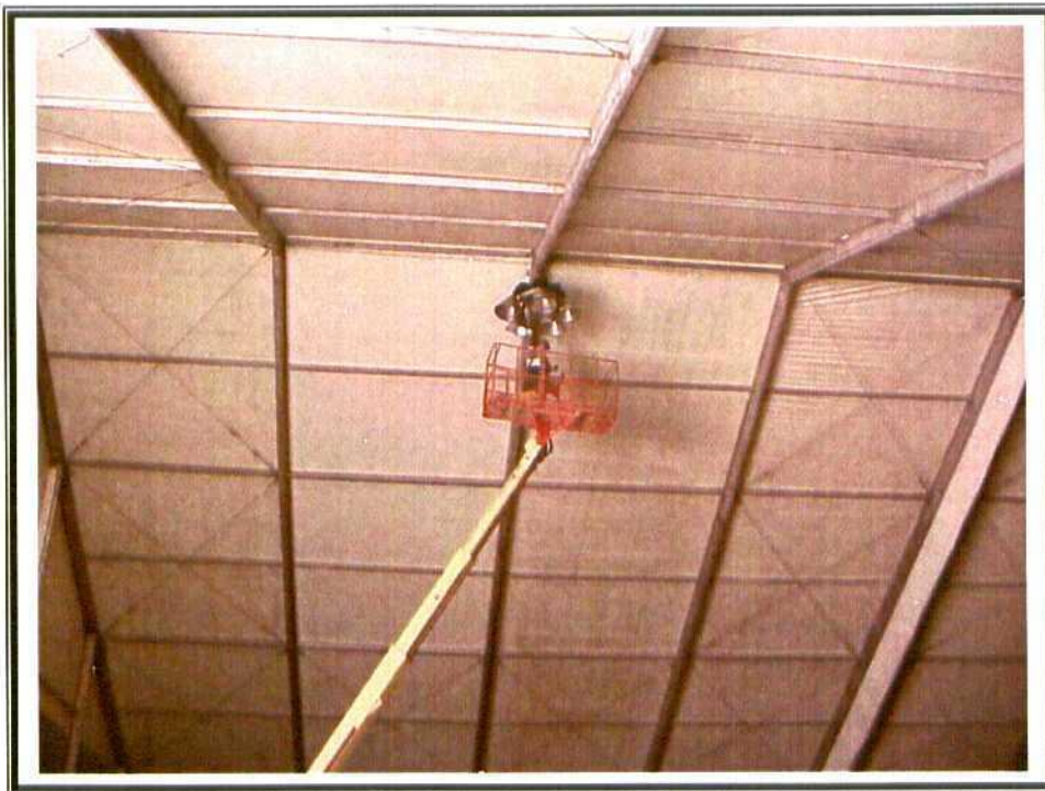
4. Electrician wiring structure lighting.
