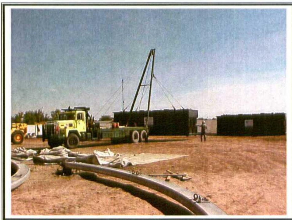
25. Winch truck loading carbon beds onto carrier truck.
