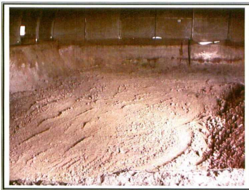
23. Phase III – Excavation – bottom hole.
