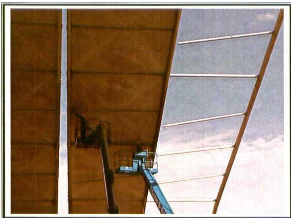
14. Structure crewman detaching crossbeams from the last ribs still standing.
