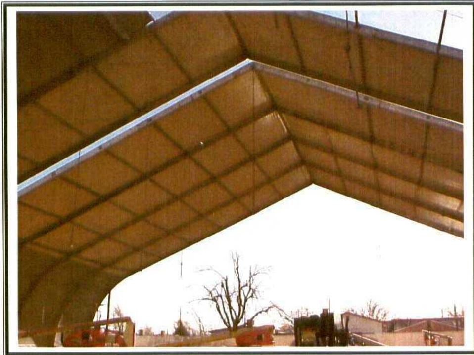
3. View from inside of structure.
