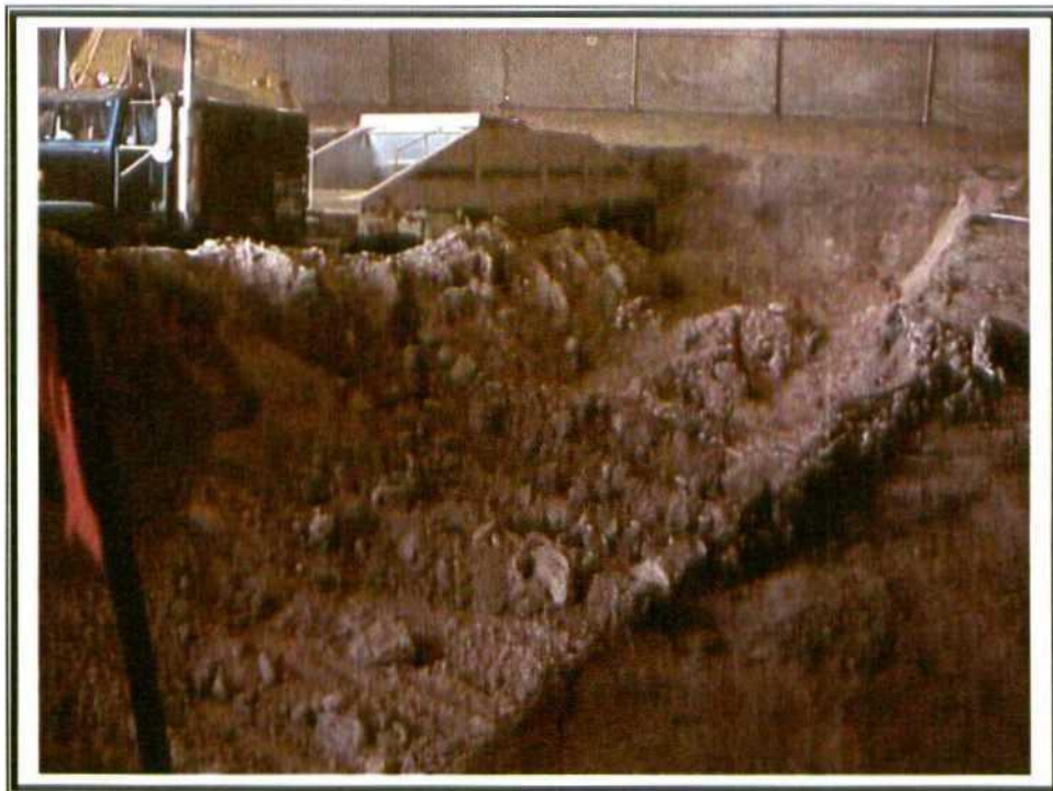
18. Phase II Excavation. Dump truck backed into structure to load up soil.
