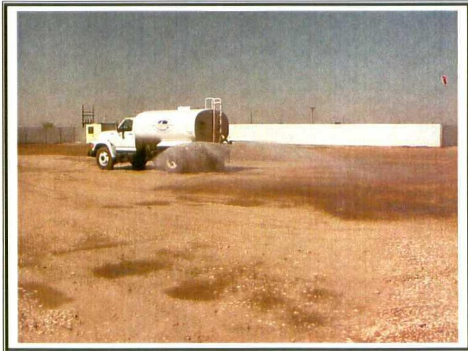
33. Phase I – Backfilling. Watering site to minimize dust.
