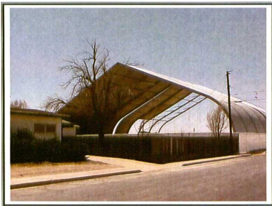
8. Rear view of structure from San Andres.
