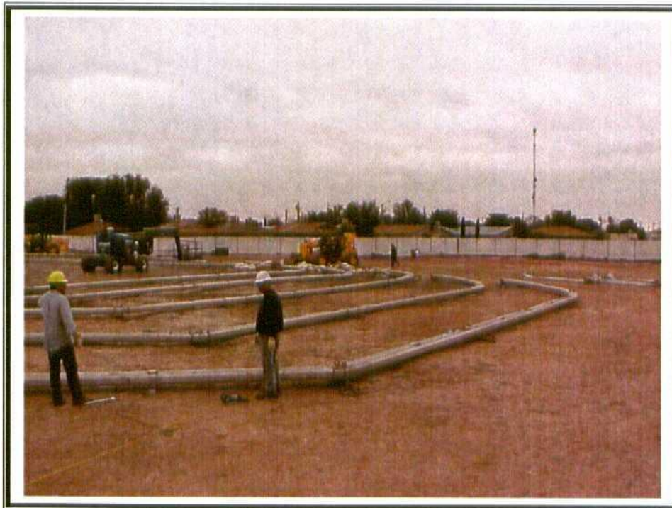
20. Structure crewmen disassemble structure framework.
