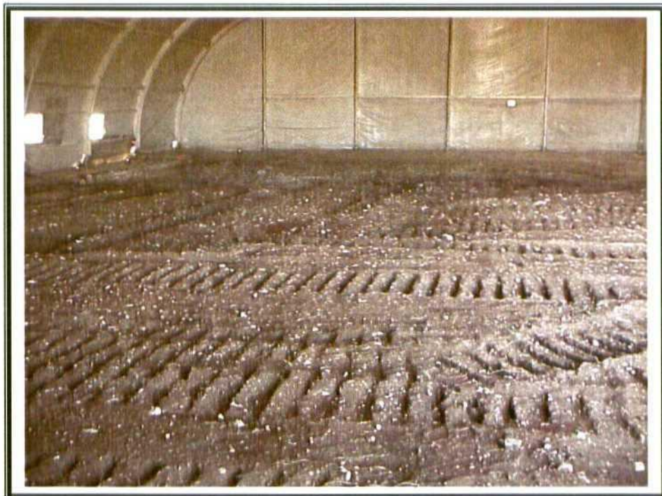
28. Phase II – Backfill almost completed.
