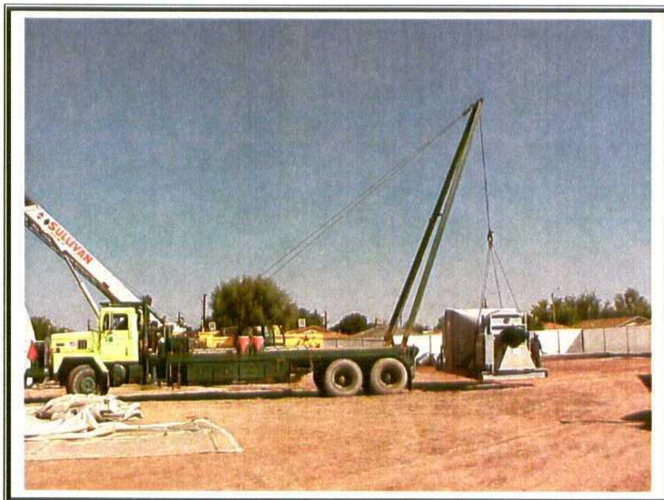
24. Winch truck loading carbon filtration unit on carrier truck.
