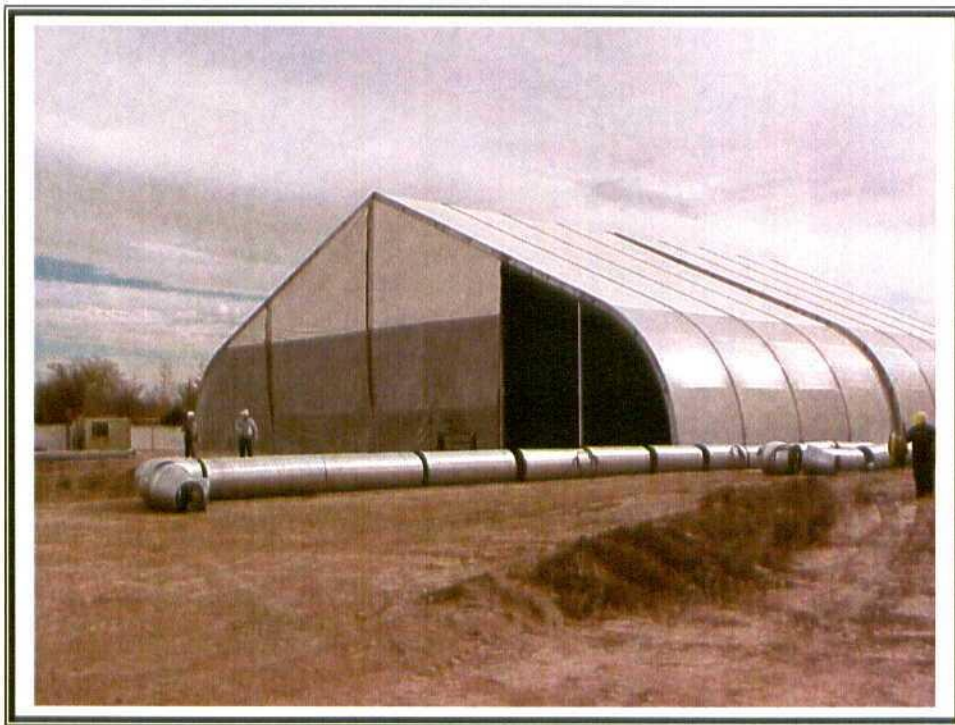
14. Assembling duct work for carbon filtration system.
