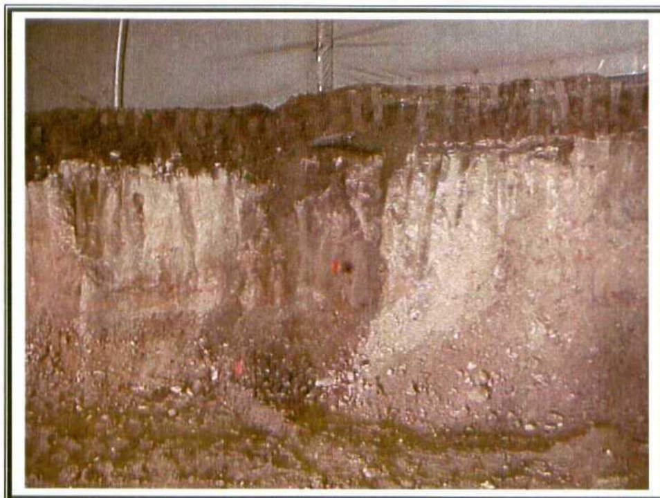
18. Phase I – Confirmation Sampling. Orange flag marks sample points on east wall and one at ground level.
