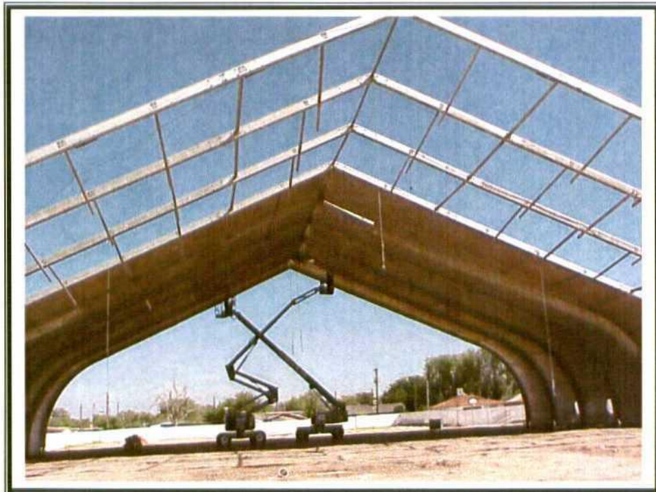
13. Front view of structure with fabric removed.
