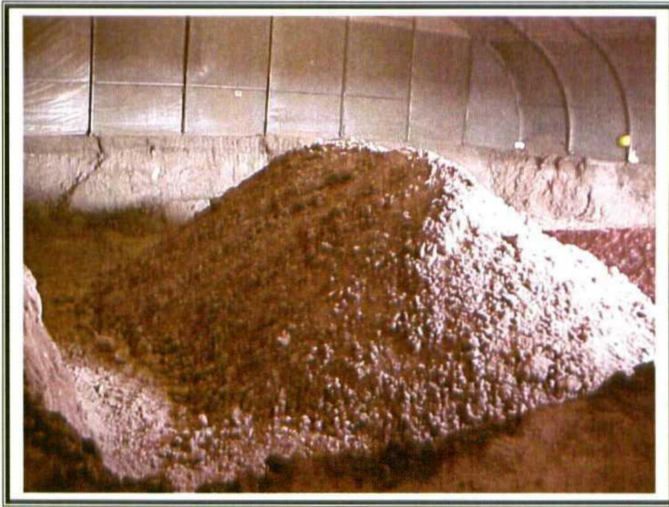
20. Phase III – Excavation.
