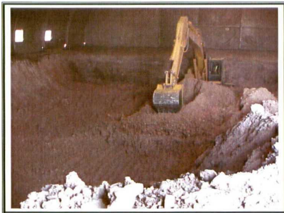
20. Phase II Excavation. Excavator piling up soil to be loaded into dump trucks.
