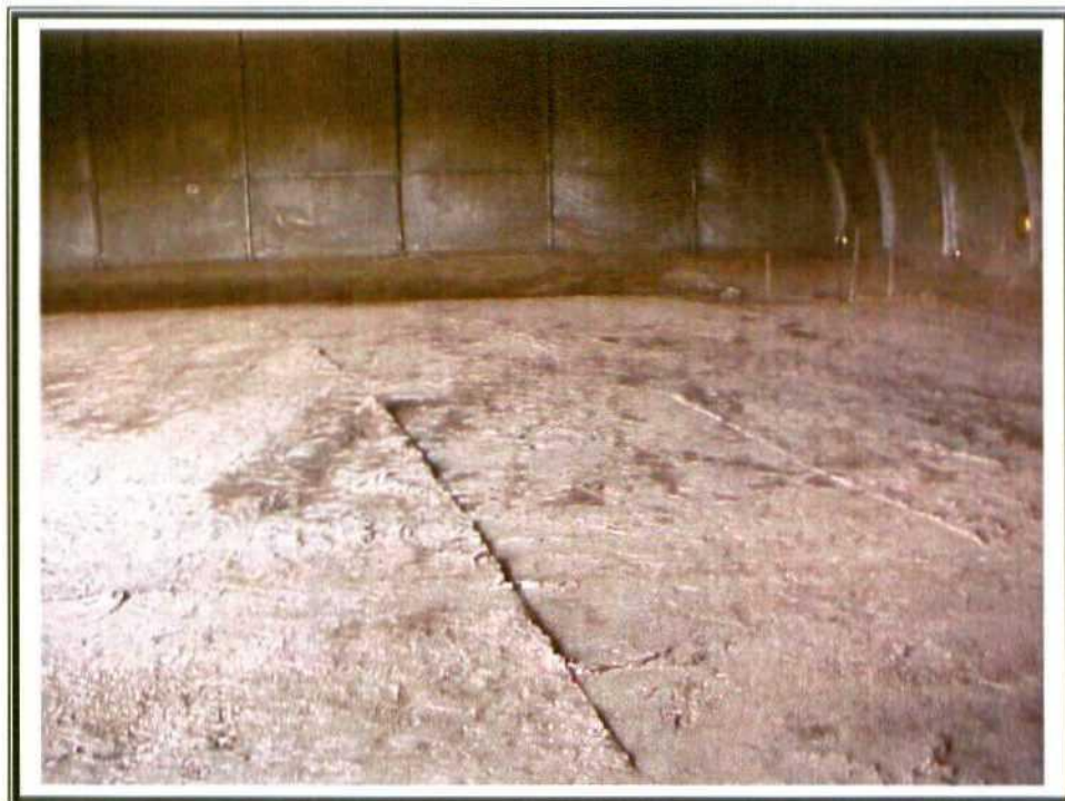
30. Phase II – Backfill completed and leveled.
