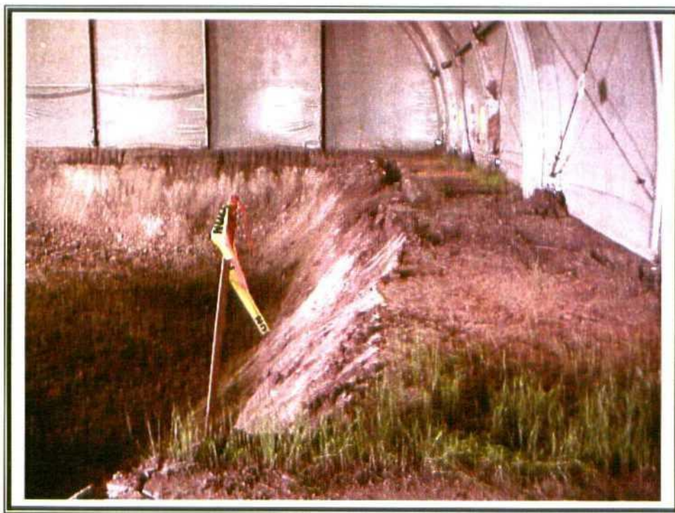
9. Phase I Excavation
