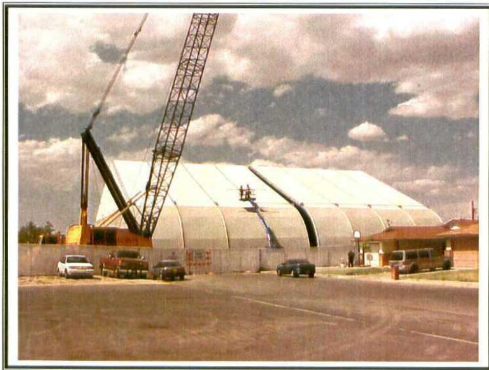
5. Universal Fabric Structure crewman securing support beams in preparation for structure move.
