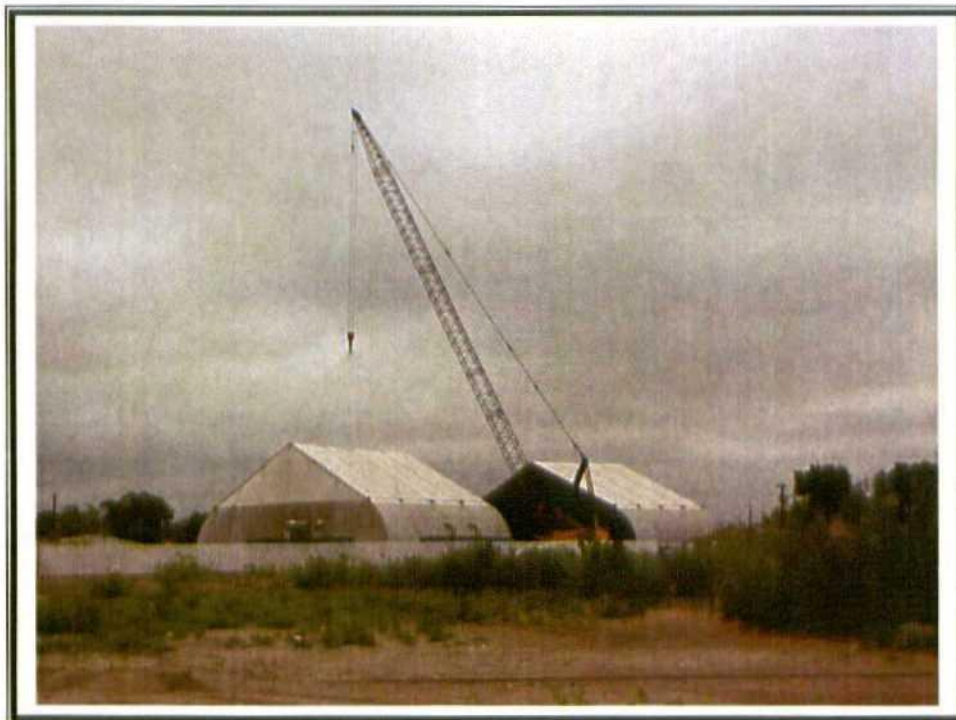
10. View from a nearby field of the structure move.
