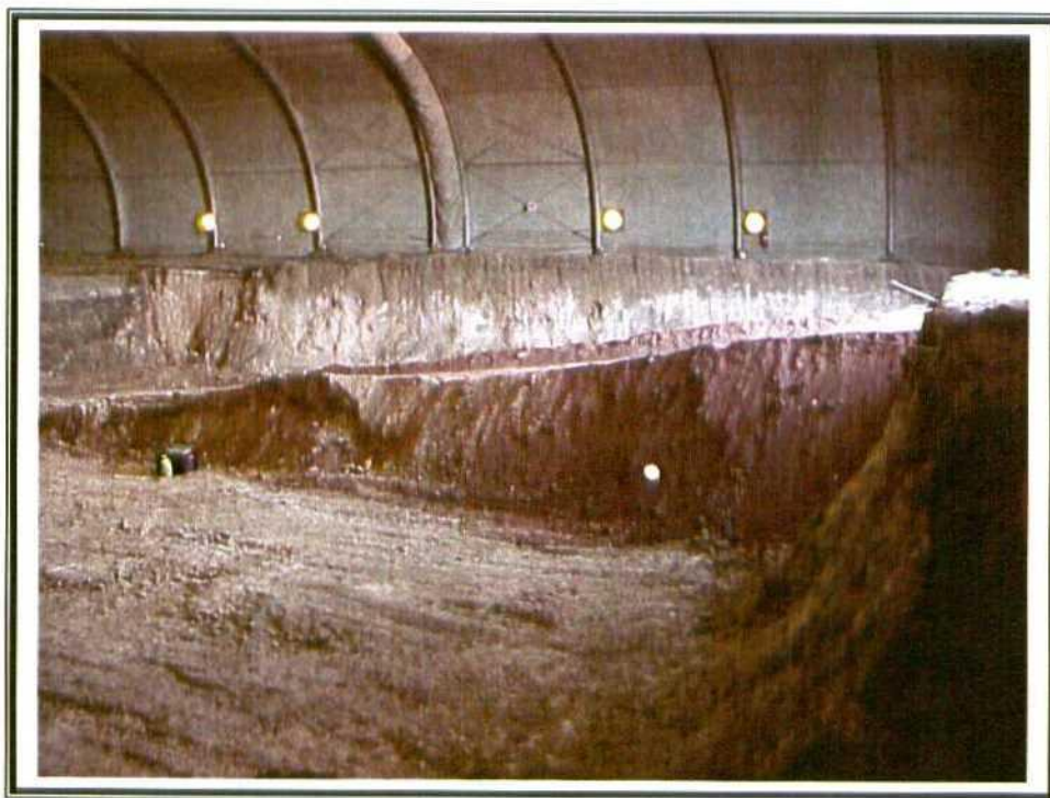
21. Phase II Excavation – bottom hole.
