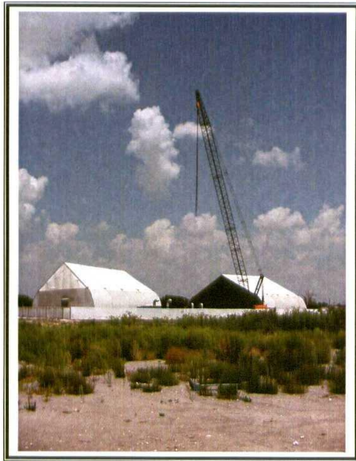
11. View of crane and structure move from nearby field.
