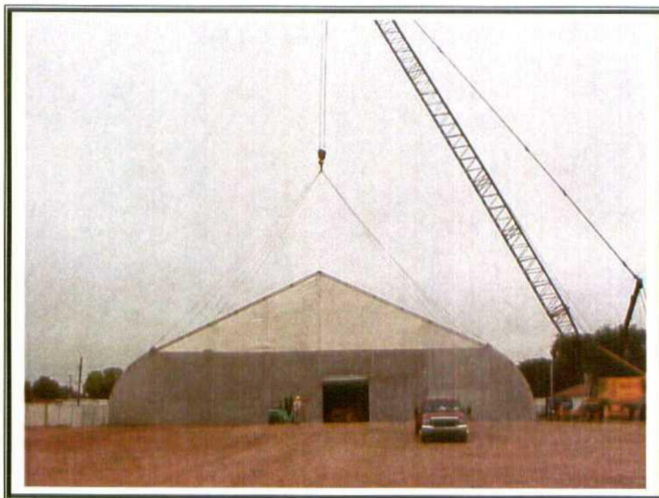
6. Rigging up crane cables to lift structure.
