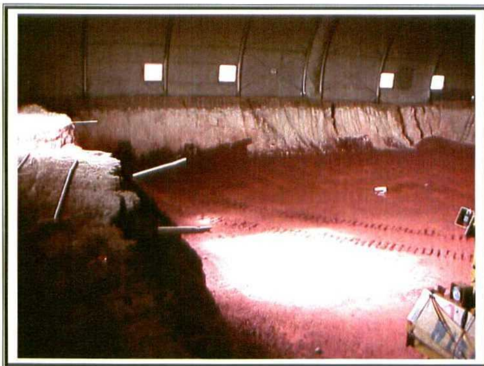
26. Phase II – Backfill clay liner.
