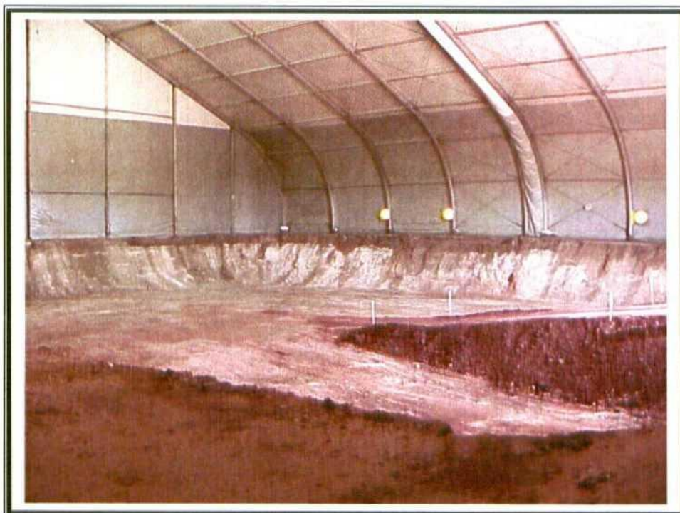
16. Phase I Excavation – Bottom hole and clay ramp
