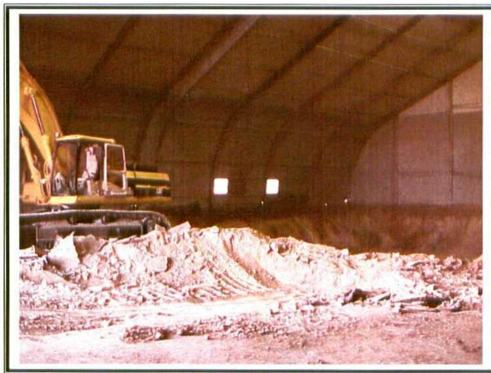
3. Phase I Excavation
