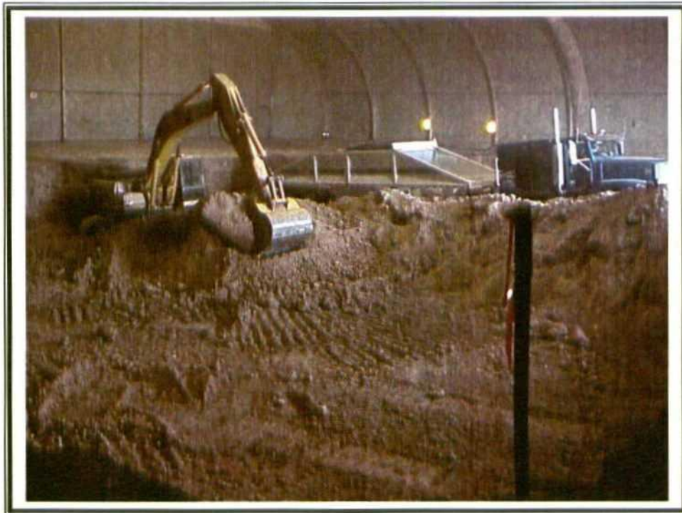
19. Phase II Excavation. Excavator loading up dump truck.
