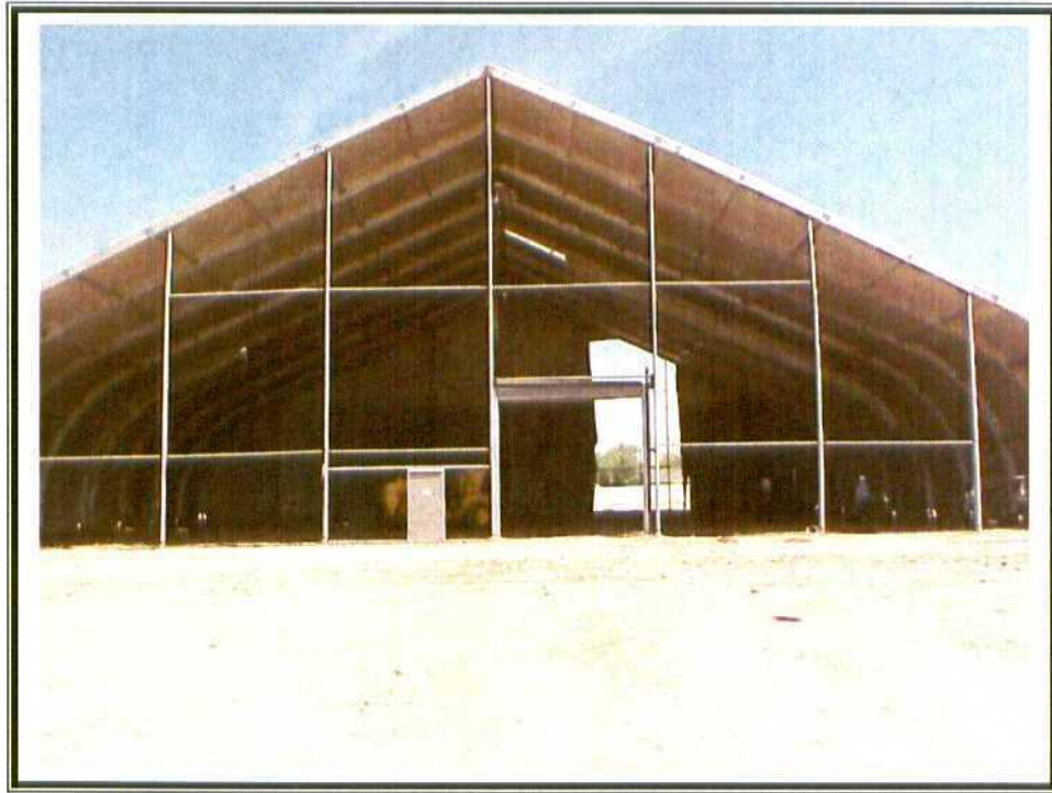
9. Front view of structure without fabric panels.
