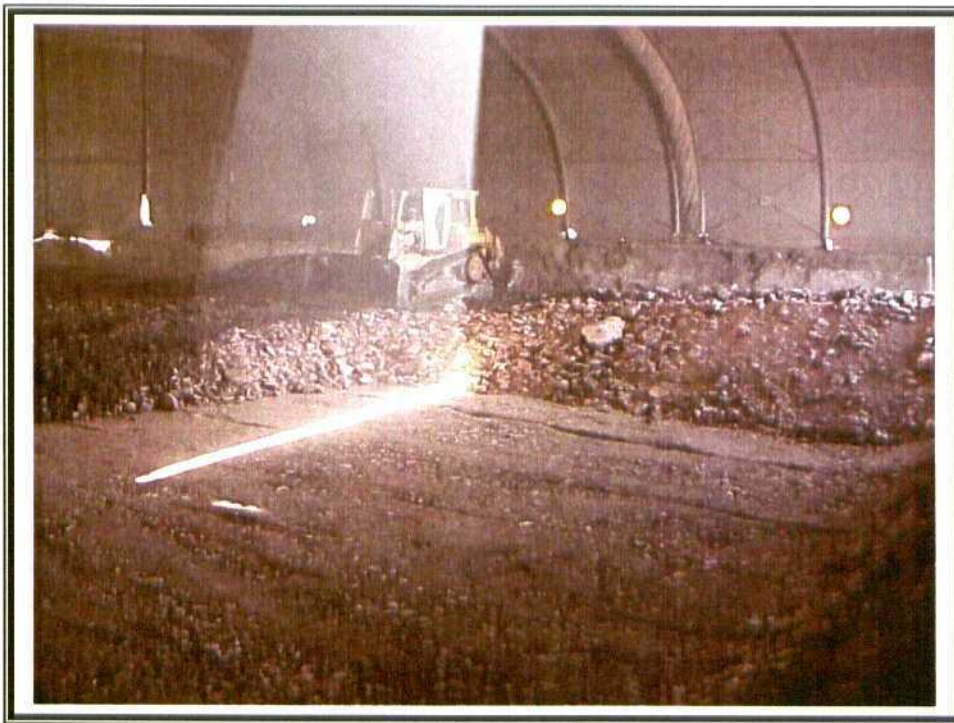
31. Phase III – Backfill. Dozer spreading caliche.
