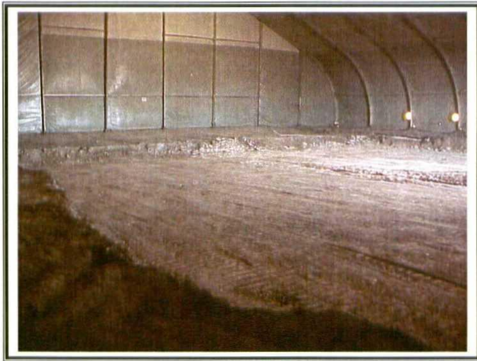
29. Phase II – Backfill at final stage with topsoil.
