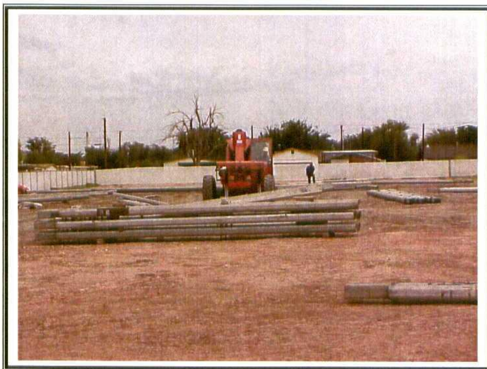
22. Framework stacked in piles.
