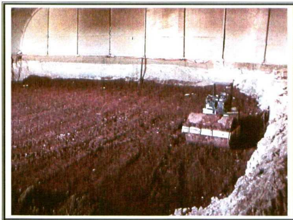
29. Phase III – Backfill. Roller packing down clay liner.
