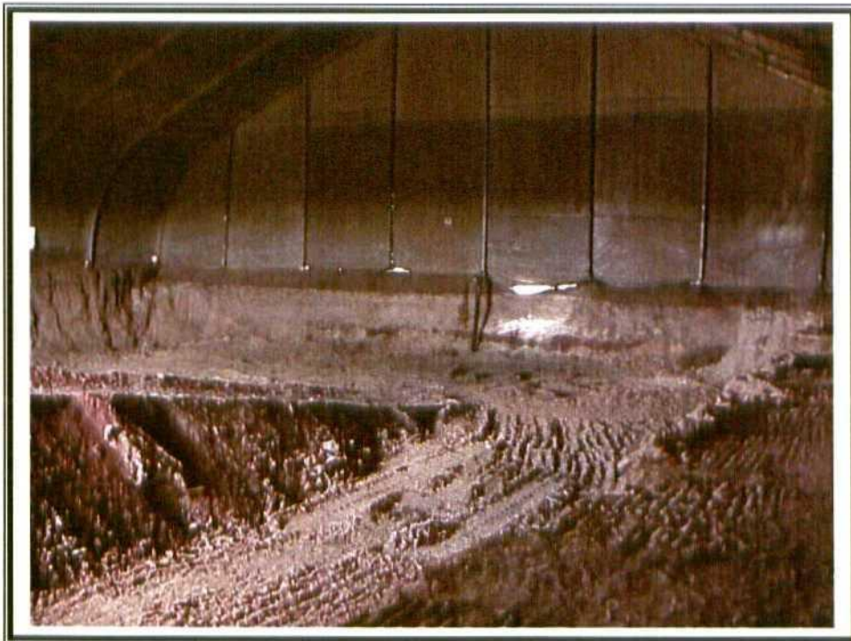
21. Phase III – Excavation.
