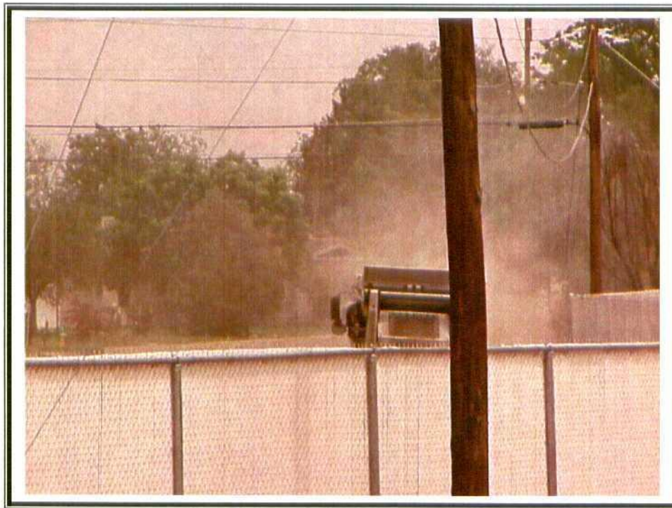
32. Phase I – Backfilling. City of Hobbs street sweeper off site on Berry Drive.
