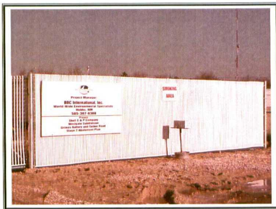
19. Project identification sign at site entrance and designated smoking area.
