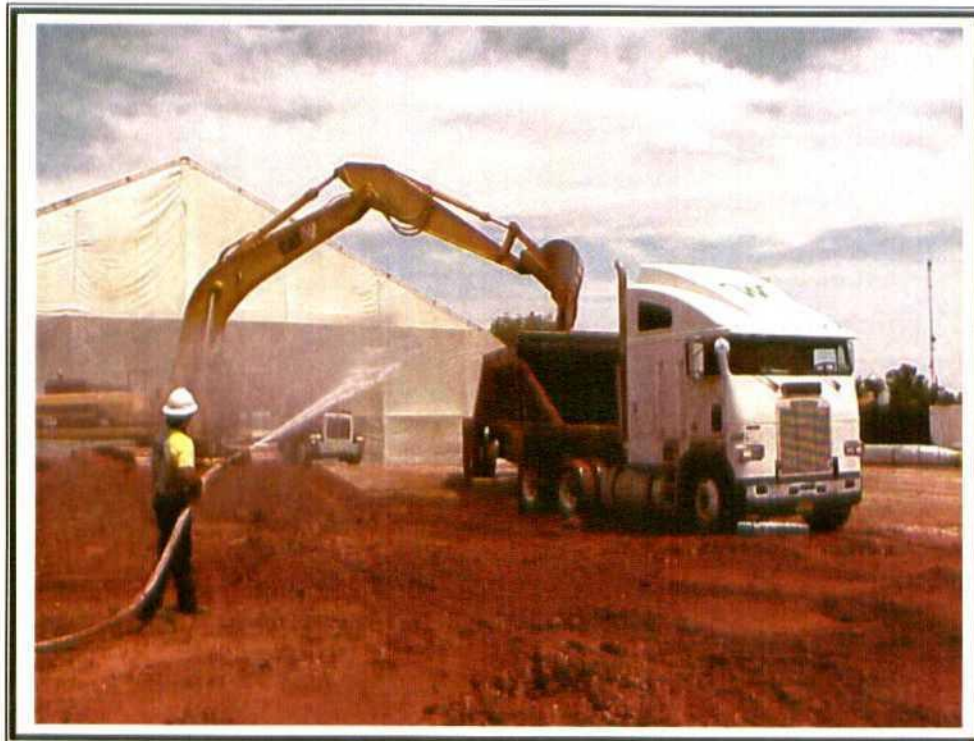
24. Phase I – Backfilling. Watering down clay to minimize dust.
