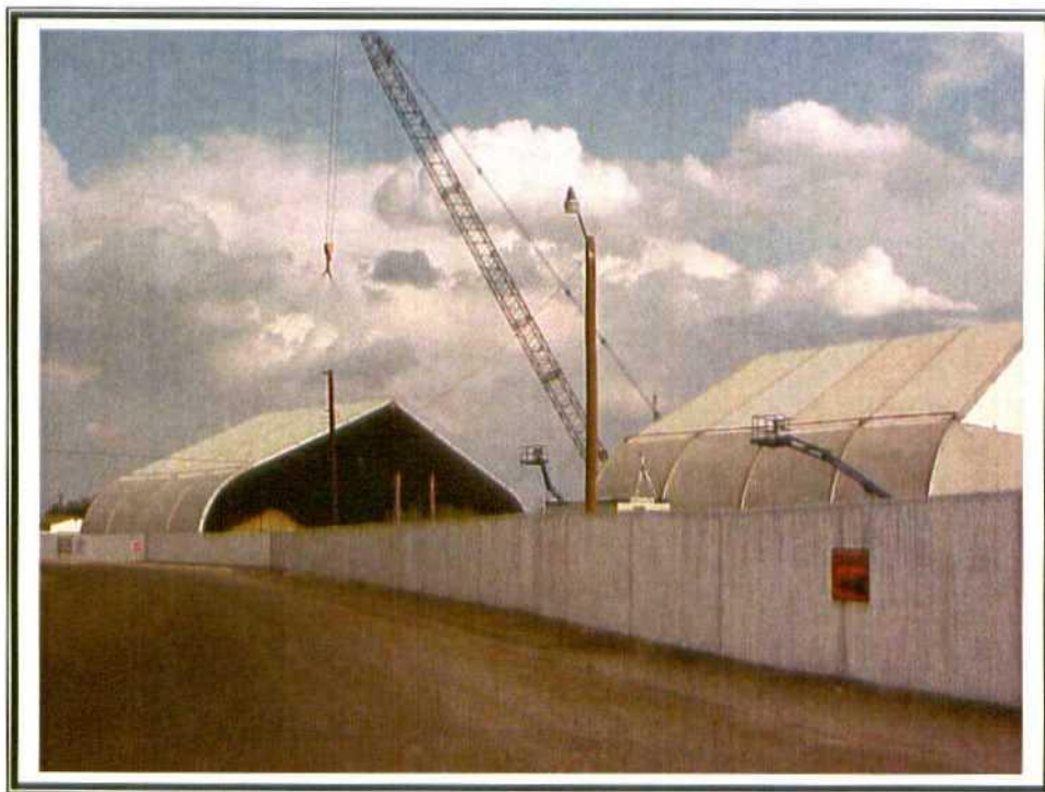
12. View of structure move from the corner of Cobb Street.
