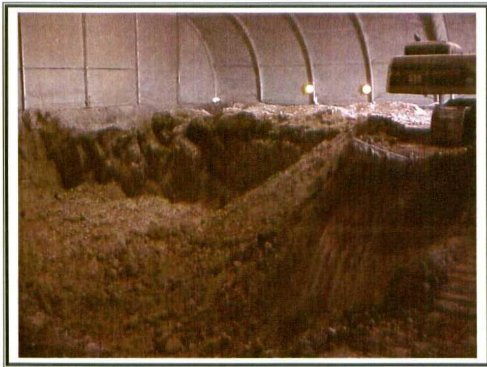
17. Phase III – Excavation.
