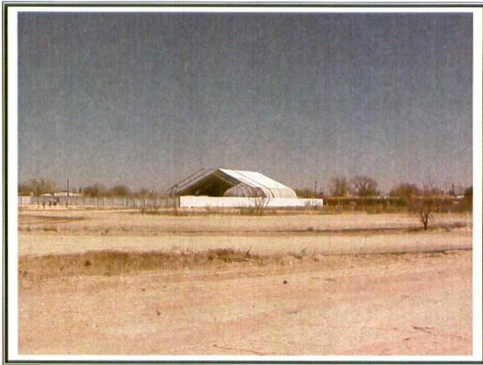
10. View of structure from nearby field.
