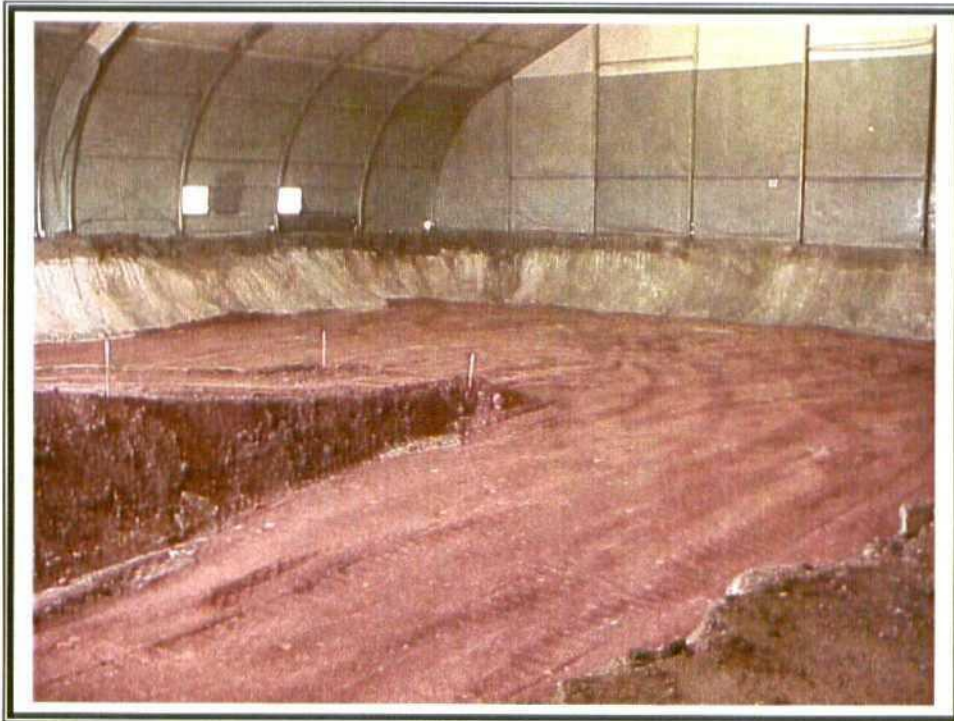
23. Phase I – Backfilling. Clay liner.
