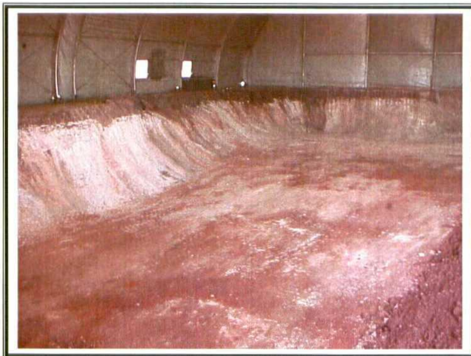
15. Phase I Excavation – Bottom hole
