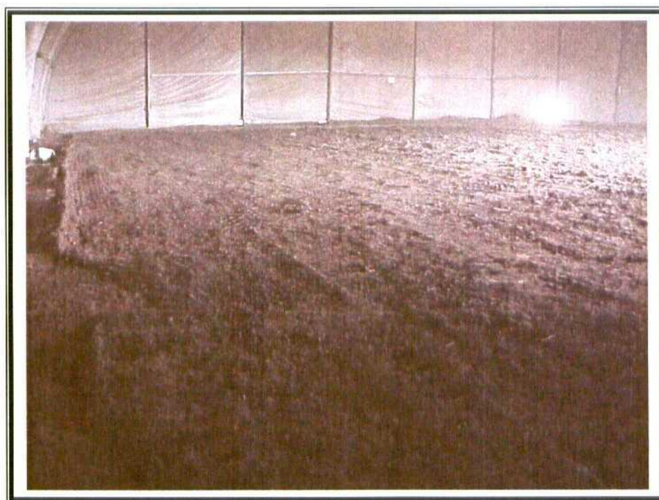
35. Phase III – Backfill topsoil.
