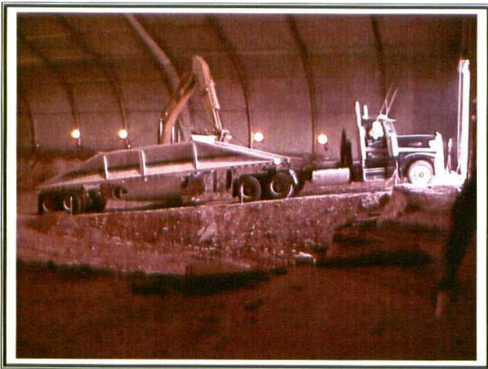
12. Phase I Excavation – ramp used to back into structure
