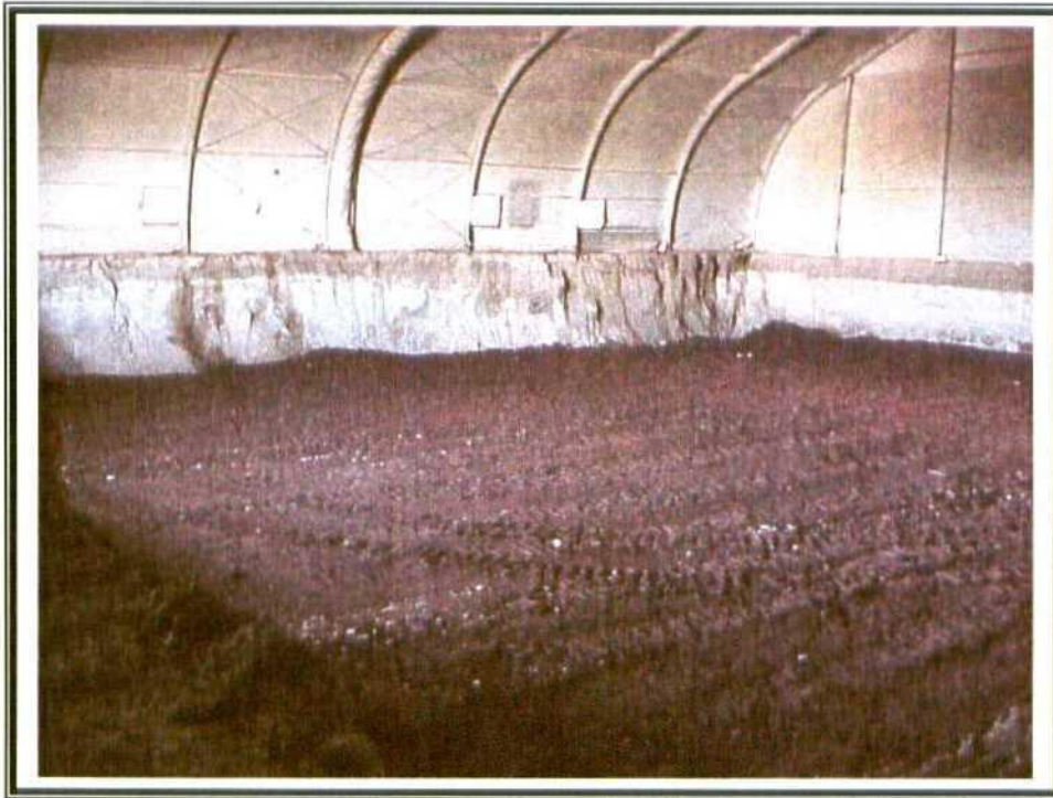
28. Phase III – Backfill. Clay liner.
