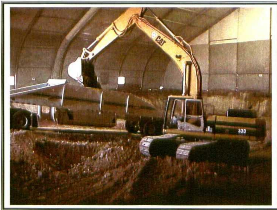
13. Phase I Excavation – Excavator loading dump truck
