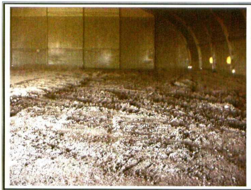
30. Phase I – Backfilling. Final stage of backfill (topsoil).
