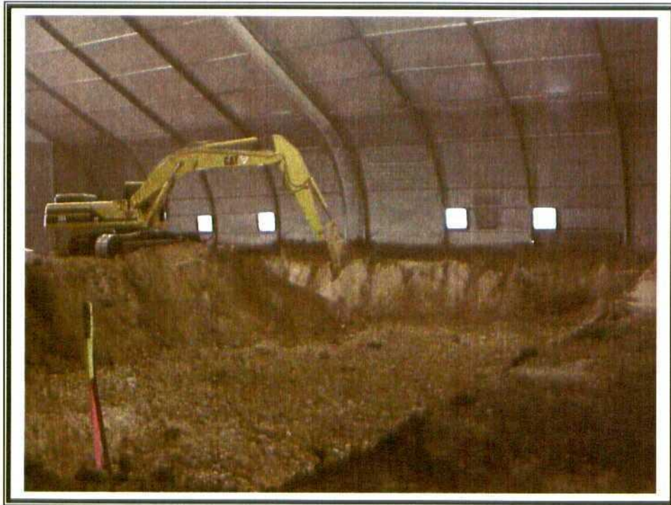
5. Phase I Excavation
