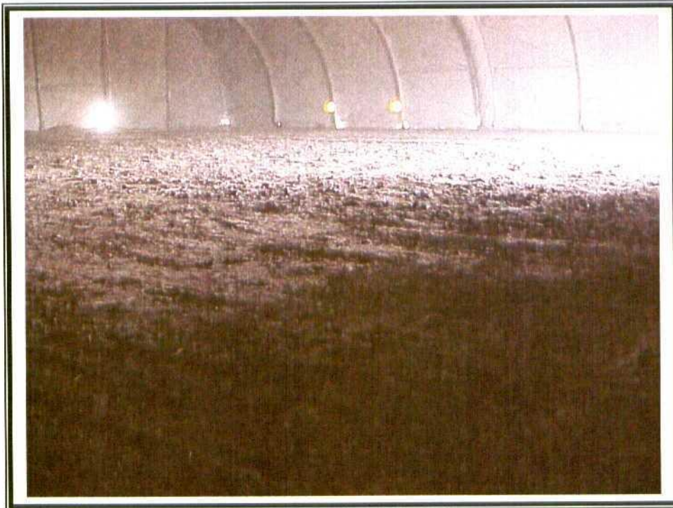
36. Phase III – Backfill topsoil.
