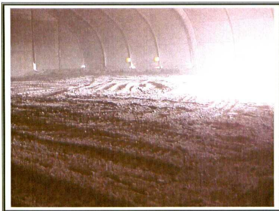
34. Phase III – Backfill topsoil.
