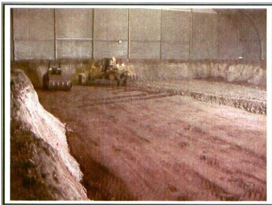
28. Phase I – Backfilling. Dozer and vibratory roller spreading caliche backfill.
