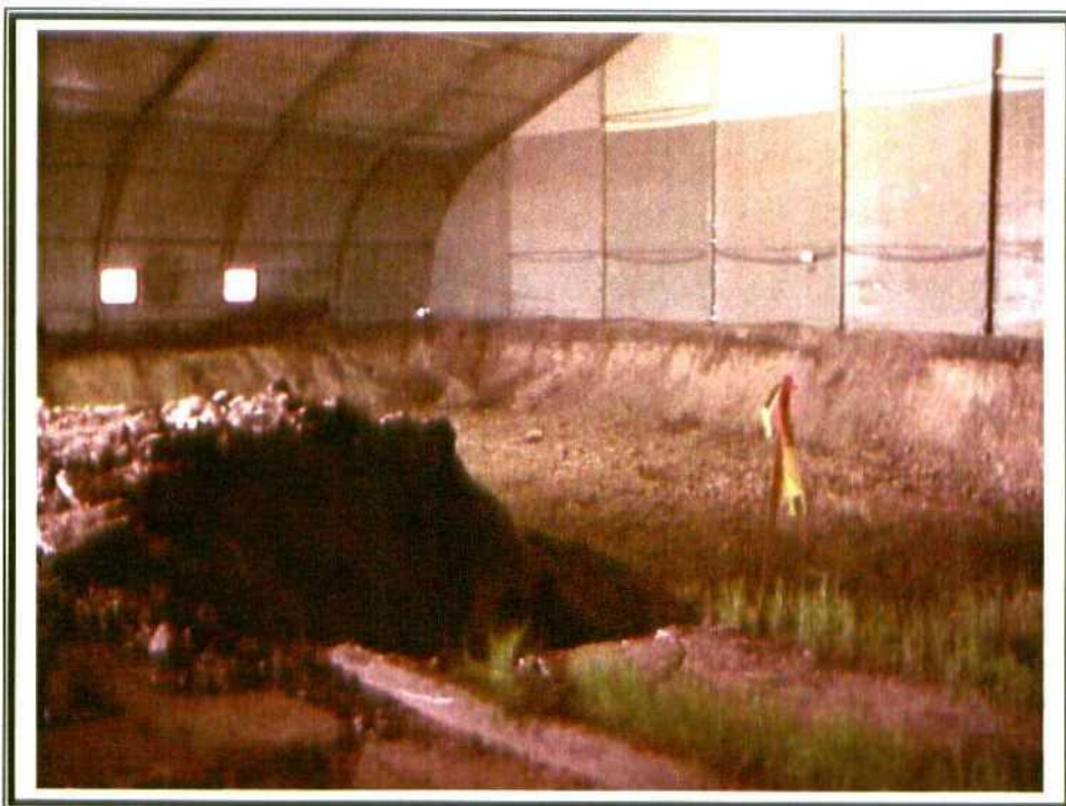
10. Phase I Excavation
