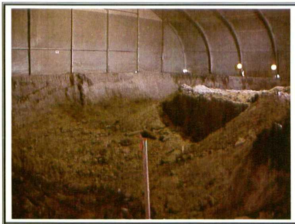
19. Phase III – Excavation.
