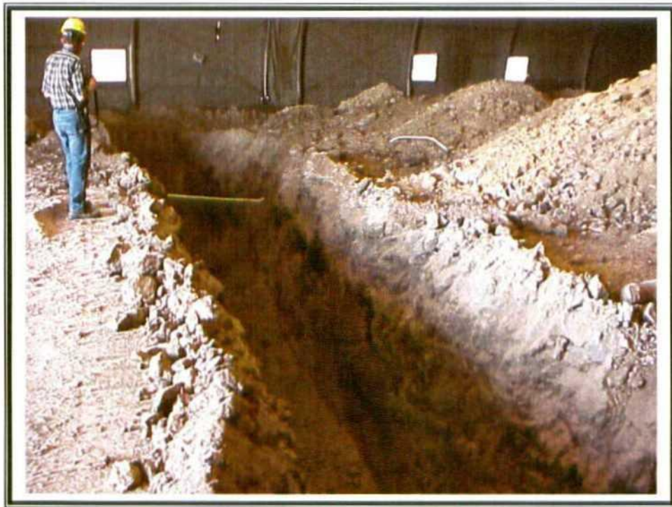
17. Phase II Excavation.
