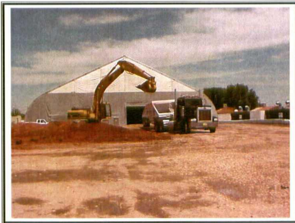
25. Phase I – Backfilling. Truck loading up clay to dump inside structure for clay liner.
