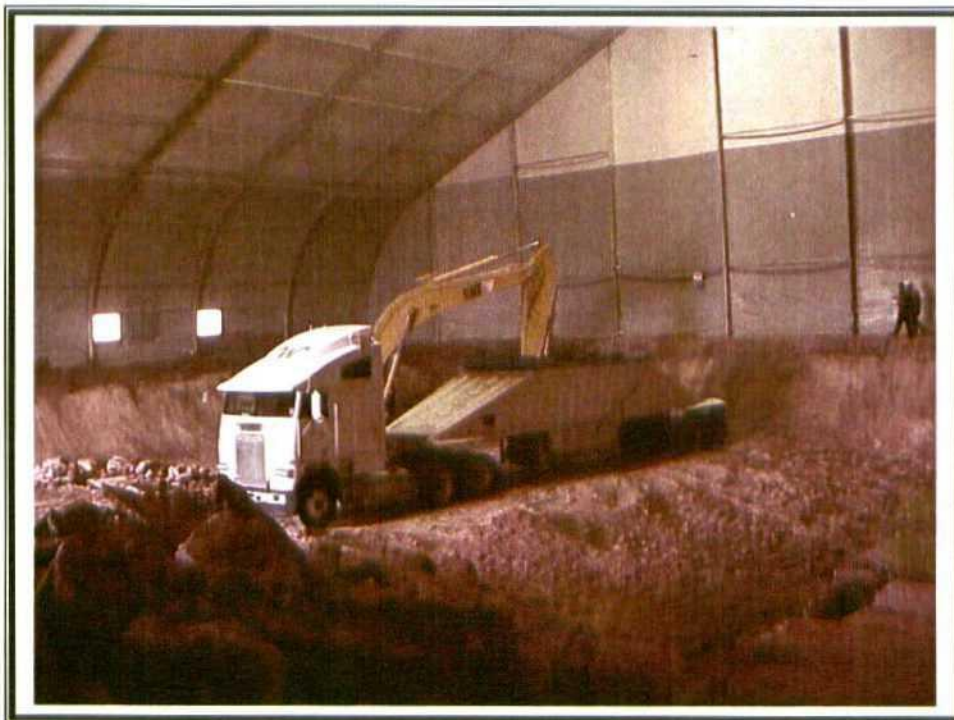
14. Phase I Excavation – Dump truck loading at bottom of excavated area
