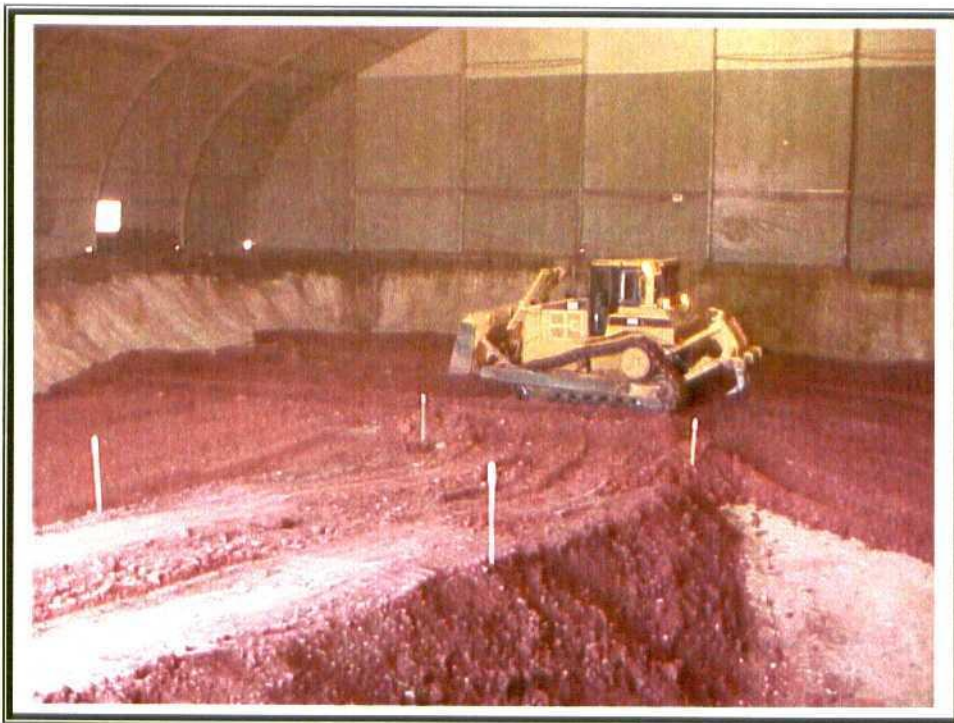
22. Phase I – Backfilling. Dozer leveling clay liner.
