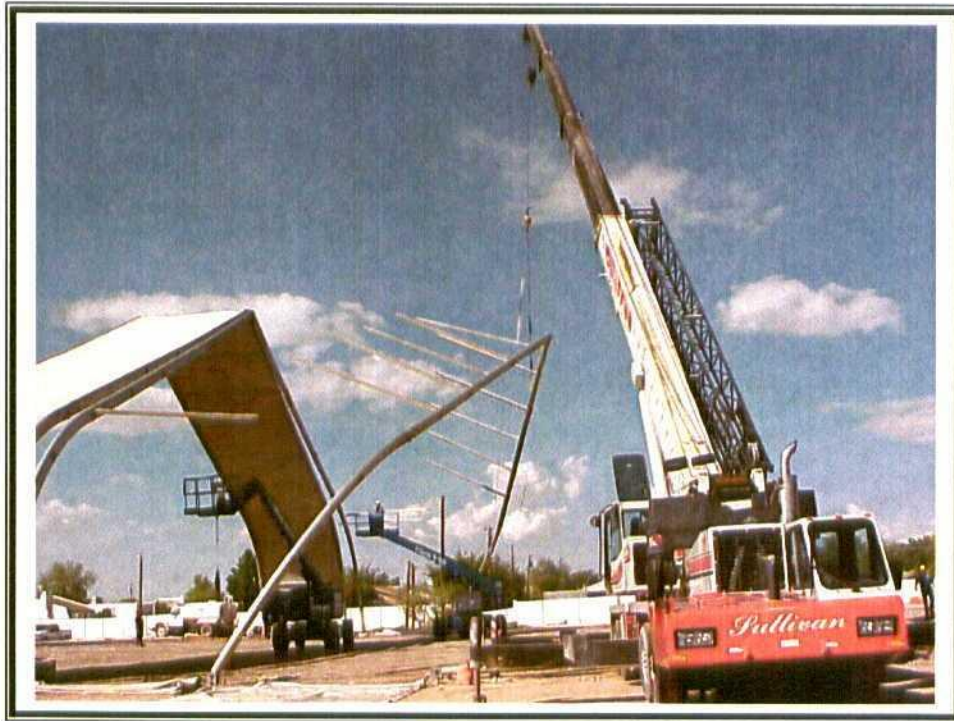
17. Crane lowering a rib of structure framework.
