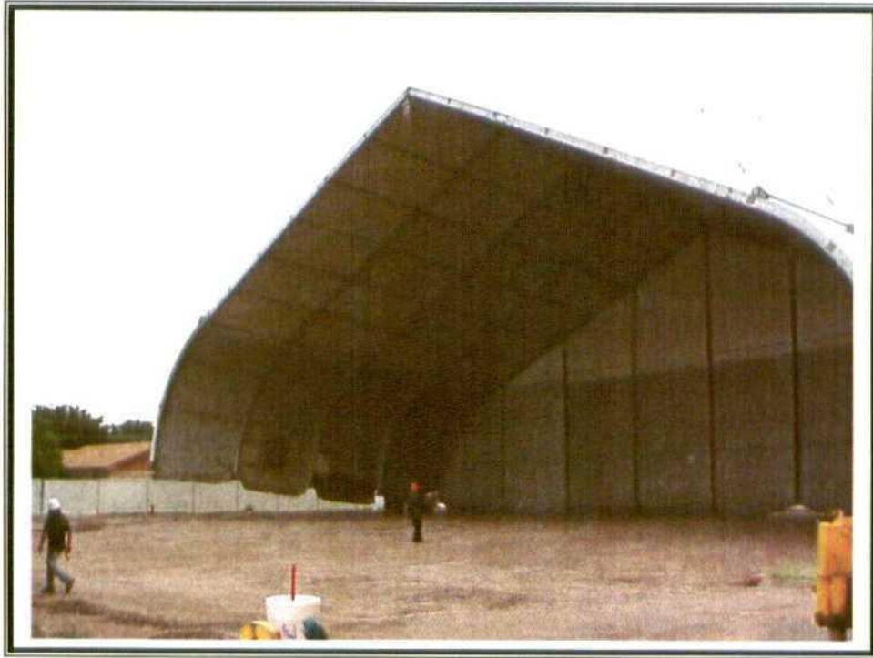
11. Lifting and moving back half of structure.
