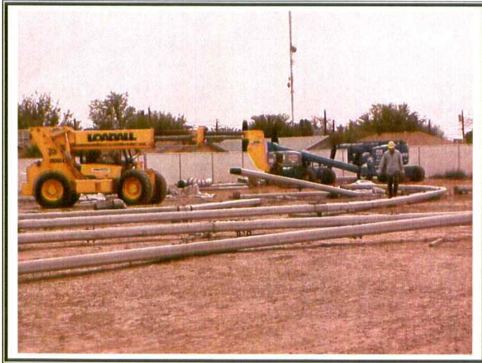
21. Structure crewmen disassemble framework and forklift stacks pieces.
