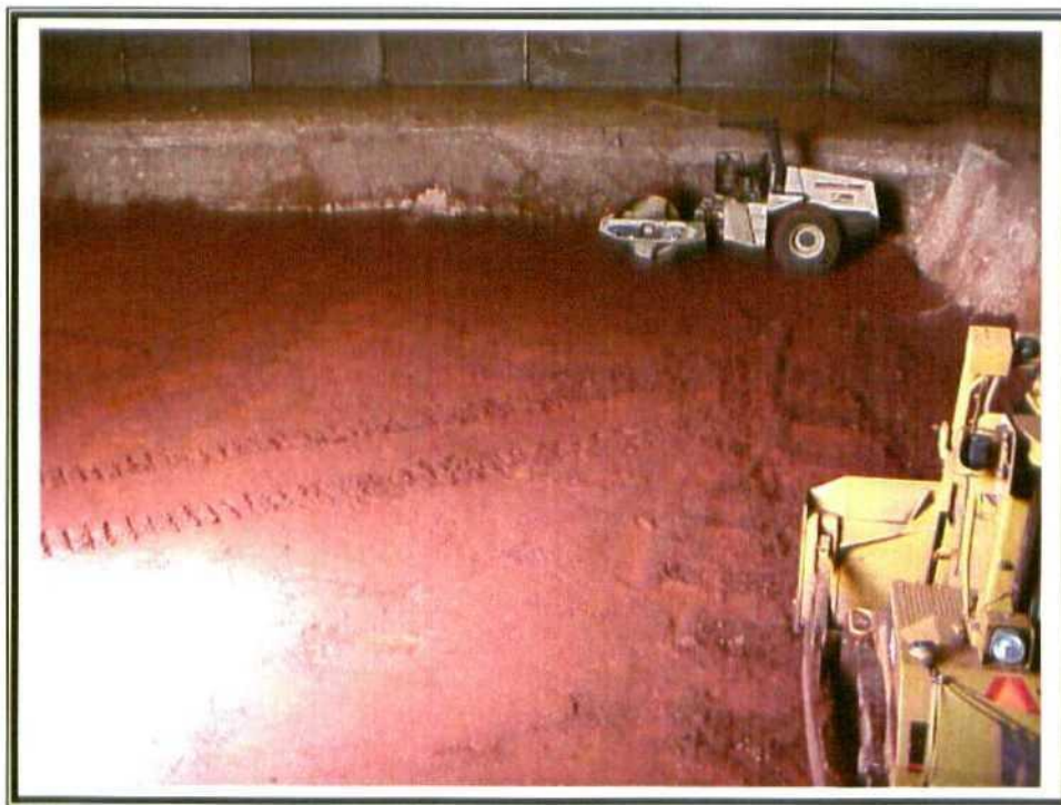
25. Phase II – Backfill clay liner.
