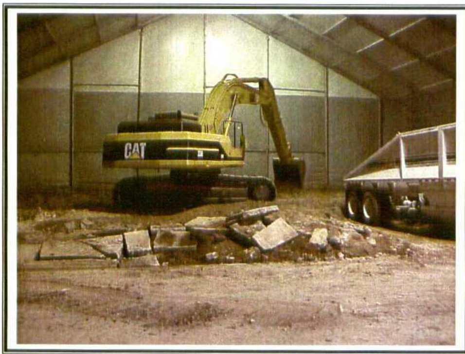
1. Phase I Excavation
