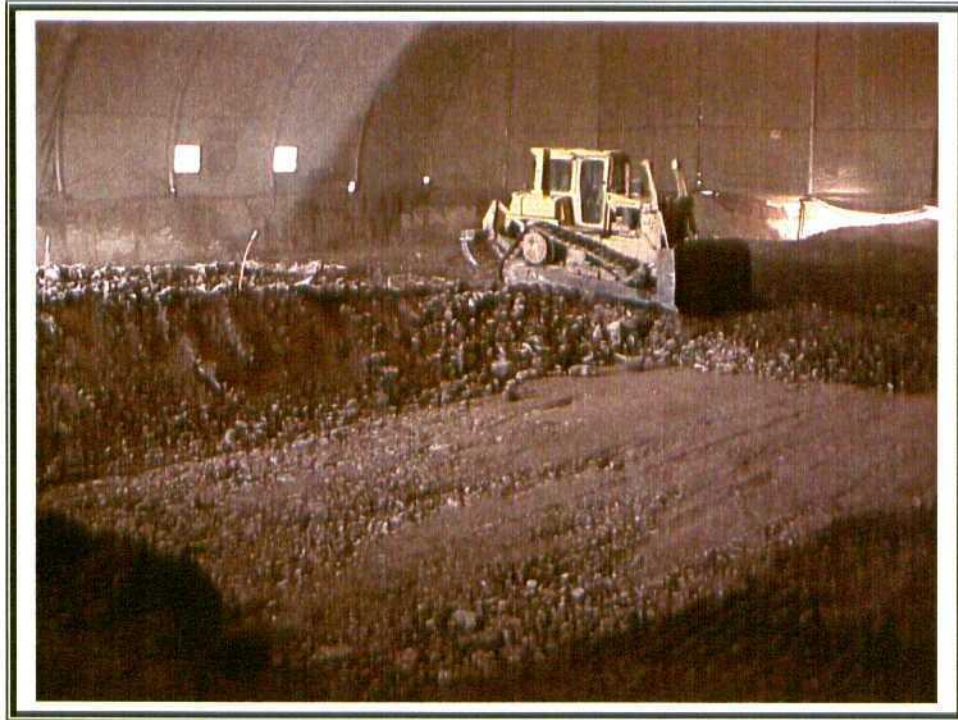
30. Phase III – Backfill. Dozer spreading caliche.
