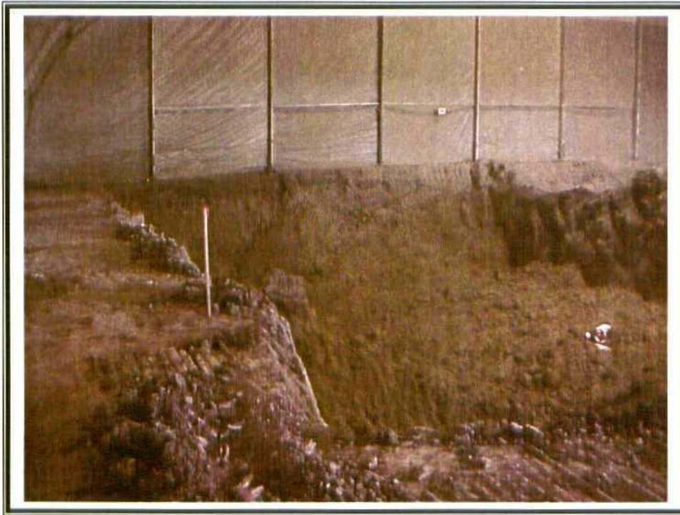
18. Phase III – Excavation.
