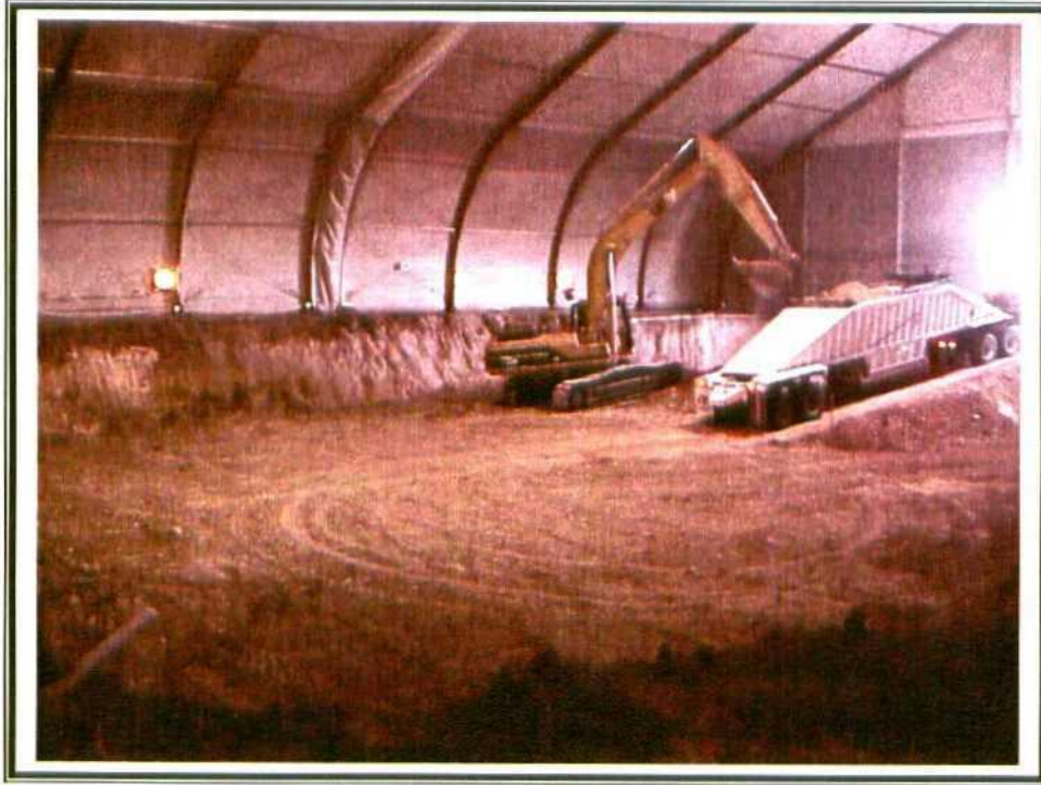
11. Phase I Excavation – Truck hauling soil out of structure
