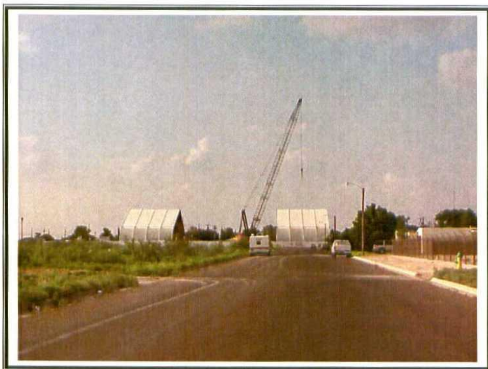
13. View of structure move from South Tasker.
