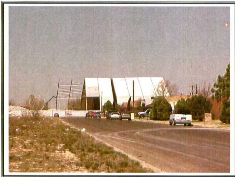
11. View of structure assembly from South Tasker.
