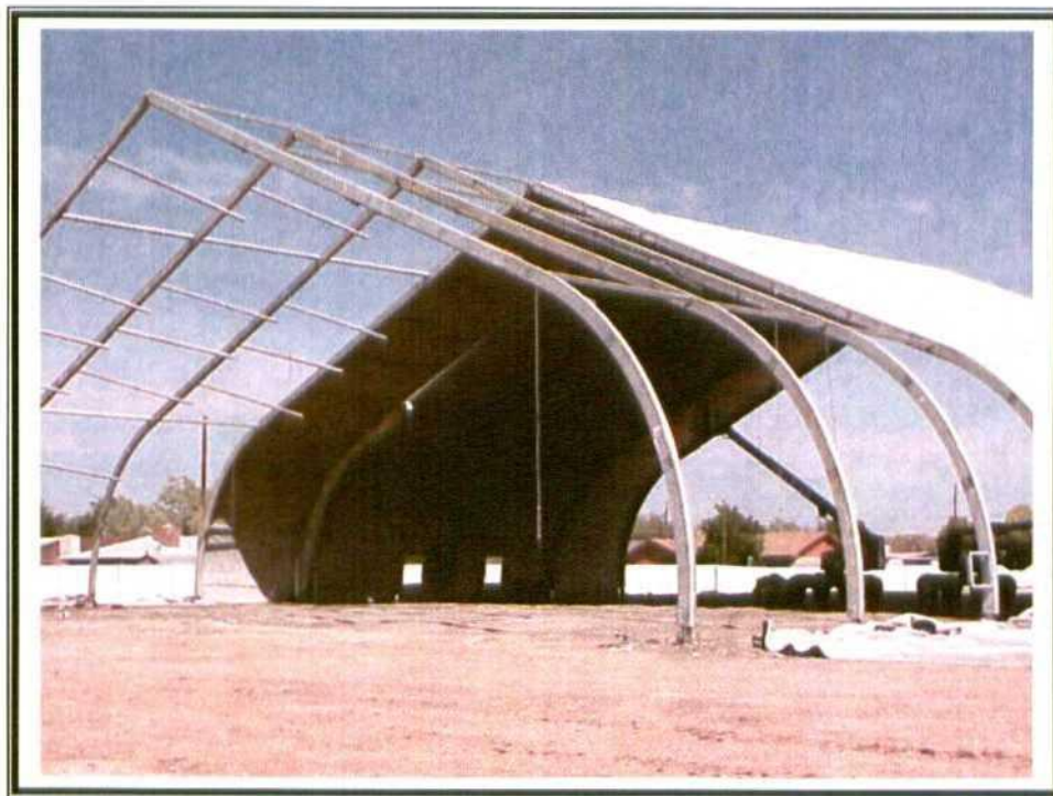
11. View of structure with fabric removed.
