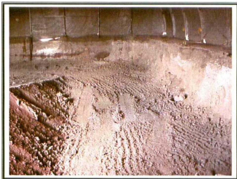
22. Phase III – Excavation – bottom hole.
