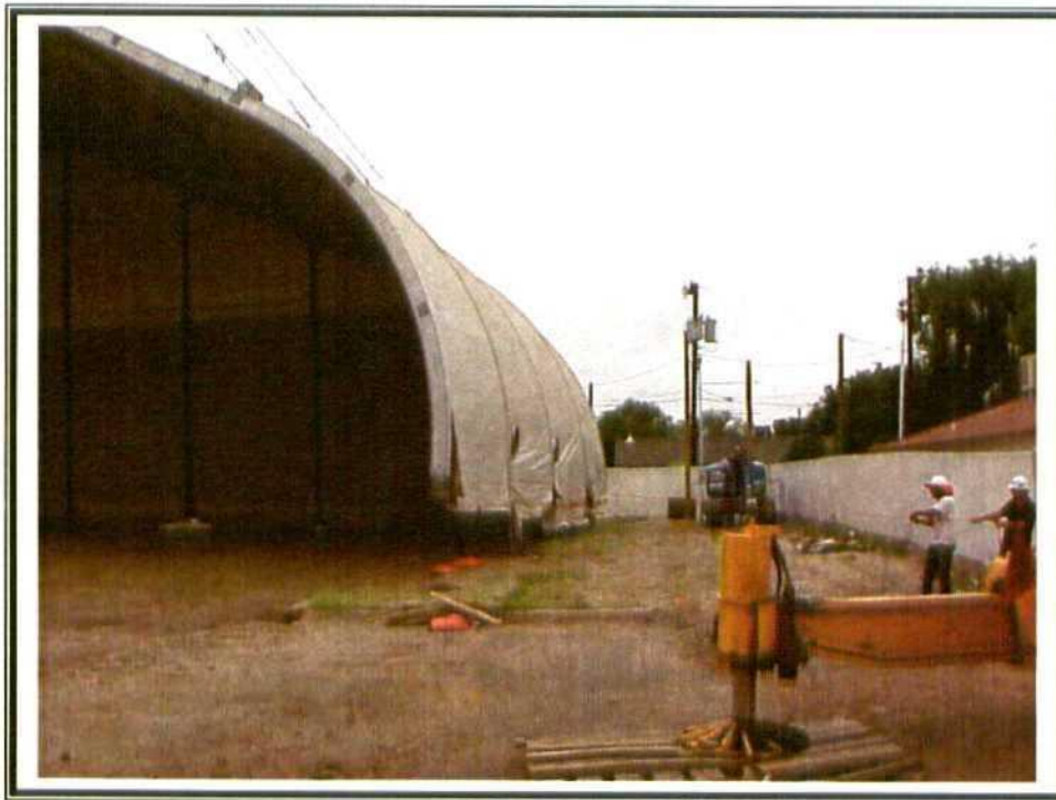
12. Lifting and moving back half of structure. Workers hold a rope tied to the corner of the structure to keep it steady.
