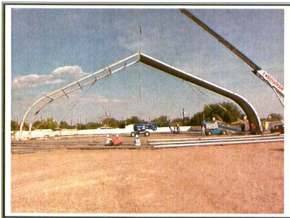
18. Last two pieces of framework standing. Final piece was tied down to stabilize it.
