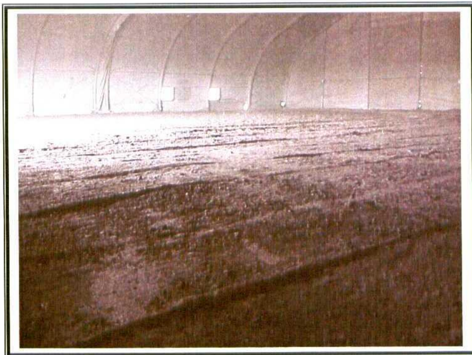
37. Phase III – Backfill completed.
