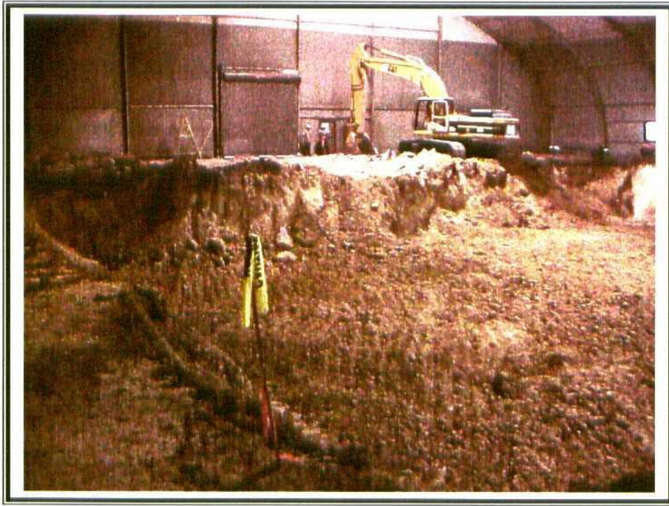
7. Phase I Excavation
