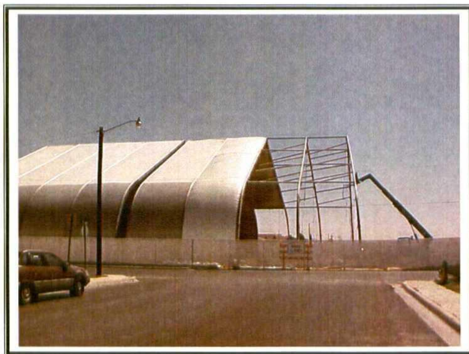
9. View of structure assembly from North Tasker Street.
