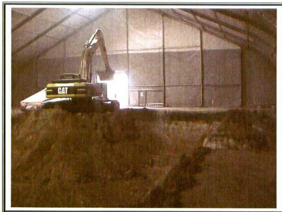
6. Phase I Excavation
