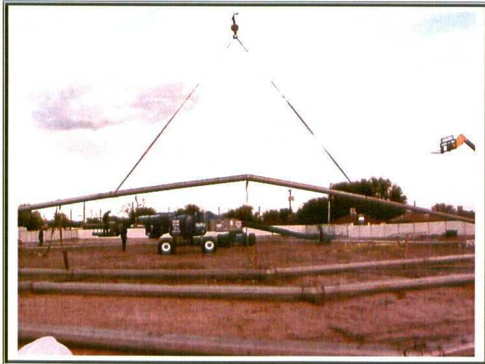
19. Final piece of structure framework is lowered.
