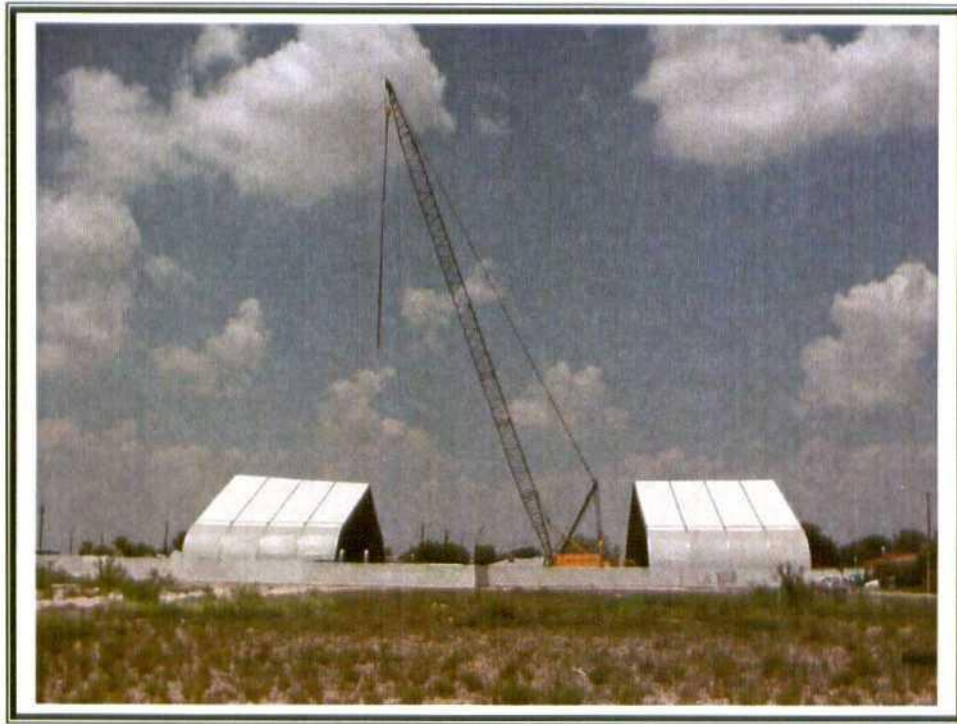
9. View of structure move from nearby field.
