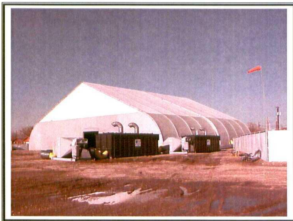
15. Structure and carbon filtration system assembly complete.
