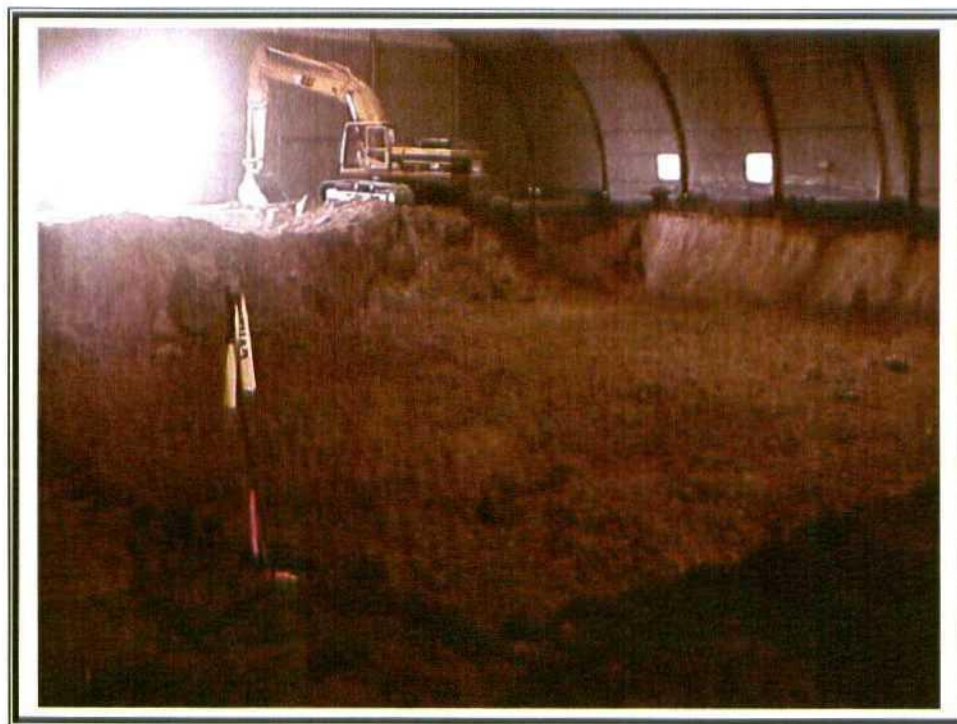
4. Phase I Excavation
