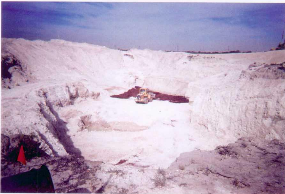
Installation of lower liner.
