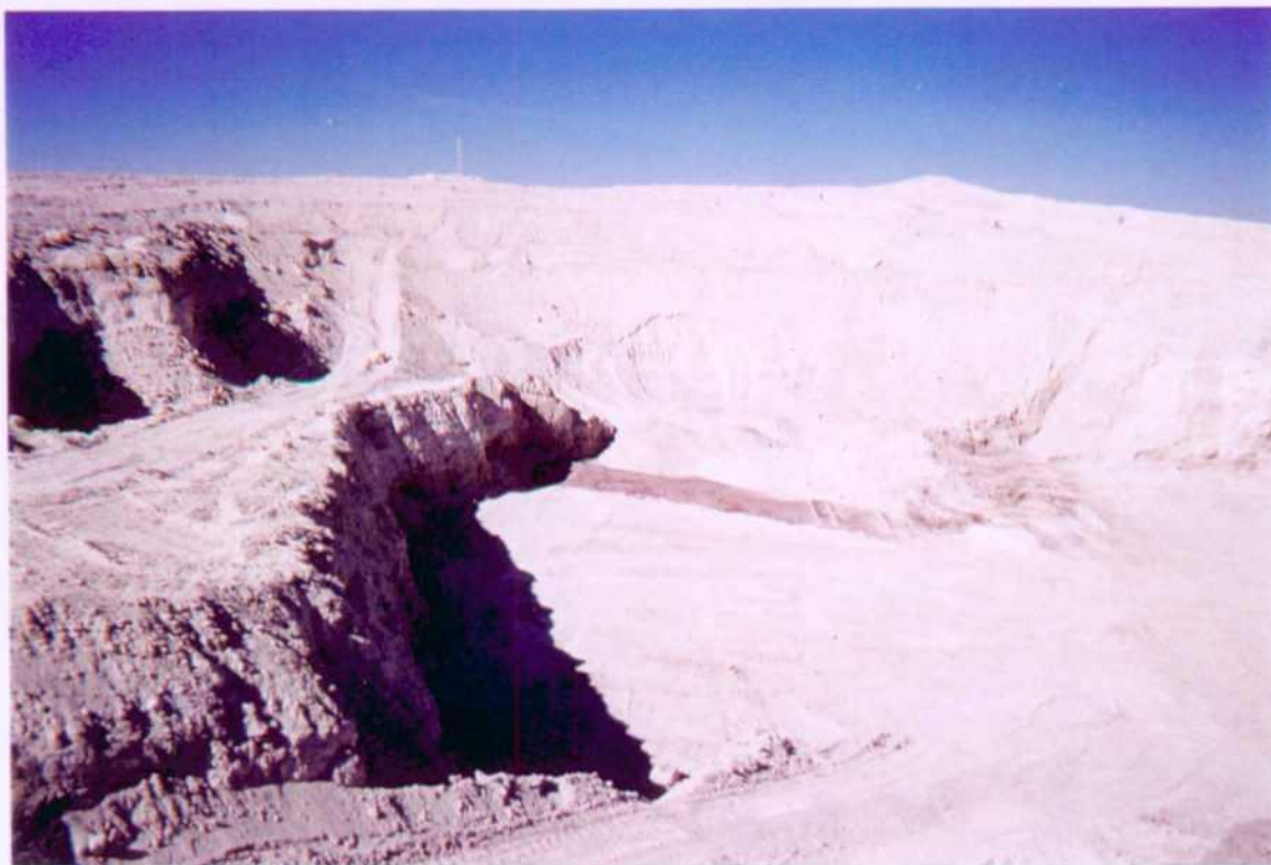
Backfilling over lower liner.
