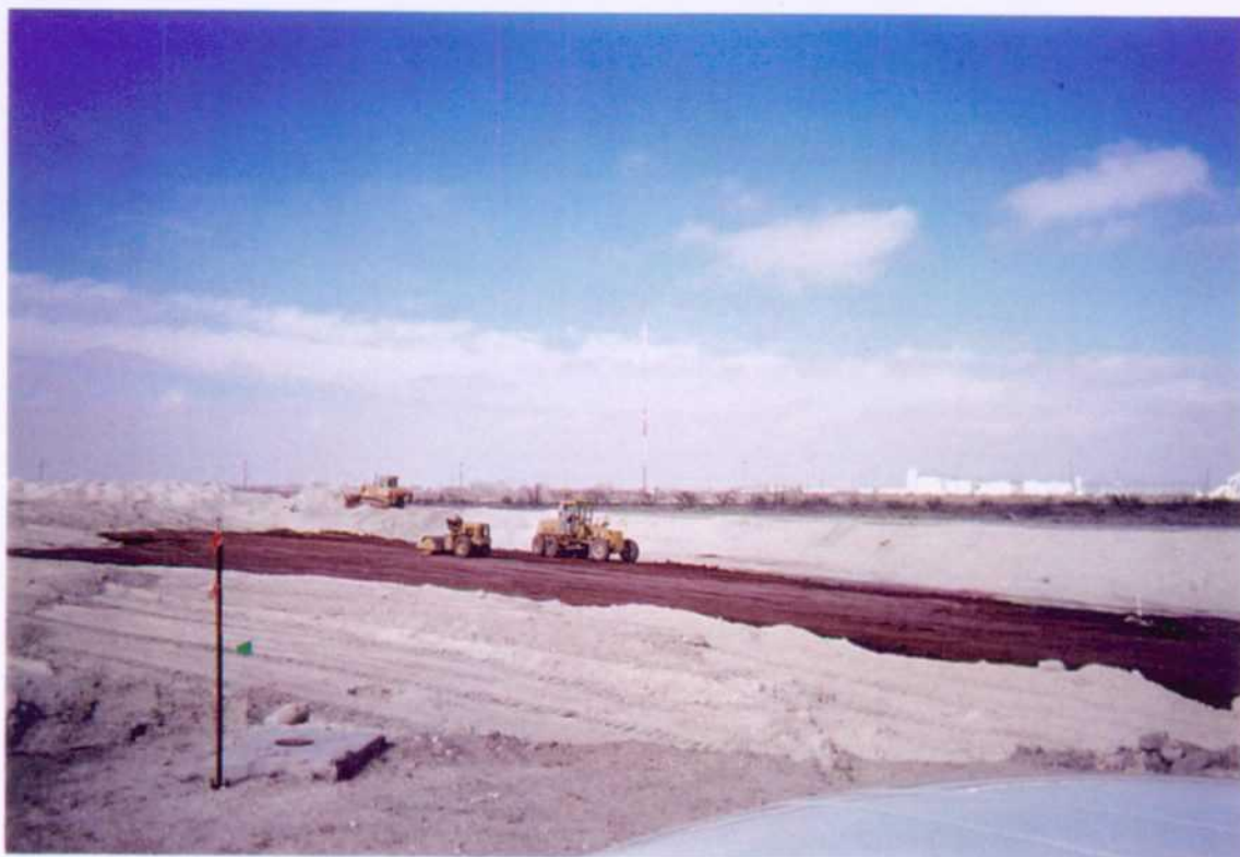
Installation of upper liner.
