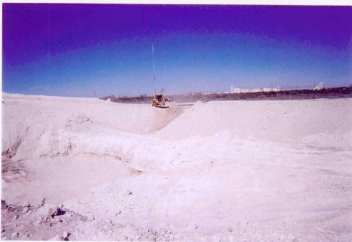
Backfilling over lower liner.
