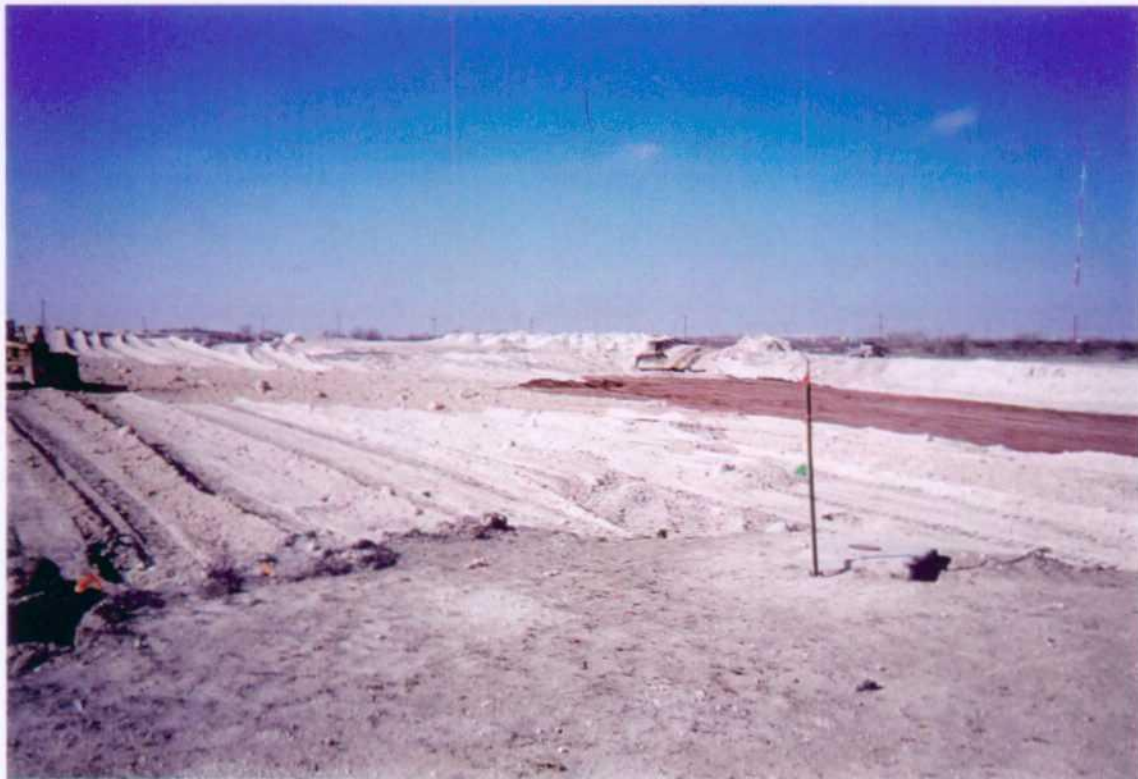
Backfilling over upper liner.
