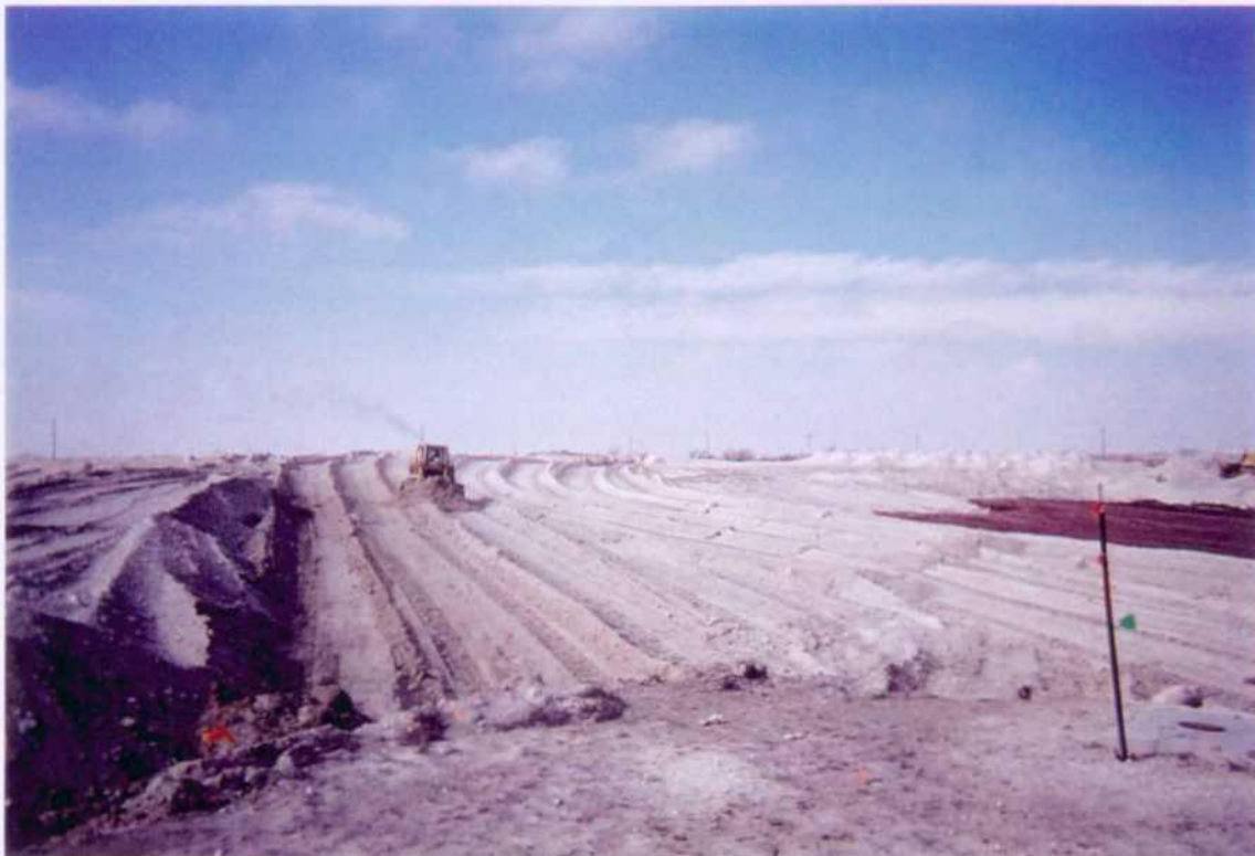
Backfilling over upper liner.
