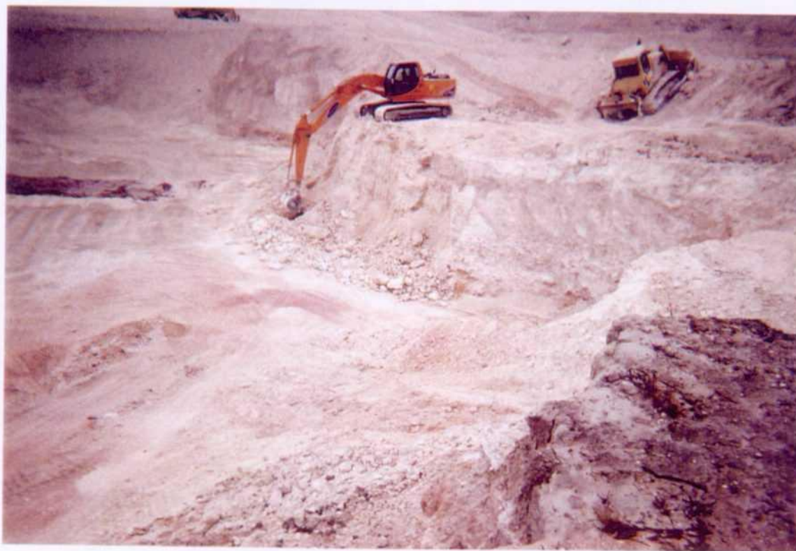
Excavation of sidewalls.
