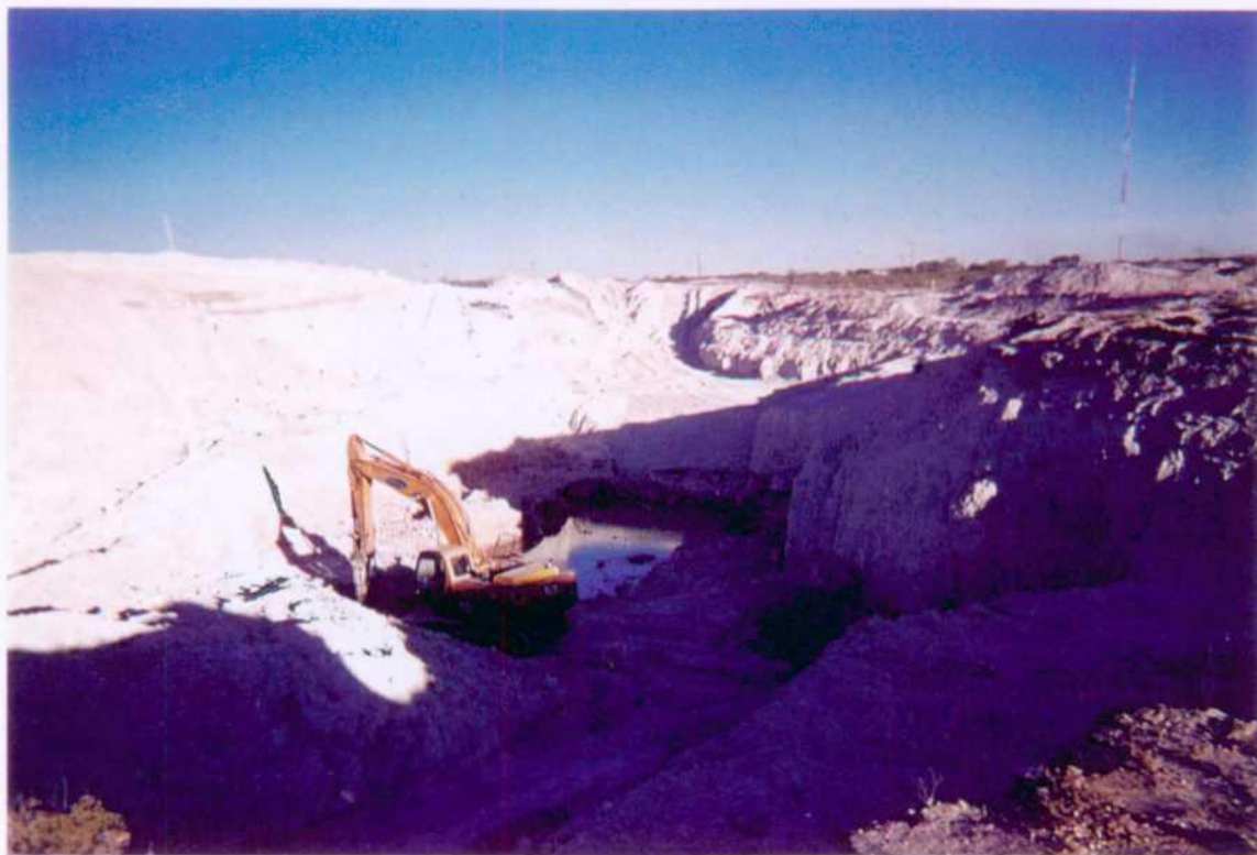
Excavation to groundwater in area where PSH was detected.
