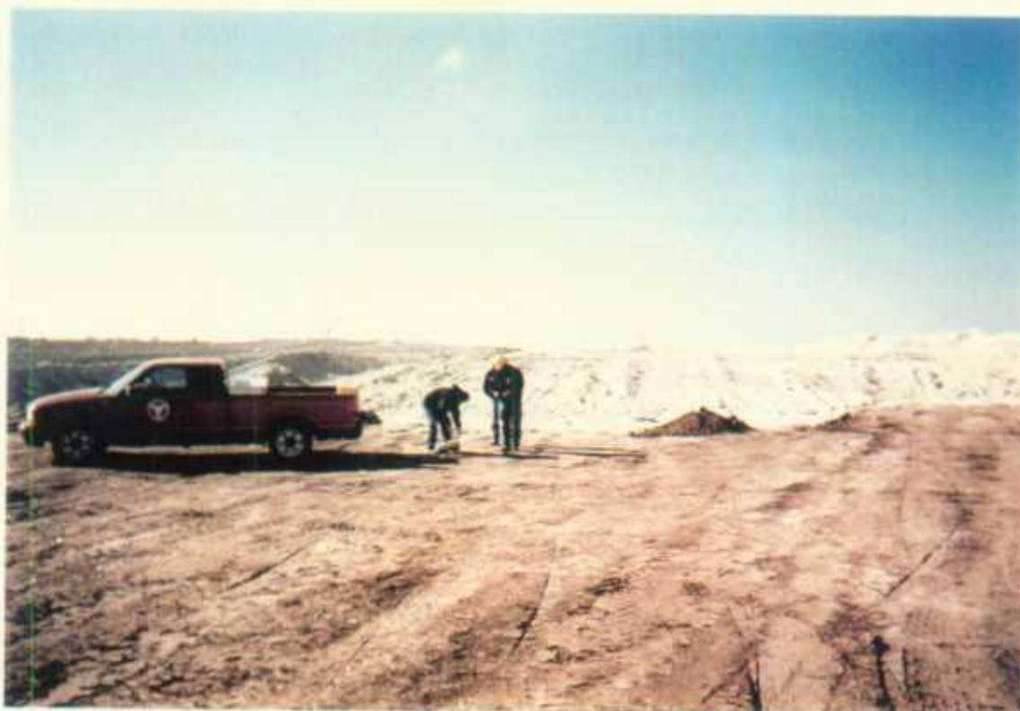
Proctor testing of upper liner.
