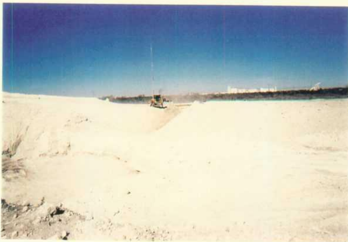
Backfilling over lower liner.
