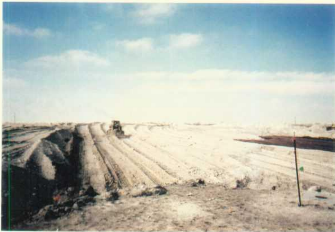
Backfilling over upper liner.
