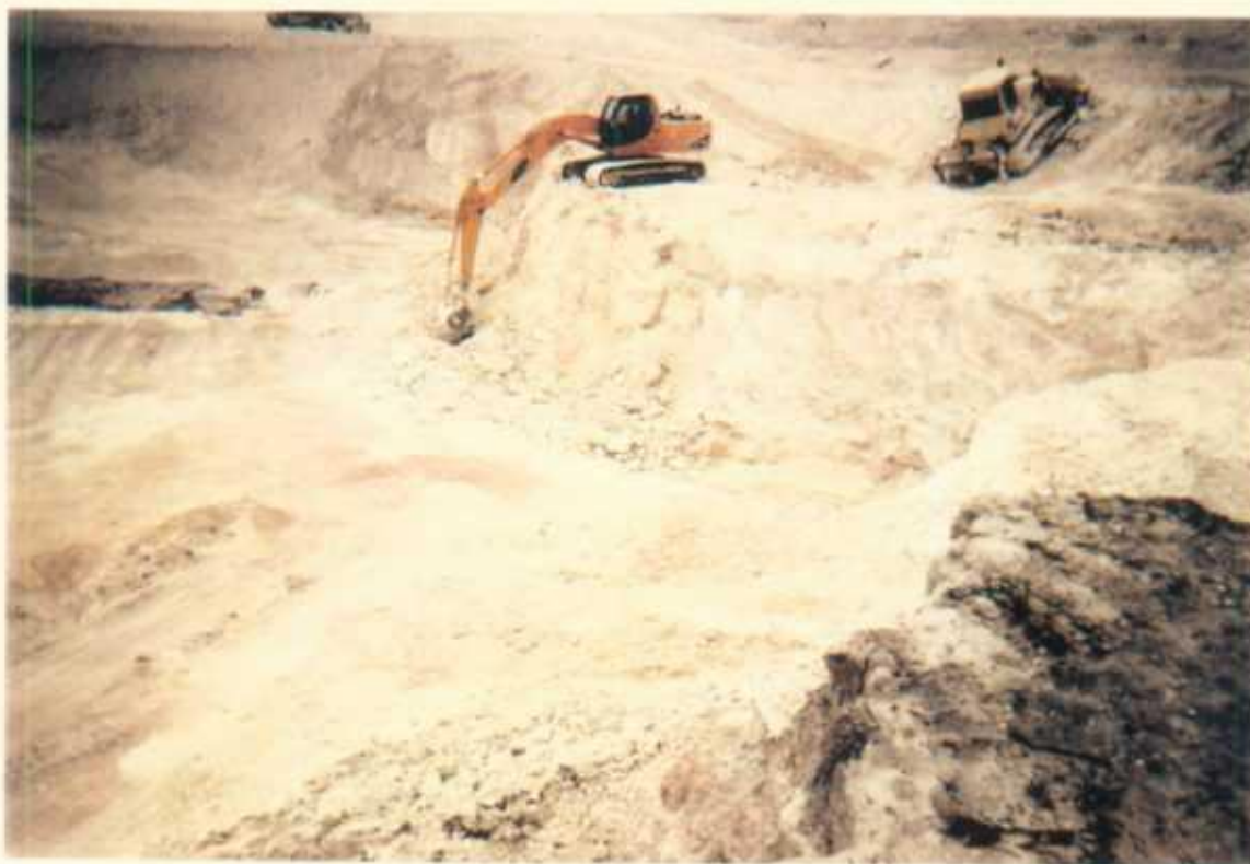
Excavation of sidewalls.
