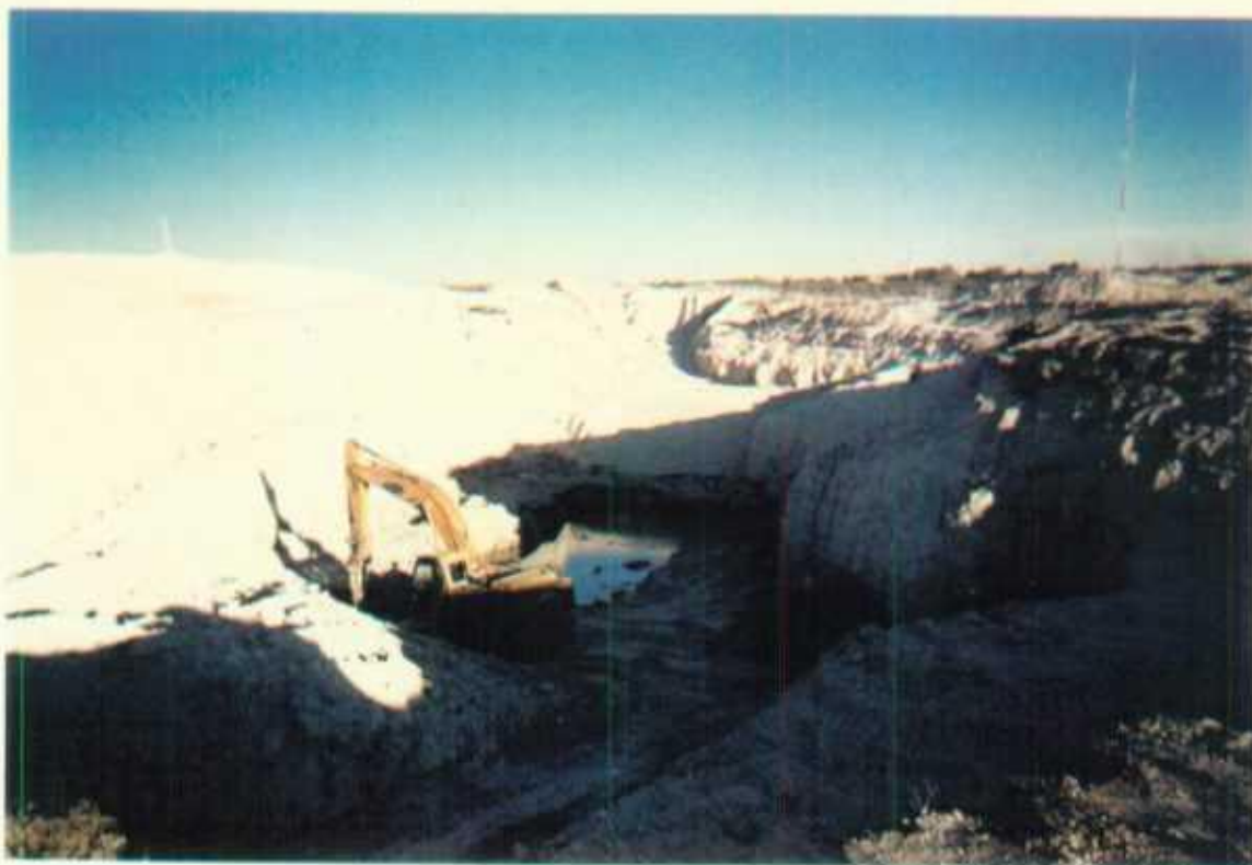
Excavation to groundwater in area where PSH was detected.
