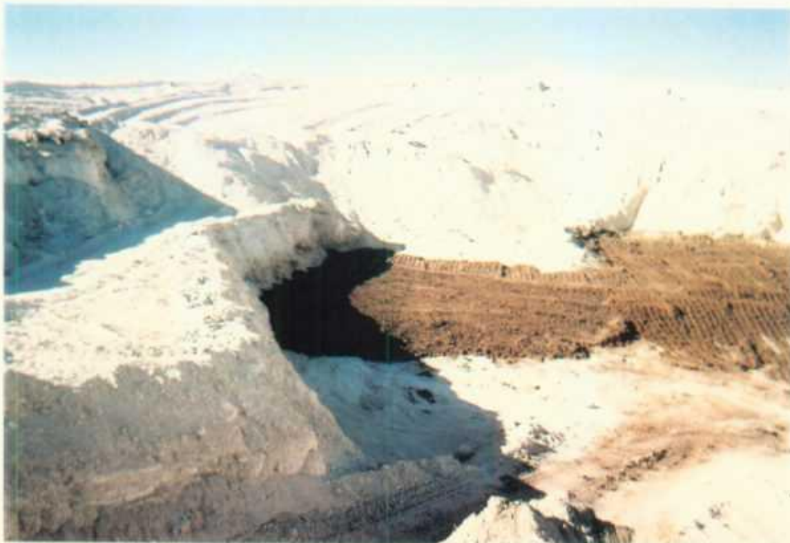
Installation of lower liner.
