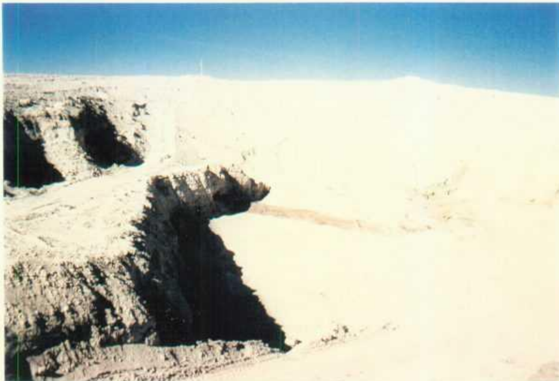
Backfilling over lower liner.
