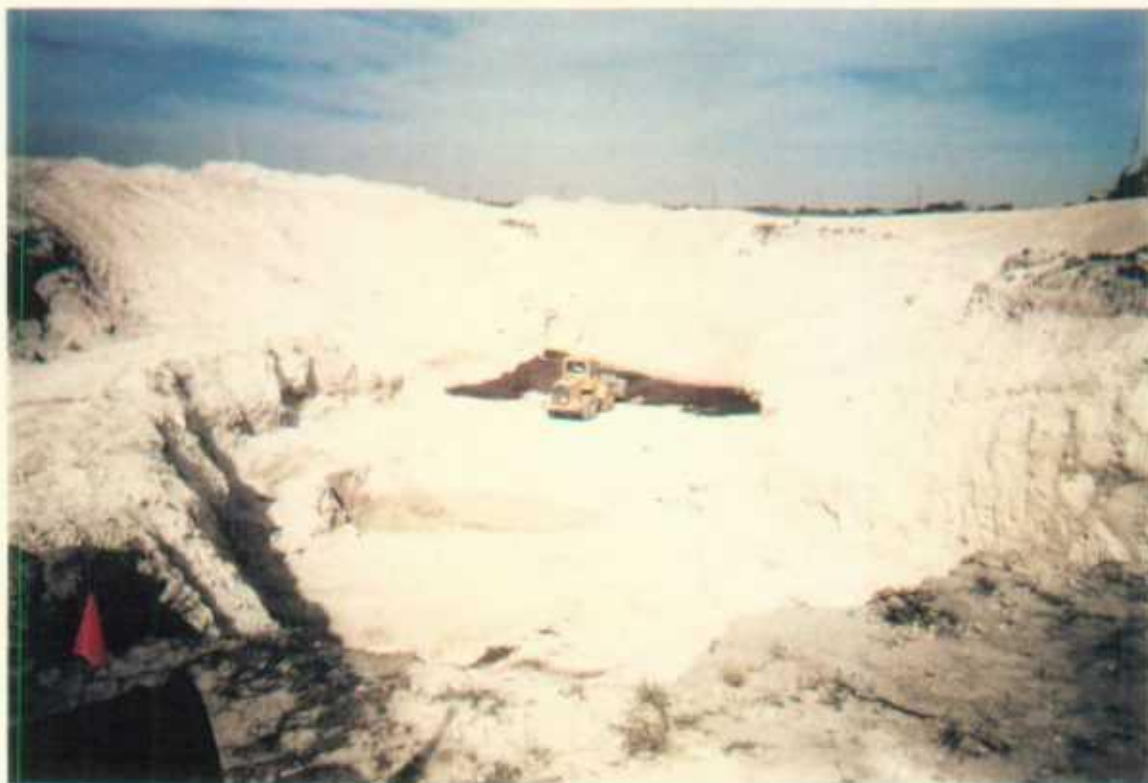
Installation of lower liner.
