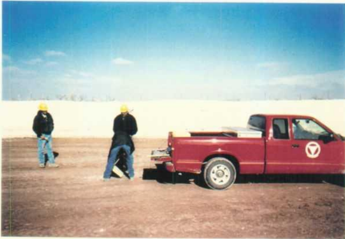
Proctor testing of upper liner.
