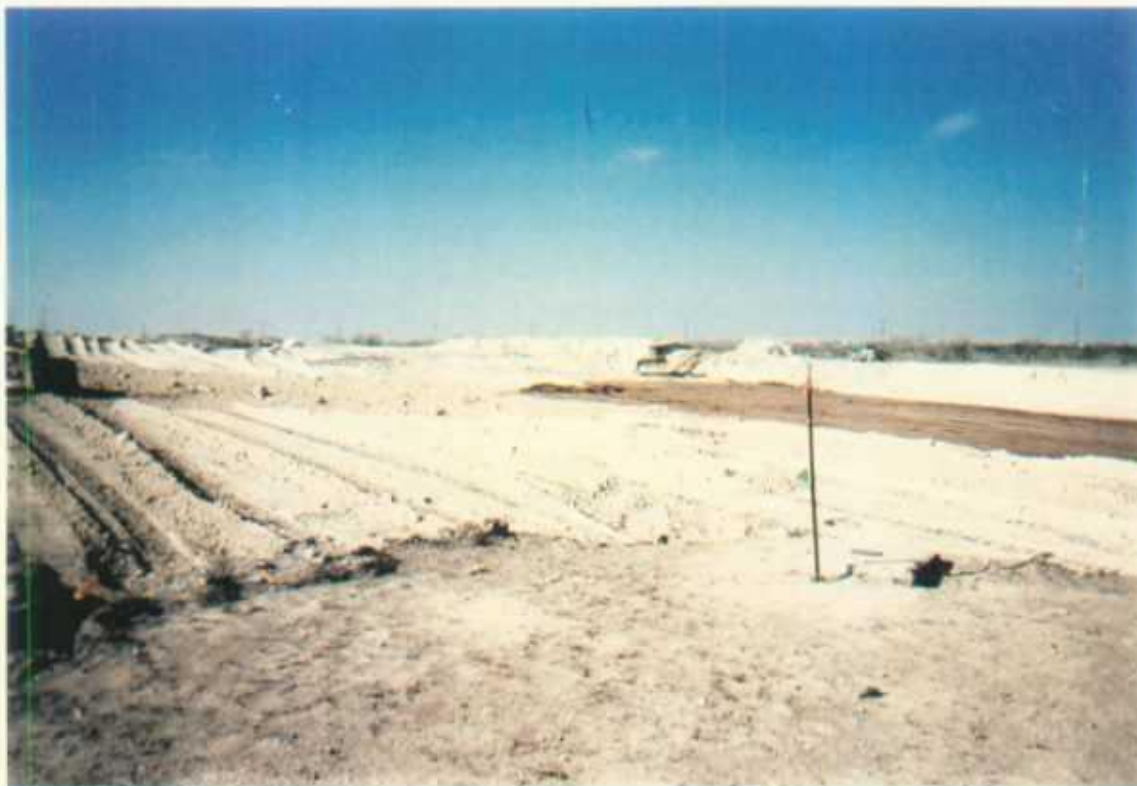
Backfilling over upper liner.
