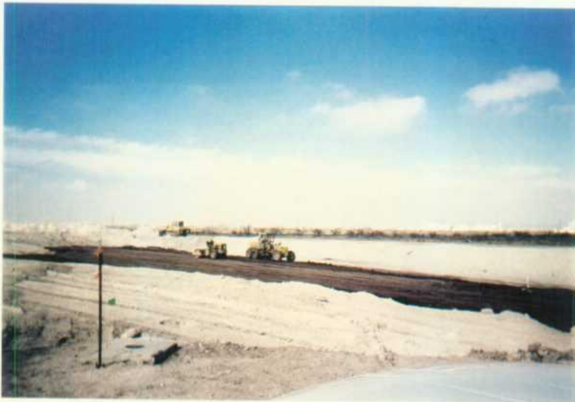
Installation of upper liner.
