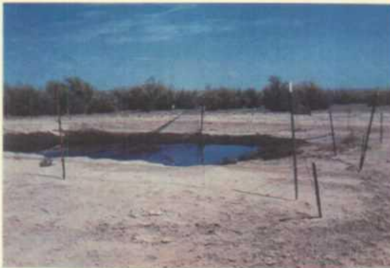
Photo 1: Williams Tank Battery unlined disposal pit prior to Yates' acquisition of the site.
