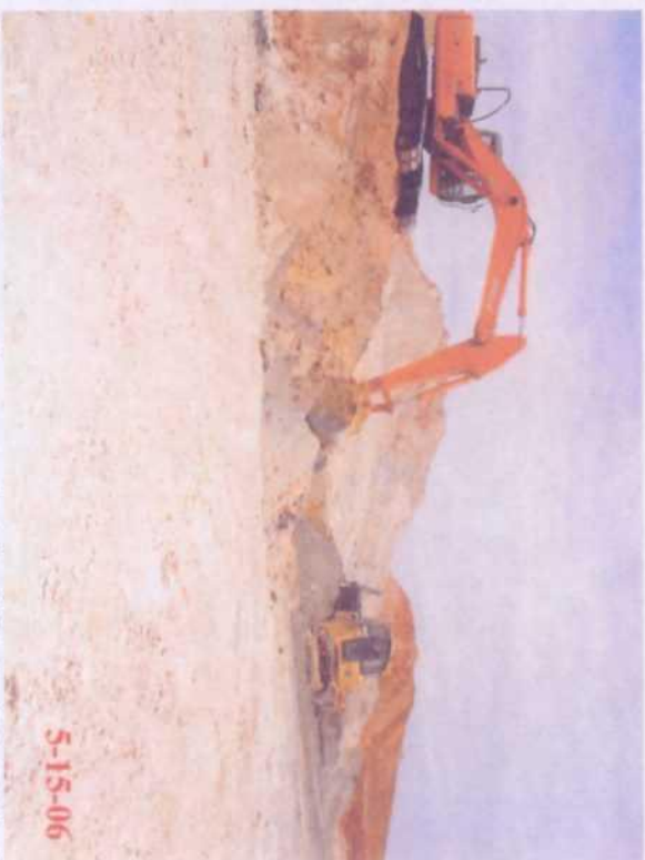
Dozer and Trackhoe excavating contaminated soil North of Test Point G
