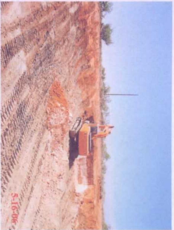
Trackhoe excavating contaminated soil on South wall of Test Point E
