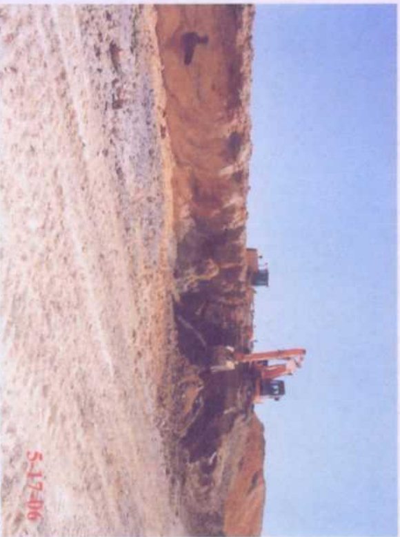
Trackhoe excavating contaminated soil on North wall of Test Point G
