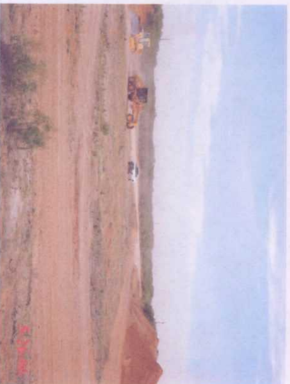
Building new caliche road to reach area of backfill material
