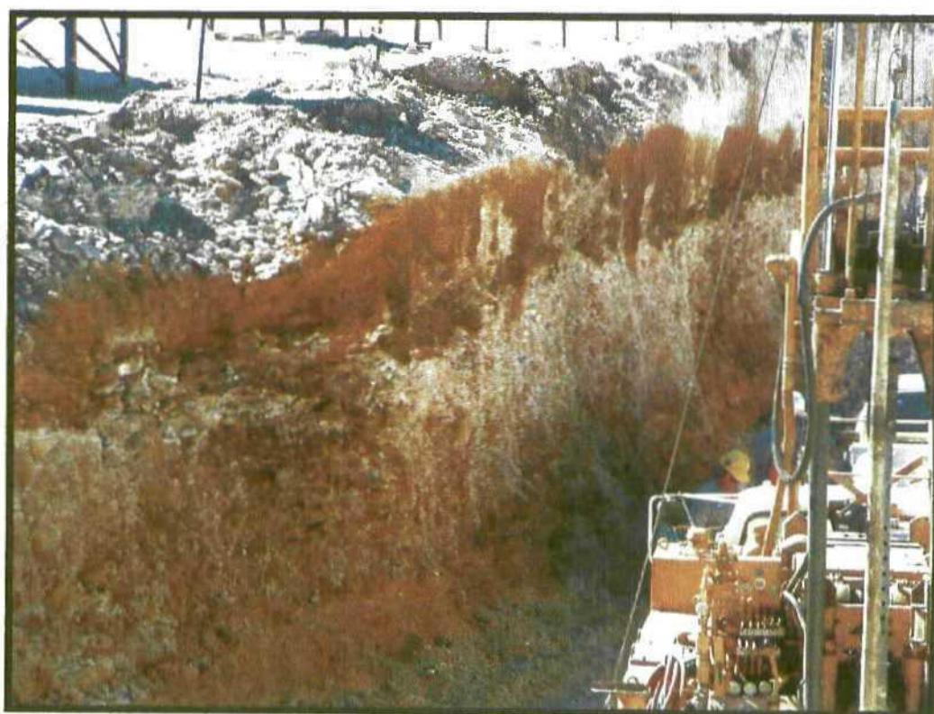
Installation of temporary recovery wells at the Monument pipeline release site, November 13, 2002 The pipeline was located adjacent to the base of the hydrocarbon stained soil on the left wall.
