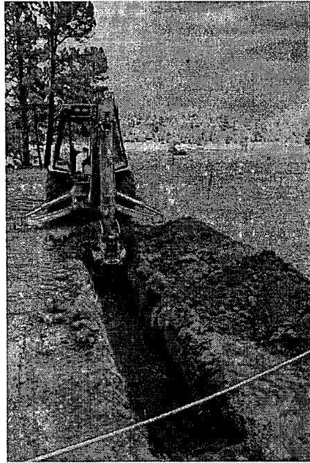
Exploratory trenching at the Gasbuggy SGZ
