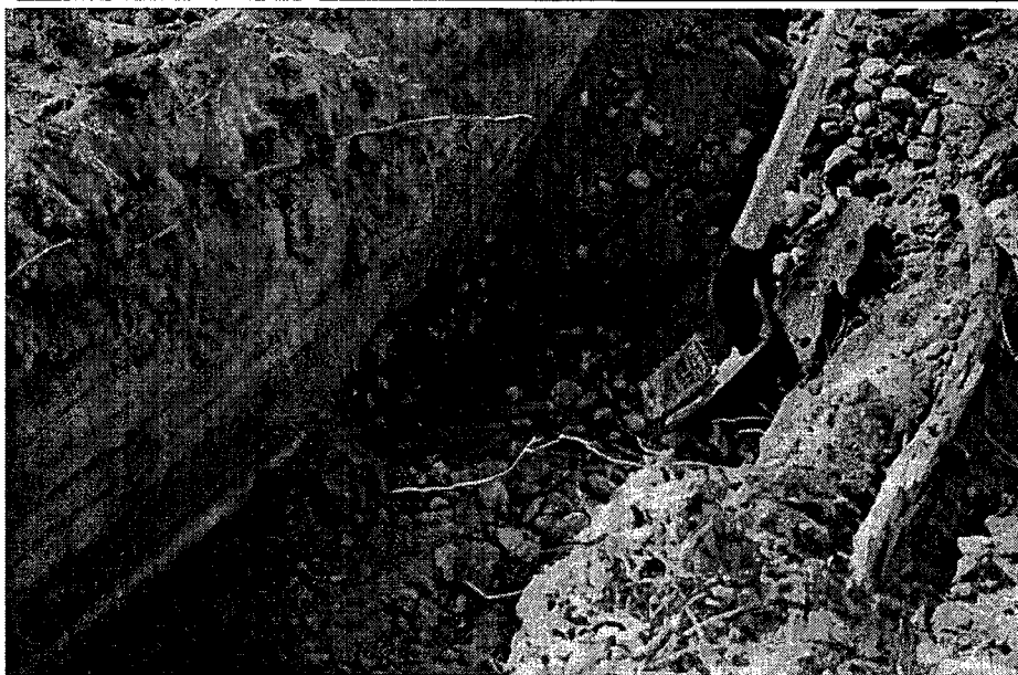
Leach line and leach rock at the Gasbuggy CP
