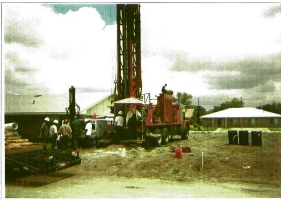
TEG Installation of TSV-M & Installation of TMW-1 by Eades Drilling
