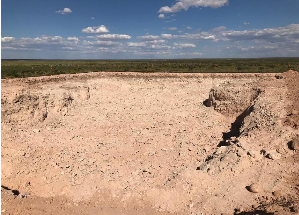
Photograph 1: View east of excavation.
