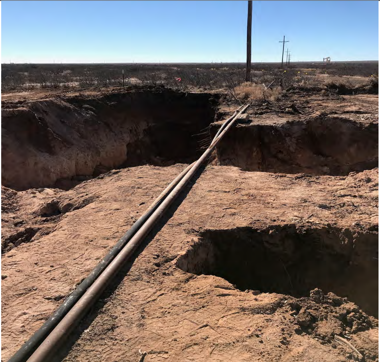
View of excavation.
