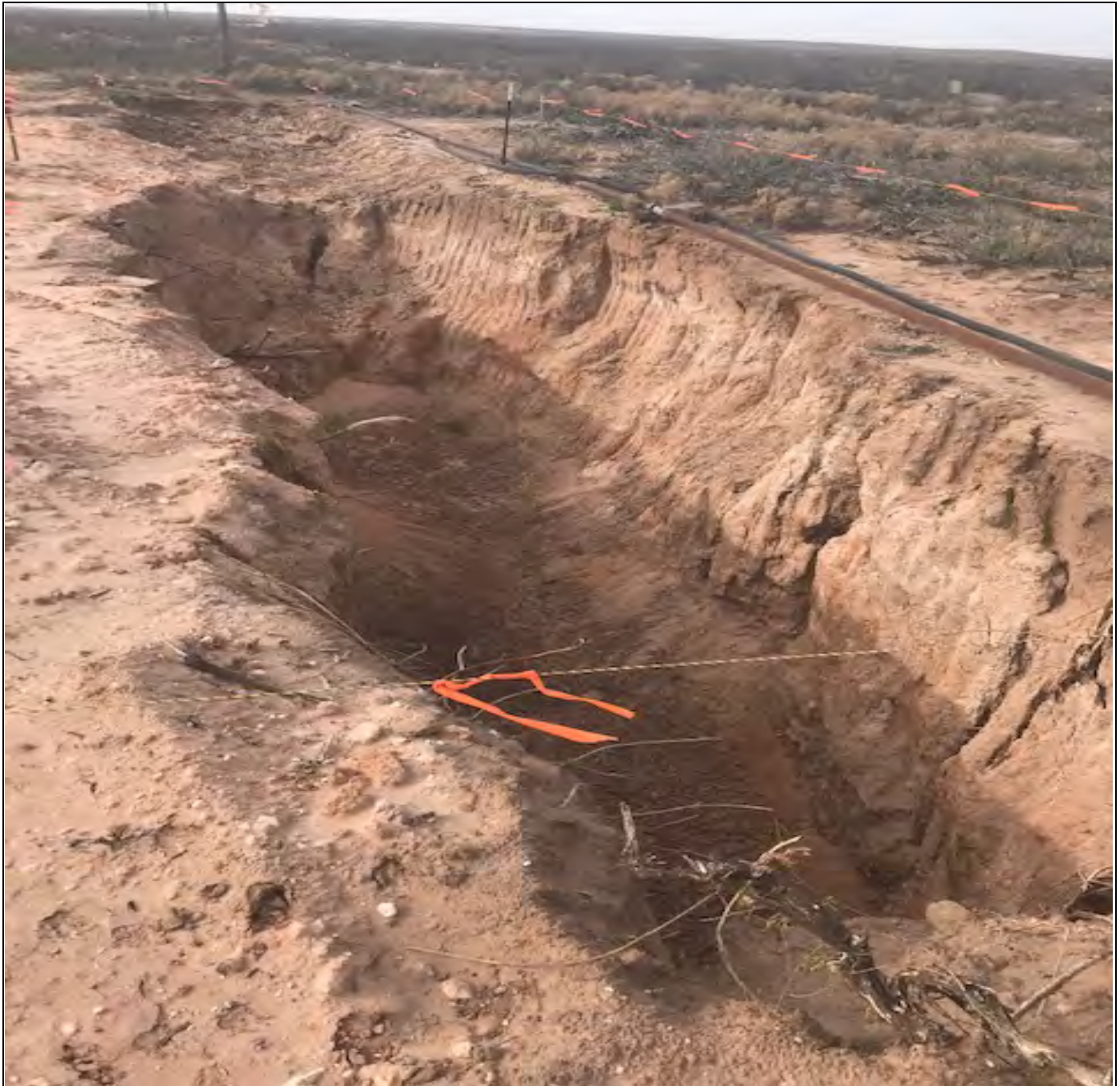
View of excavation.
