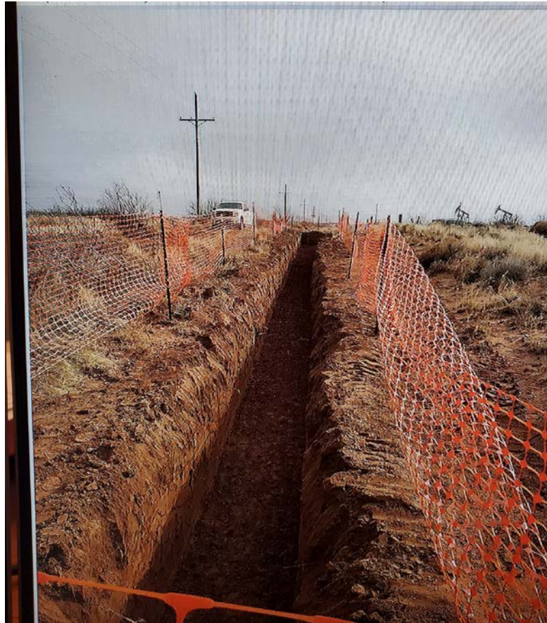
View of Excavation
