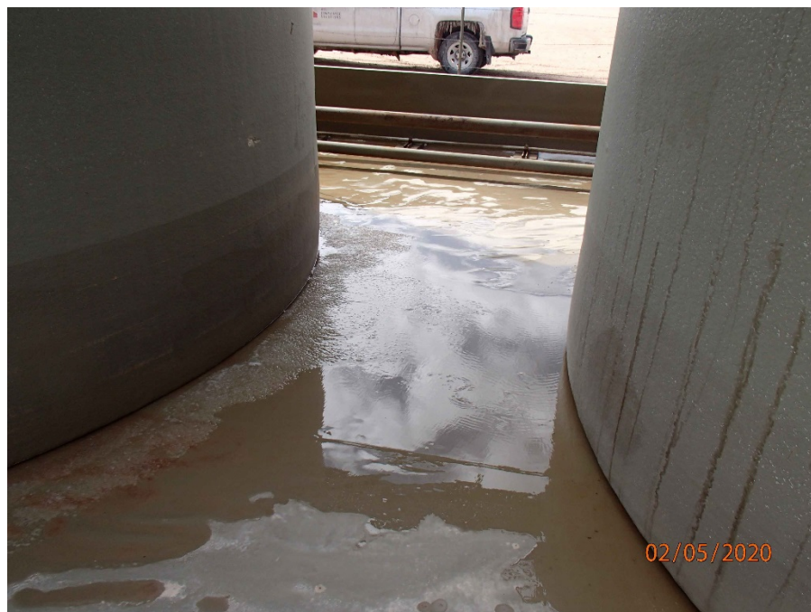
View of standing water between the tanks in the secondary containment.
