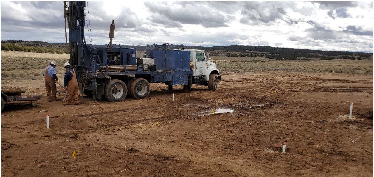
Photo 2: SB-6 boring installation. SB-1 through SB-5 at right. Photo taken 3/11/2020.
