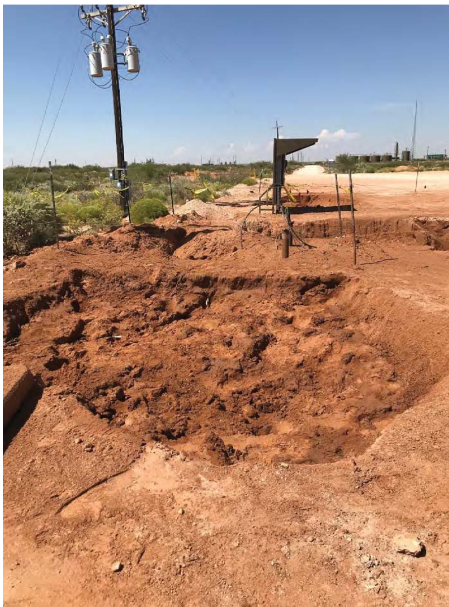
View of the eastern excavation facing west.
