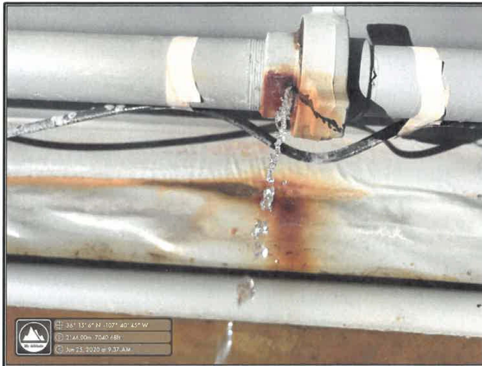
Photo 1: View of Leaking Line
