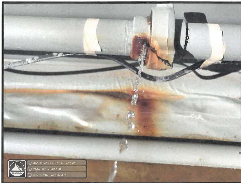
Photo 1: View of Leaking Line
