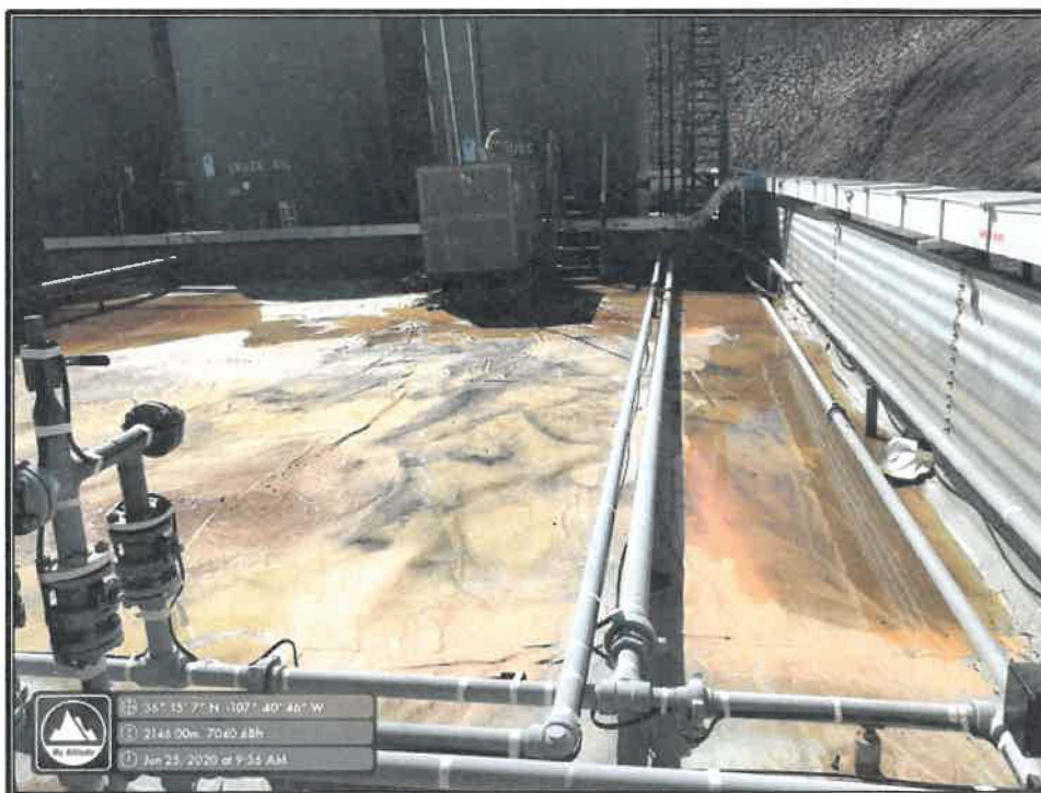
Photo 2: View of Water on Liner
