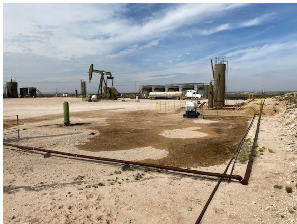
Photograph 1: View of staining on pad from release facing west.
