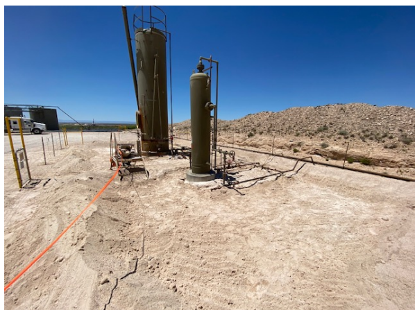
Photograph 5: View of excavation around equipment facing northwest.
