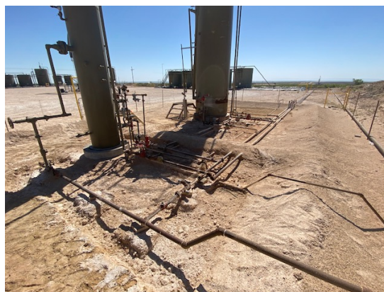
Photograph 4: View of hydrovac excavation around equipment facing southwest.
