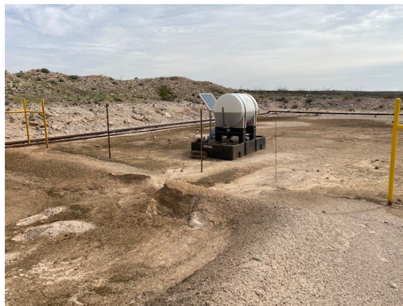
Photograph 2: View of breached earthen berm and staining in northeast corner of well pad.
