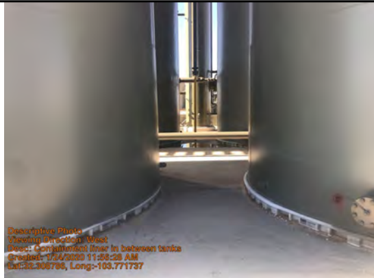
Containment liner in between tanks
