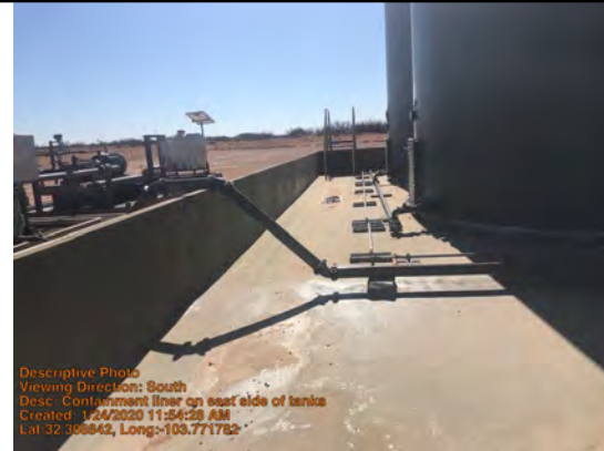
Containment liner on east side of tanks
