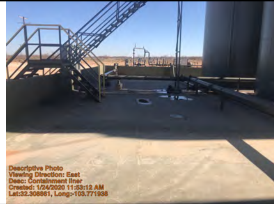
Containment liner on north side of tanks
