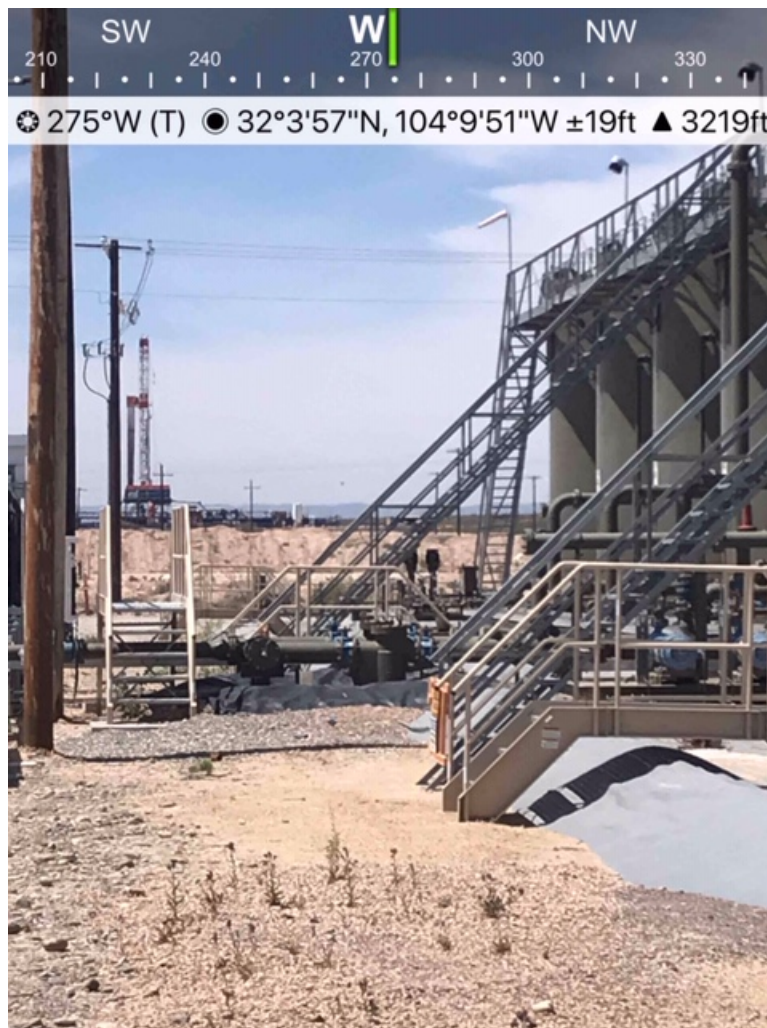
Proposed excavation area viewing west
