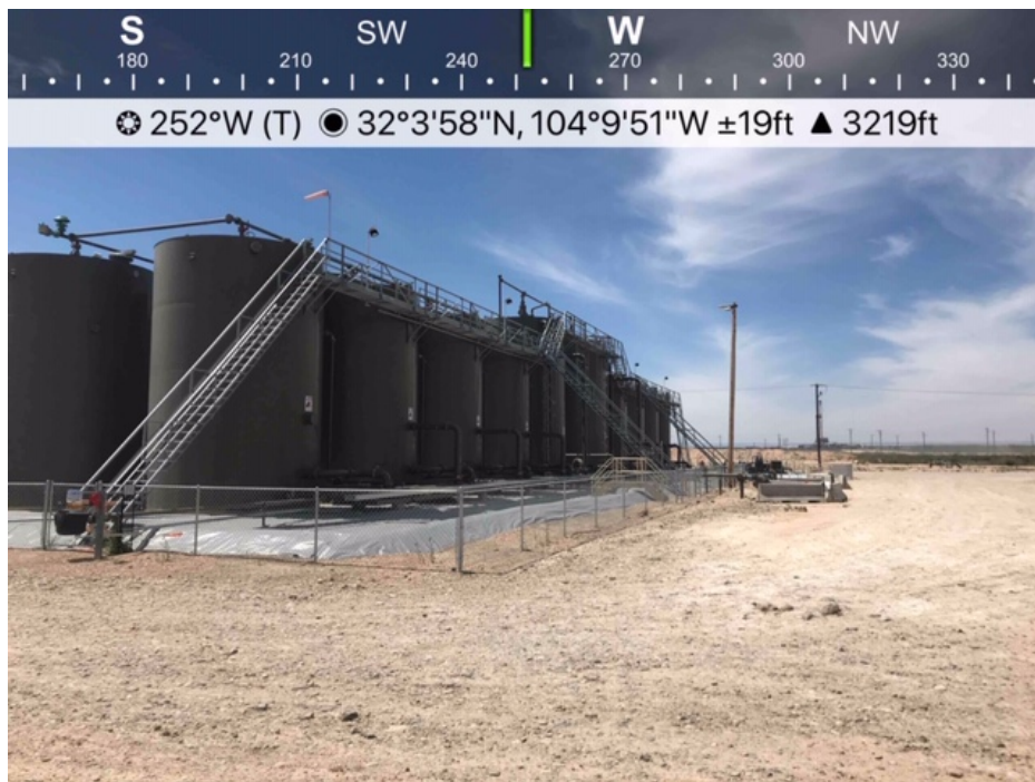
Spill within lined containment viewing southwest/west
