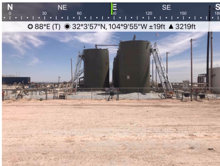
Spill within lined containment viewing east
