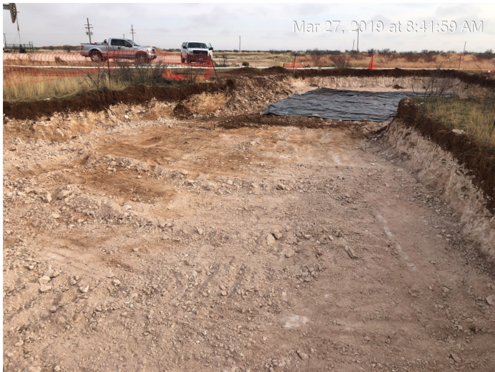
View North – View of excavation and liner installation at Bottom Hole 5 and 6
