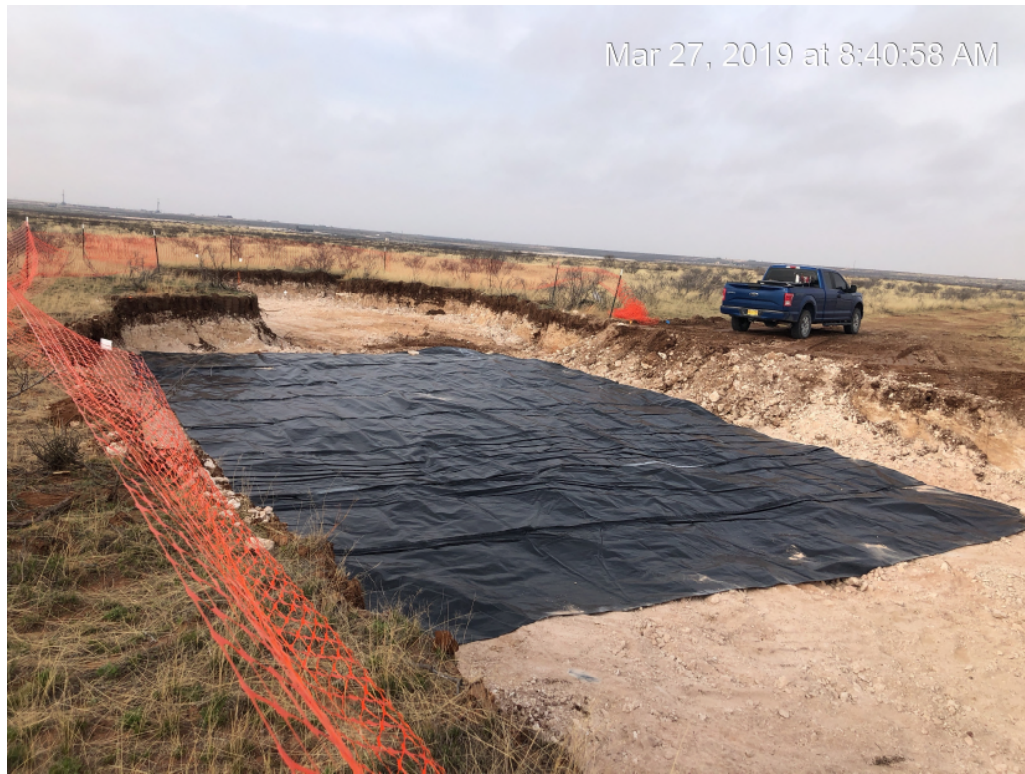
View Southwest – View of excavation and liner installation at Bottom Hole 5 and 6
