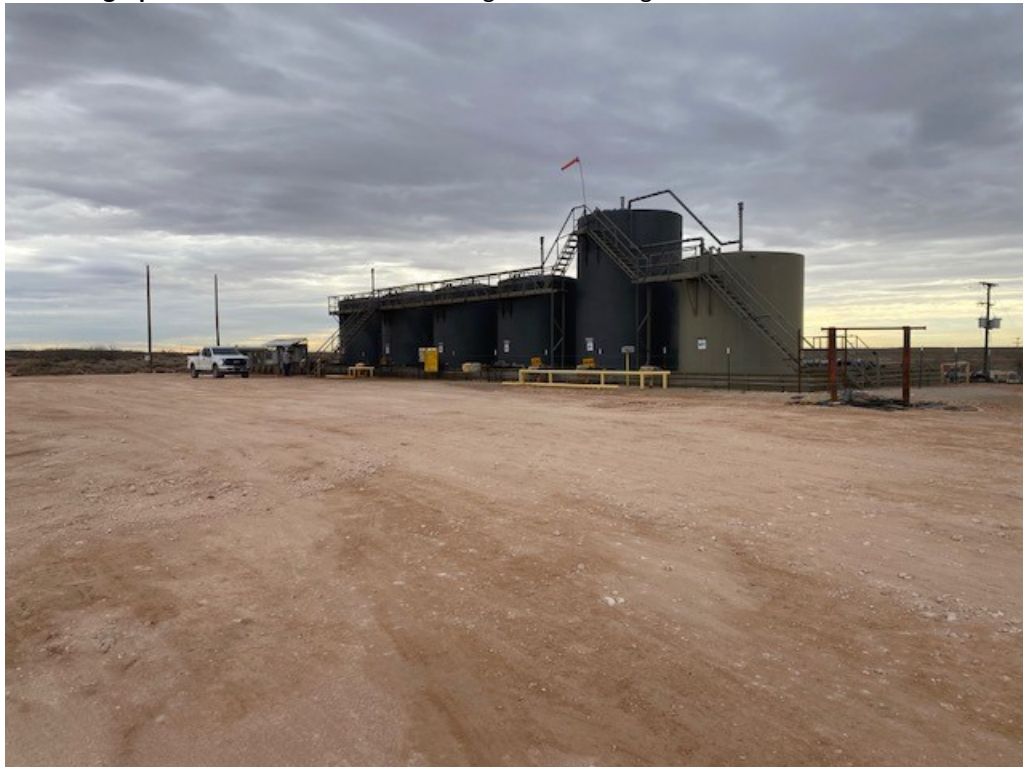
Photograph 8: Northeastern view of Site after final backfilling operations.
