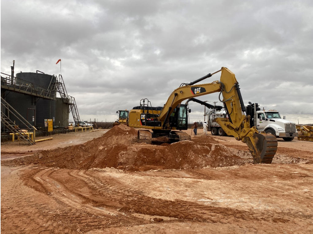
Photograph 3: Western view of the Site during excavation activities.
