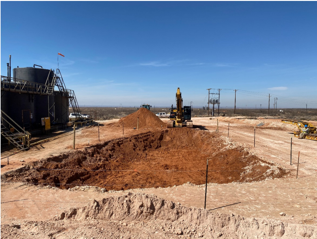
Photograph 4: Western view of the Site during final excavation activities.
