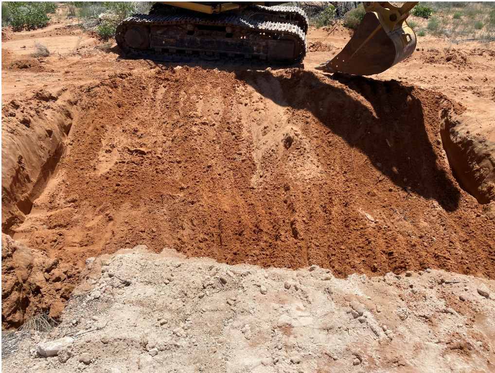
Photograph 6: Southern view of Site during final excavation activities in pipeline ROW.
