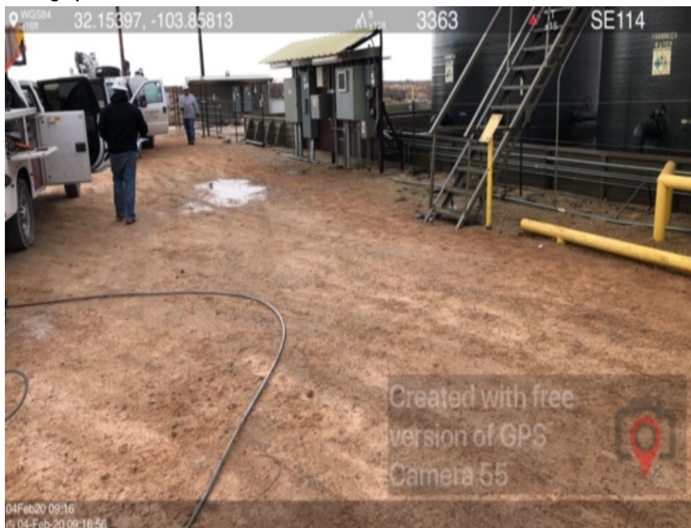
Photograph 2: Southeastern view of release extent.
