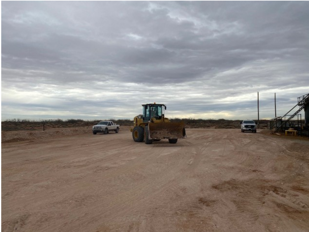
Photograph 7: Eastern view of Site during the backfilling activities.
