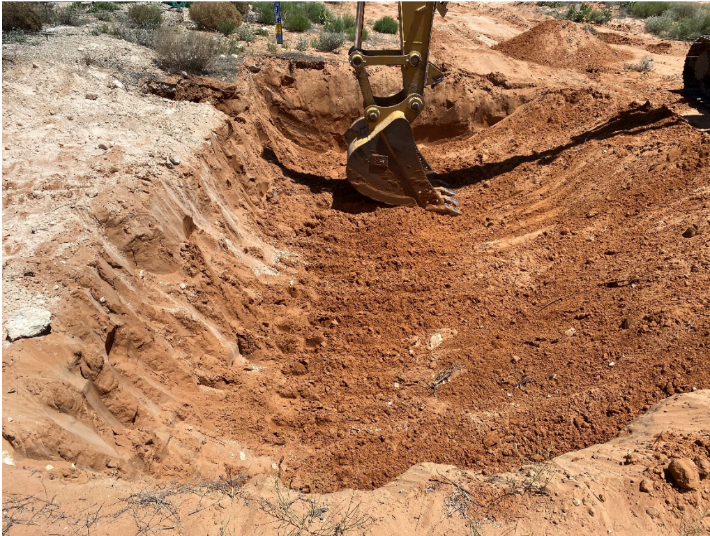
Photograph 5: Eastern view of Site during excavation activities in pipeline ROW.
