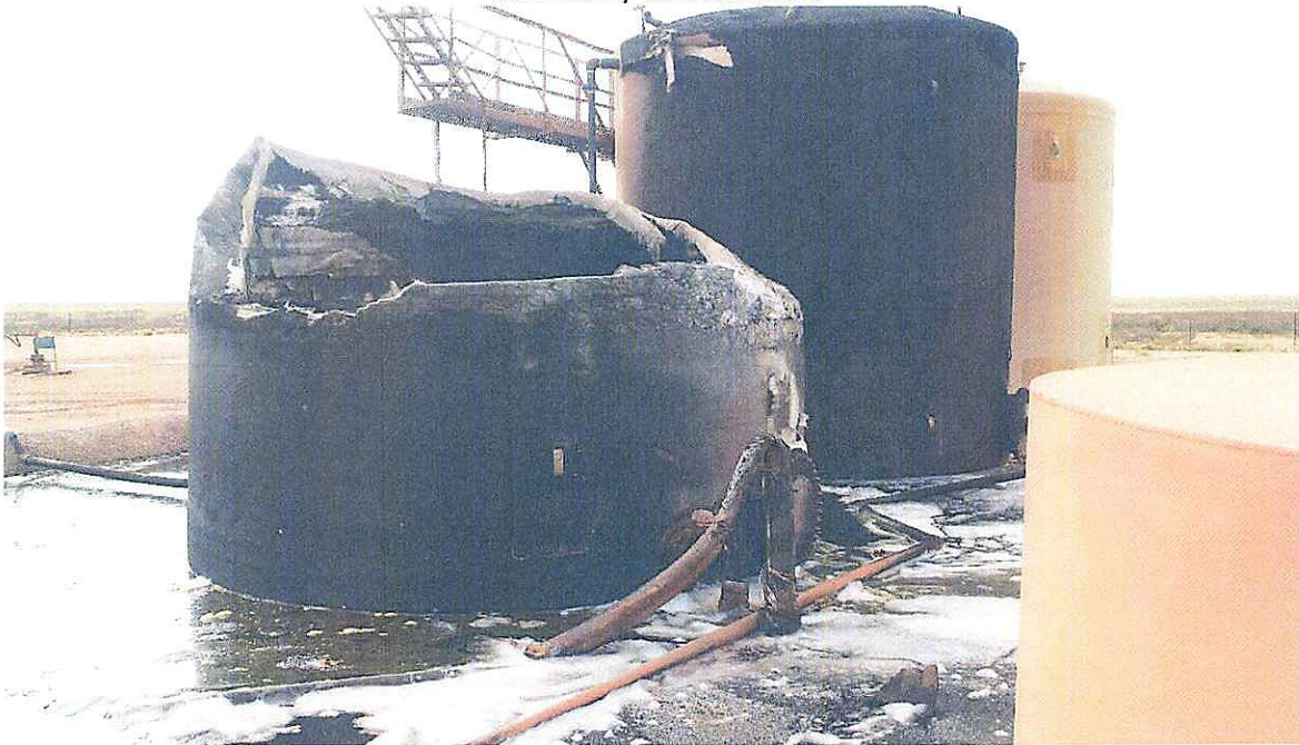
Photograph 1: Burned Production Water Storage Tanks and Standing Water in Lined, Bermed Secondary Containment
