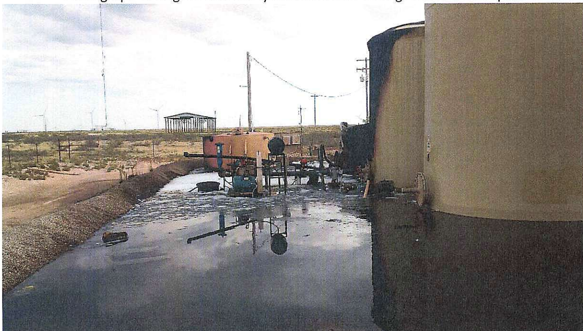
Photograph 2: Original Secondary Containment Holding All Released Liquids
