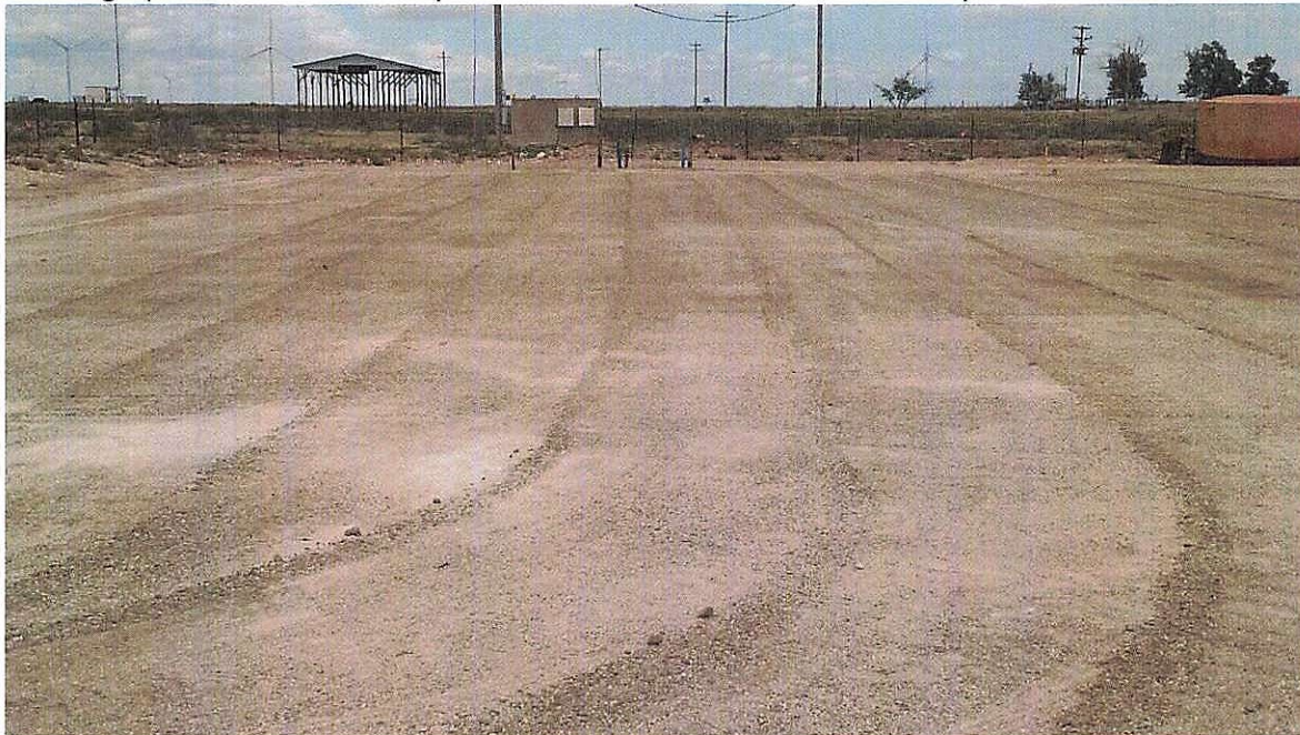
Photograph 6: Pad Surface Prepared for Installation of New Secondary Containment Structure
