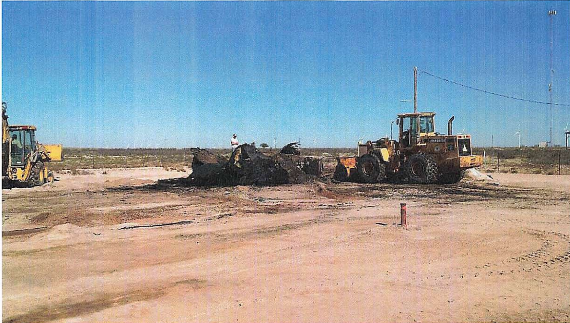
Photograph 5: Removal of Secondary Containment Liner and Berm to Make Way for New Secondary Containment Structure
