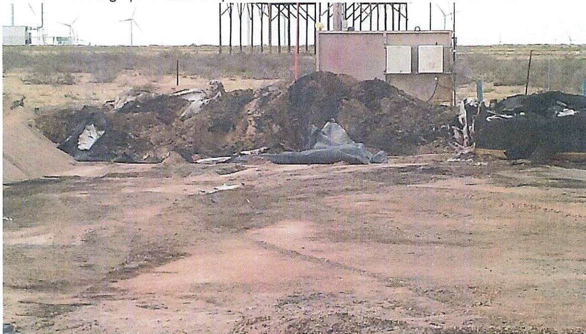
Photograph 4: Secondary Containment Liner and Earthen Berm Removed
