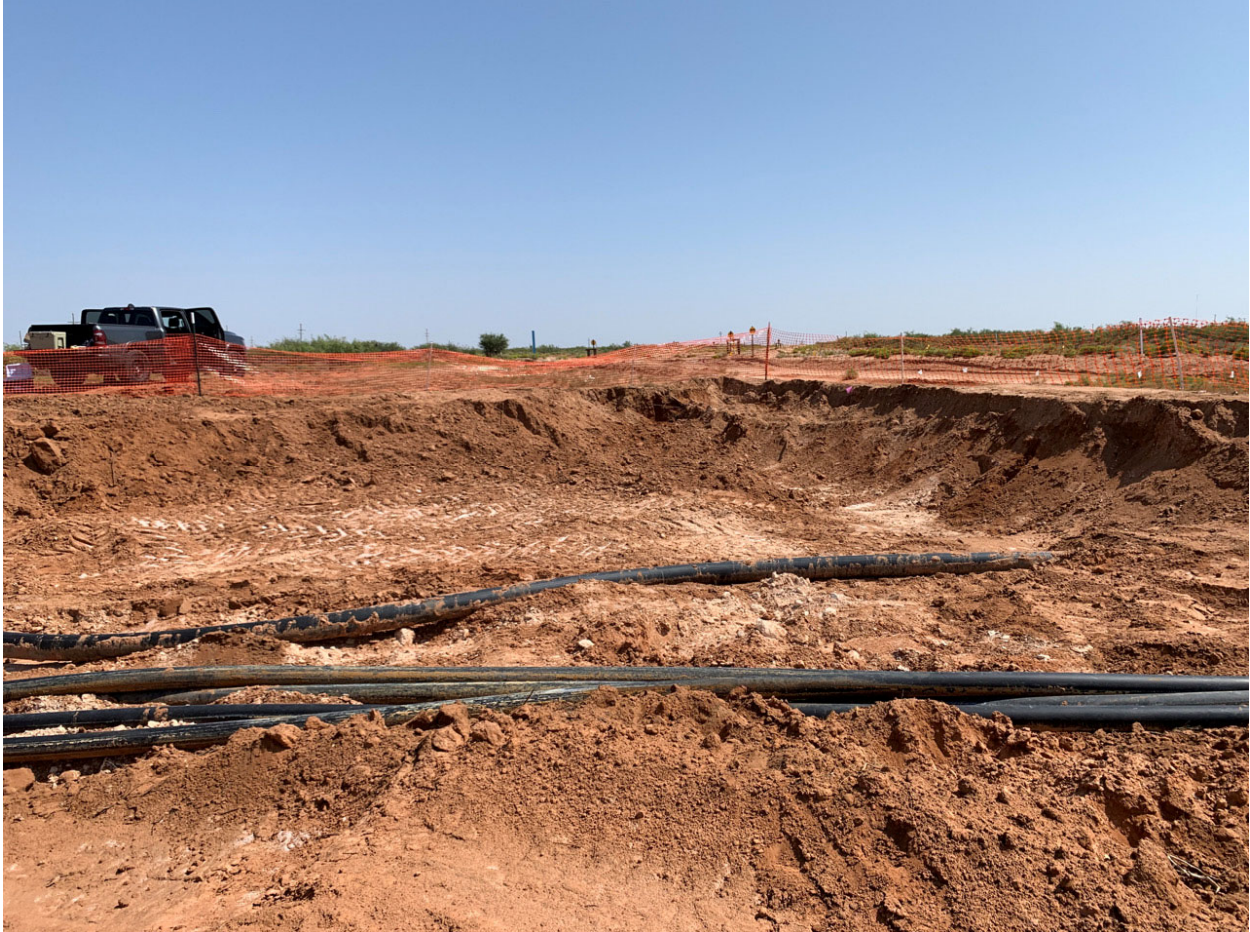
Excavation Facing East
