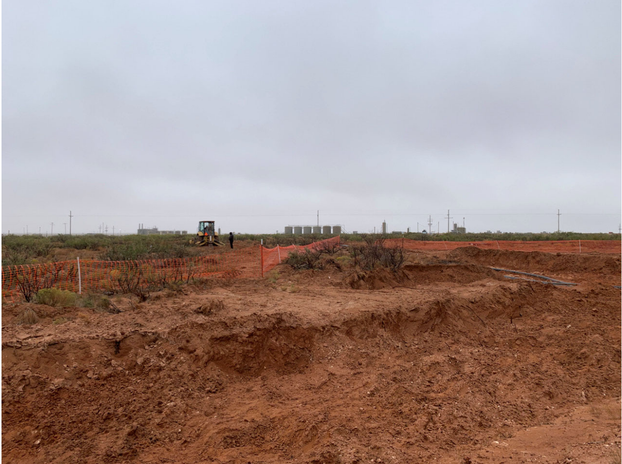
Excavation Facing North
