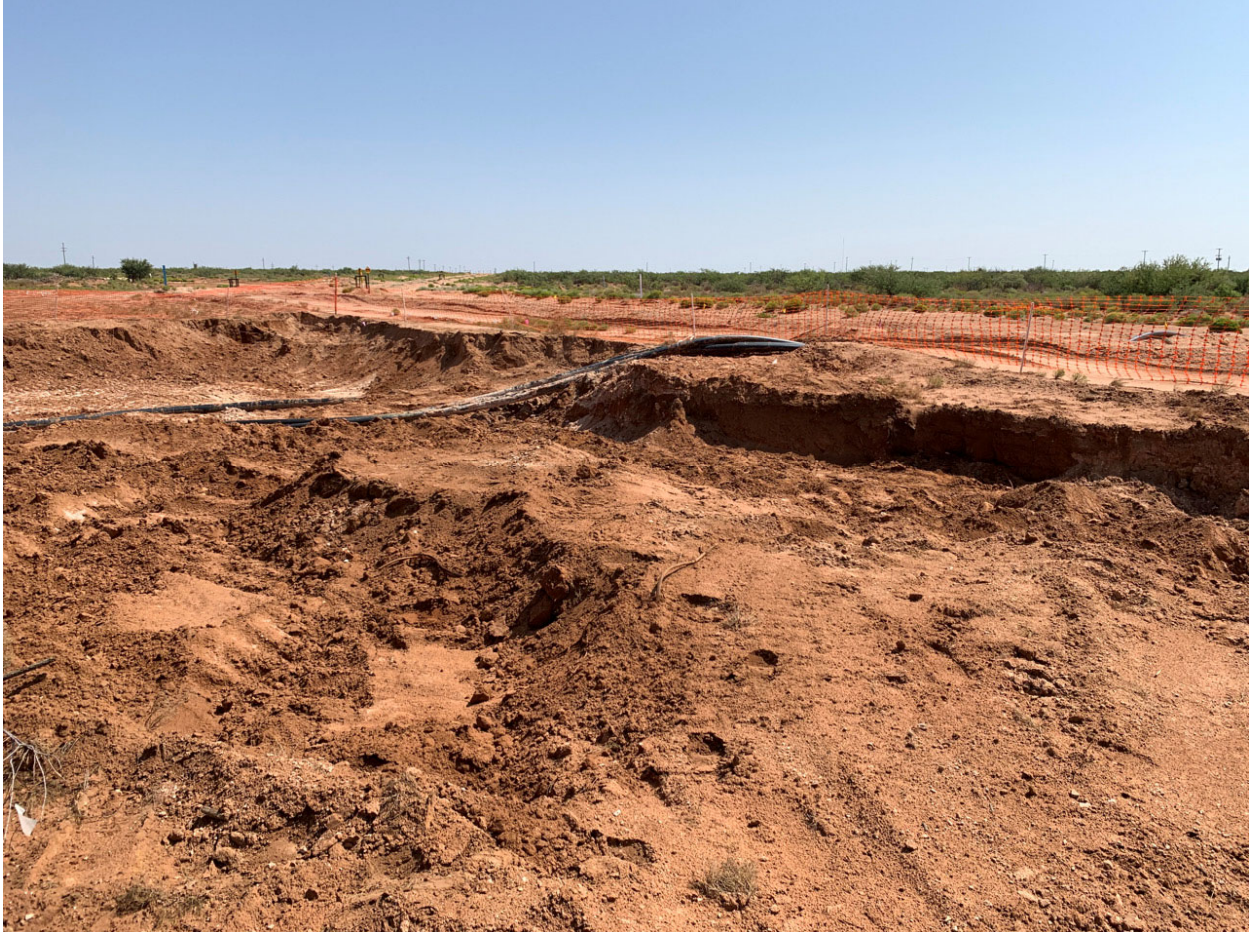
Excavation Facing South
