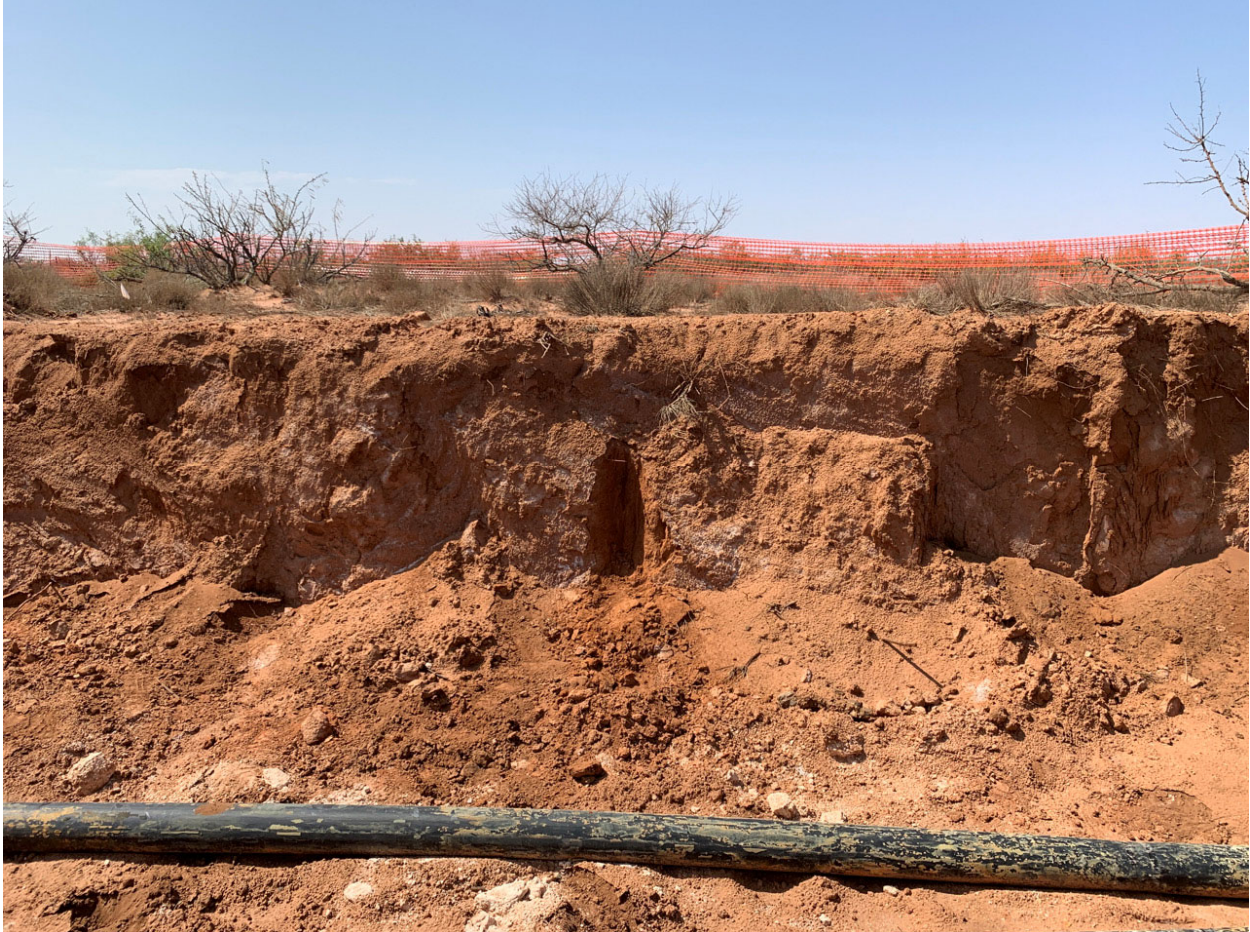
Excavation Facing West
