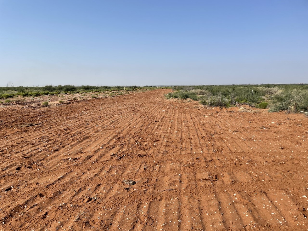
Backfill on Location
