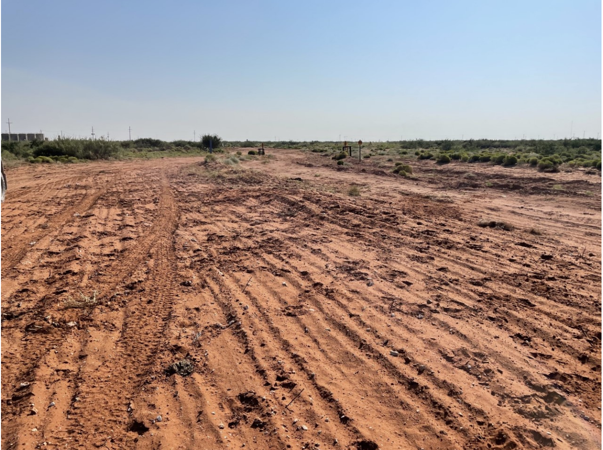
Backfill on Location
