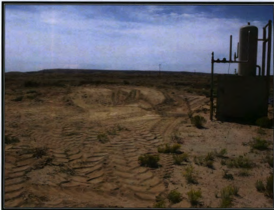
Photo 2: Excavated Area After Backfilling and Recontouring
