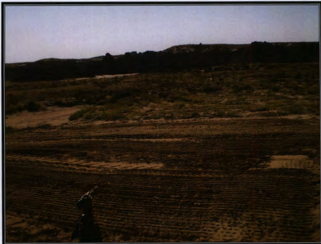
Photo 2: Excavated Area After Backfilling and Recontouring
