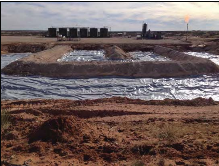
Geomembrane cover over stabilized cuttings 12/29/2014
