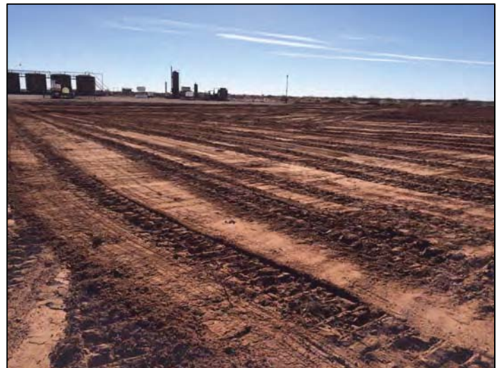
Backfill complete (facing southwest) 1/20/2015
