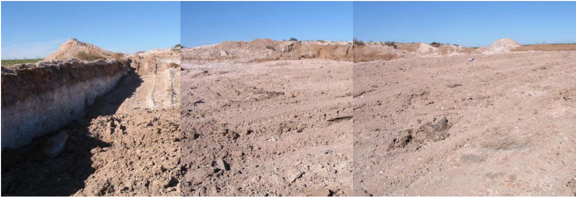
Figure 1: View to northwest and northeast of stabilized material on October 14, 2014. Surface of stabilized material is 4-feet below ground surface.
