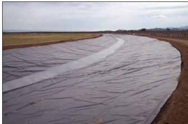
Irrigation Canal Liner
