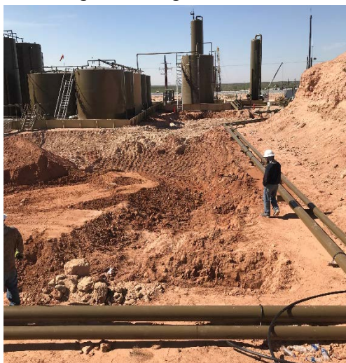
Photograph 5: South facing view during excavation activities.
