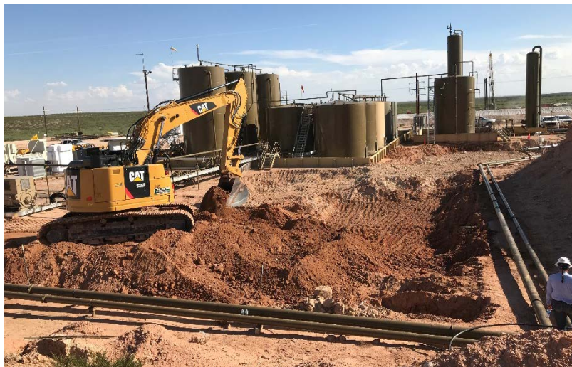
Photograph 4: South facing view during excavation activities.
