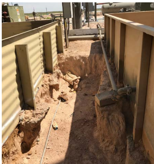
Photograph 3: View of open excavation between containments.
