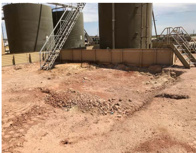
Photograph 2: Southeast facing view during excavation activities.
