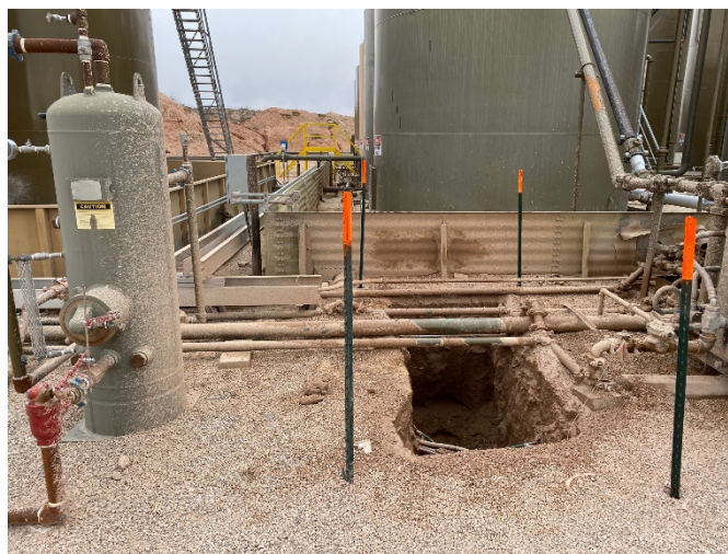
Photograph 6: North facing view of excavation south of containment.
