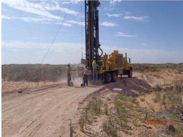
Drilling SB-2, facing southeast
