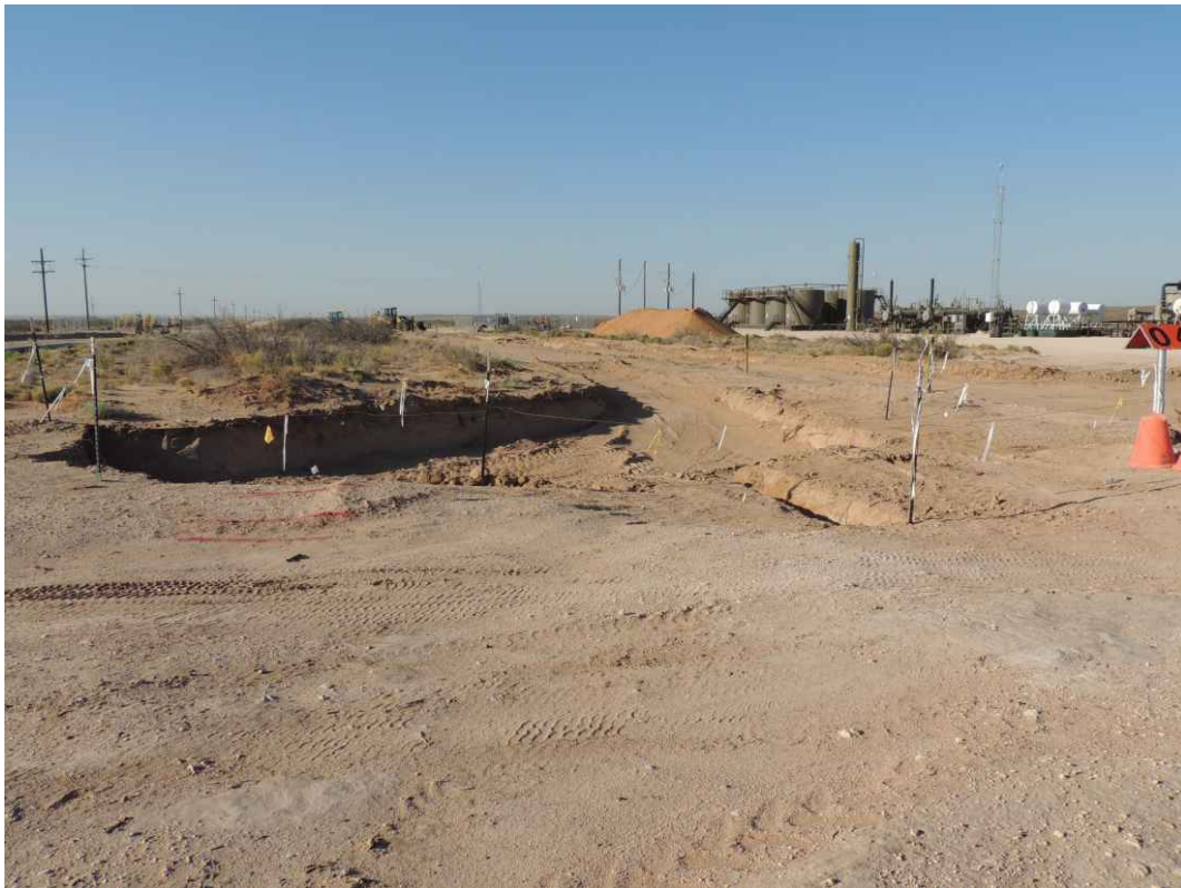
View South – Excavation Area of AH-2
