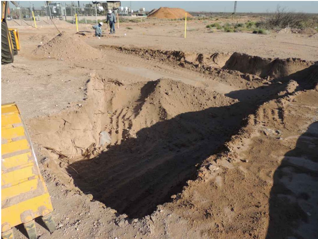
View Northwest – Deeper Excavation near AH-8
