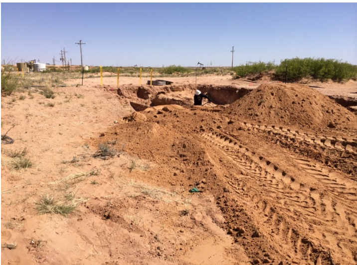
Backfilling of lined area 5/2/14
