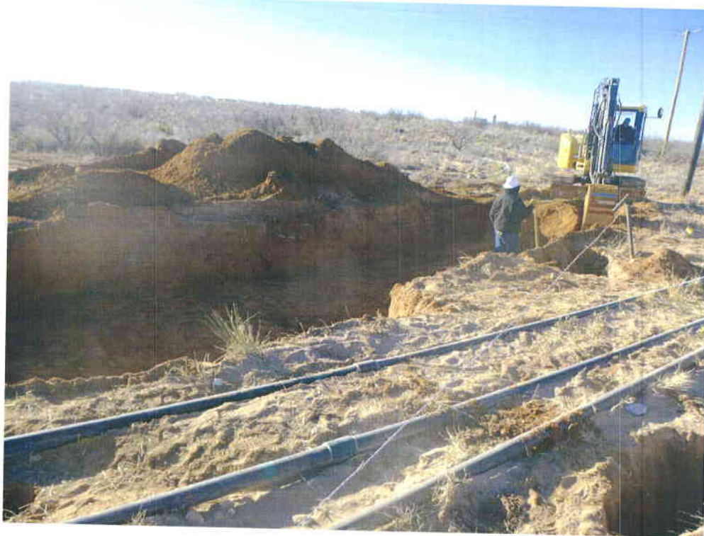
Excavation of impacted area north leg of the flowline
