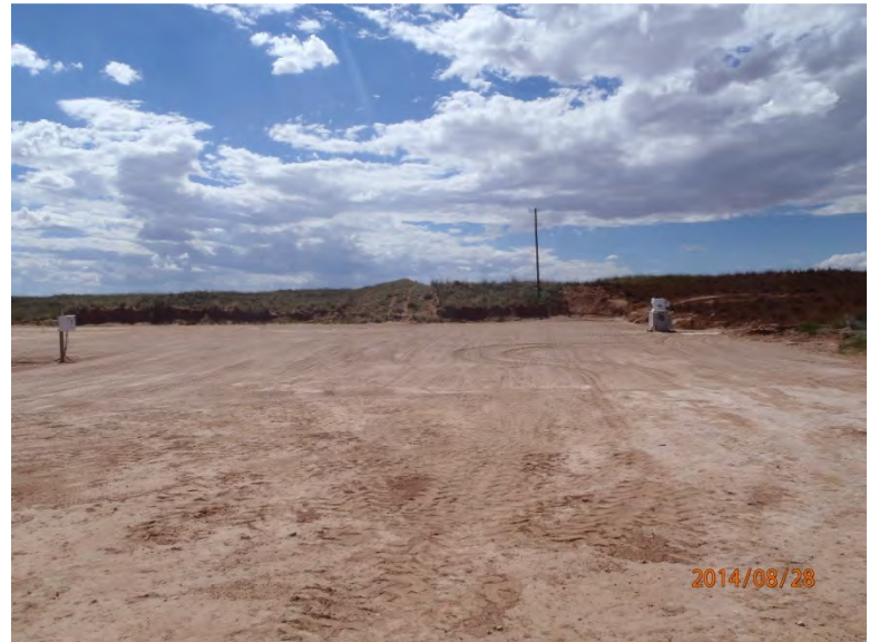
Scrape of pad completed, facing west 8/28/14
