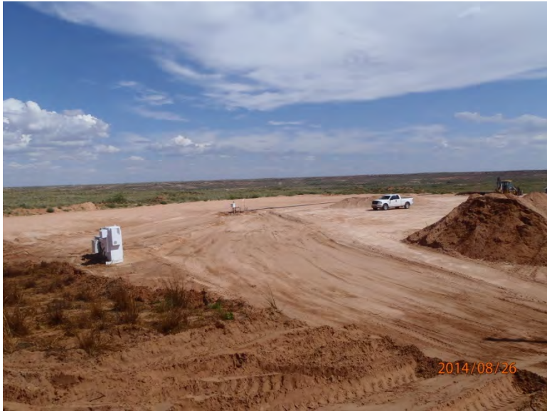
6 inch scrape completed, facing southeast 8/26/14
