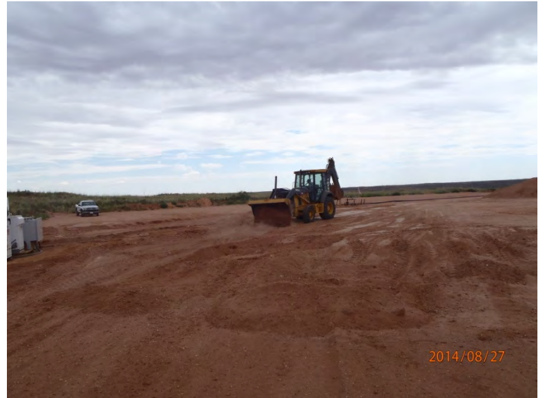
Backfilling scrape, facing southeast 8/27/14
