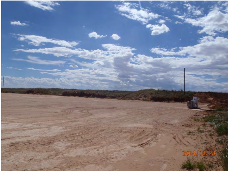
Scrape of pad completed, facing southwest 8/28/14
