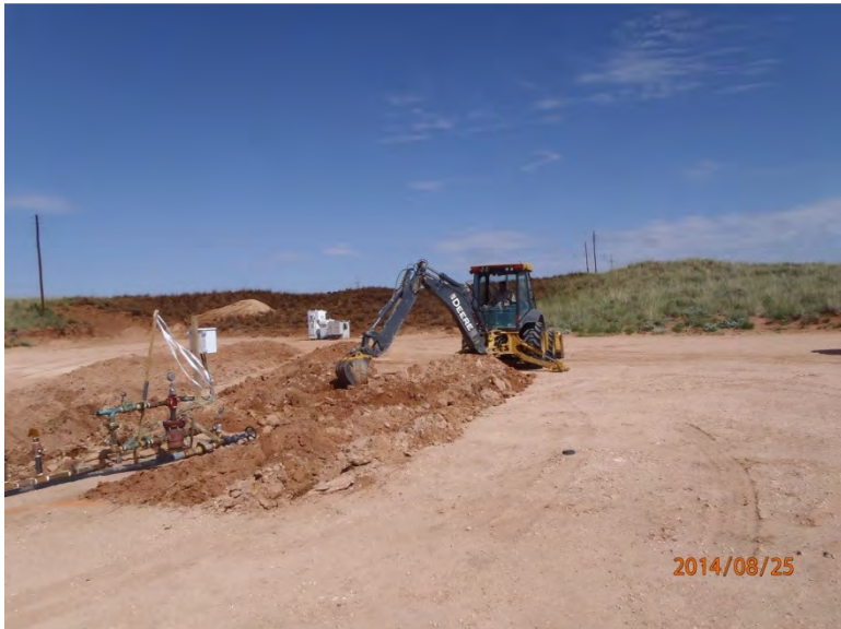
Scraping pad to 6 inches bgs, facing northwest 8/25/14
