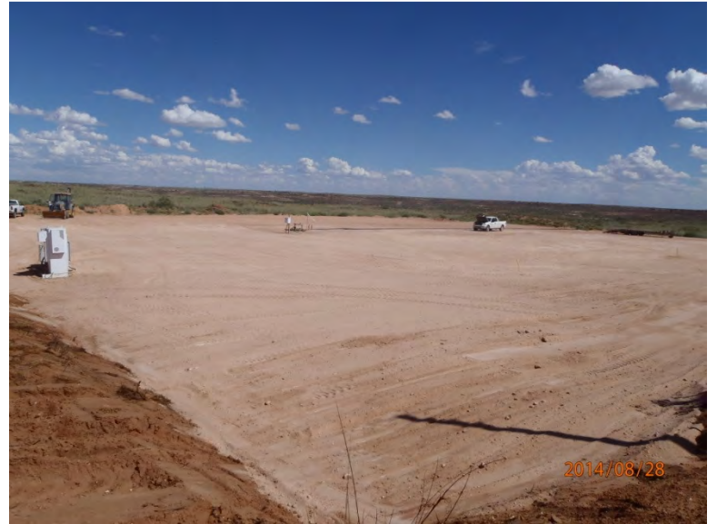
Scrape of pad completed, facing southeast 8/28/14
