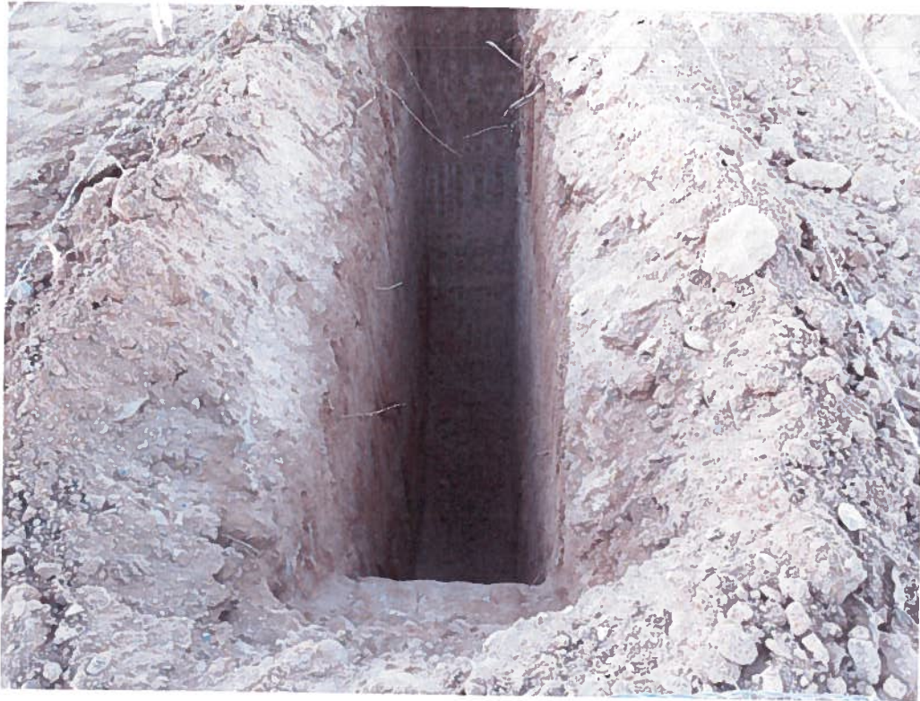
View East – T-1 in Area of AH-1
