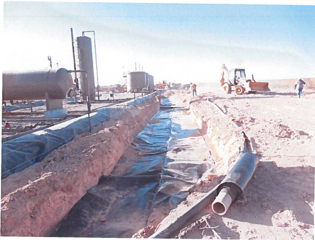
View South – Areas of AH-1 and AH-2 with Liner Installed
