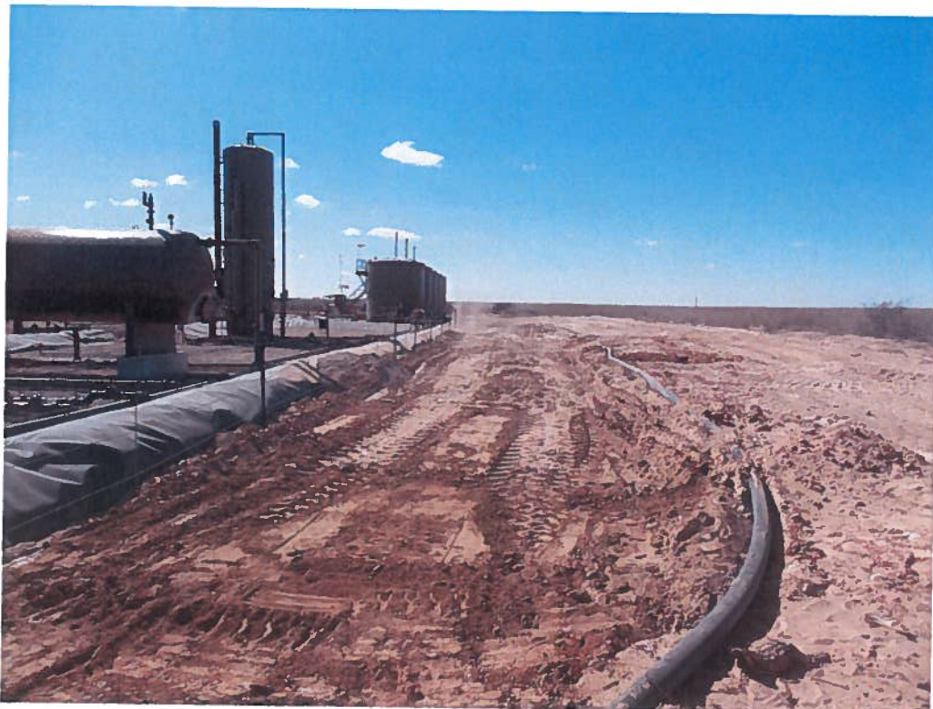
View South – Excavation Backfilled
