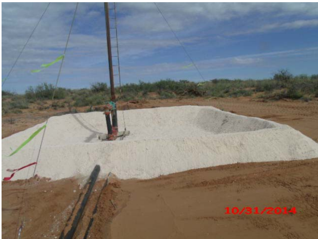
Photograph #9 – Berm rebuilt around flare
