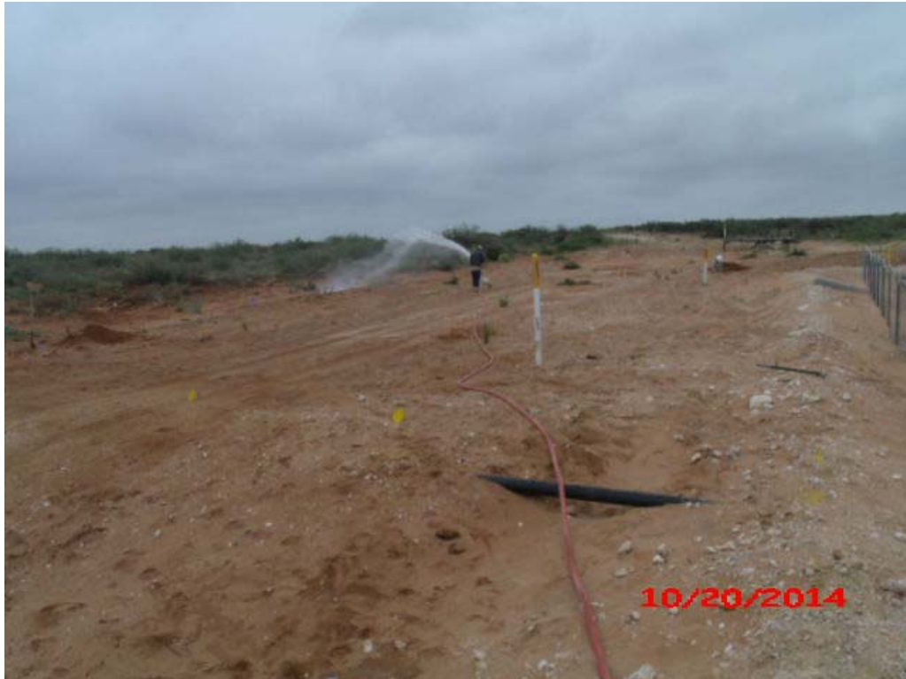
Photograph #5 – Application of Micro-Blaze
