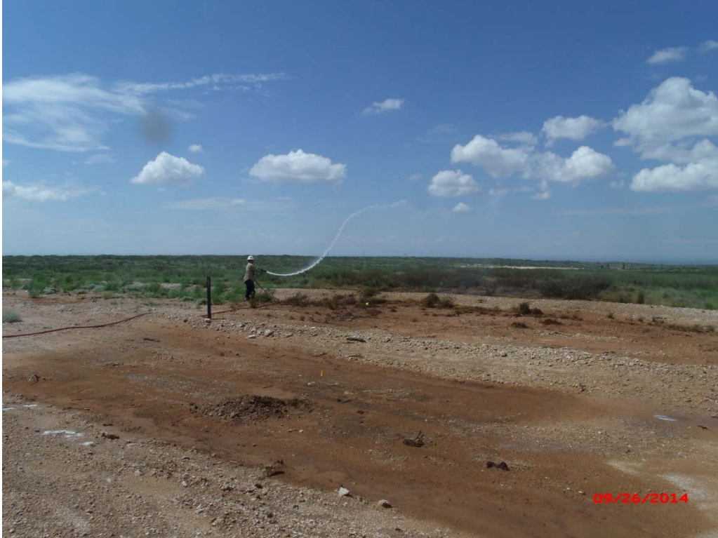
Photograph #5 – Application of Micro-Blaze
