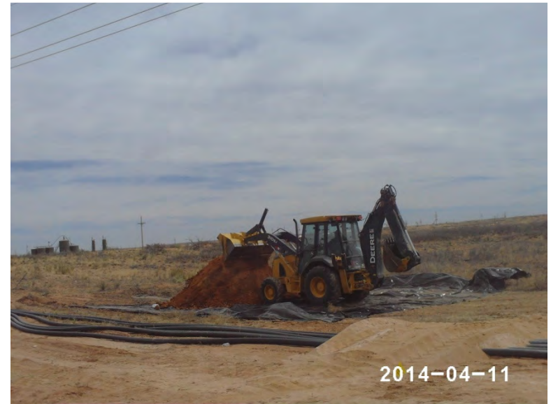
Place soil pile on plastic, facing northeast 4/11/14
