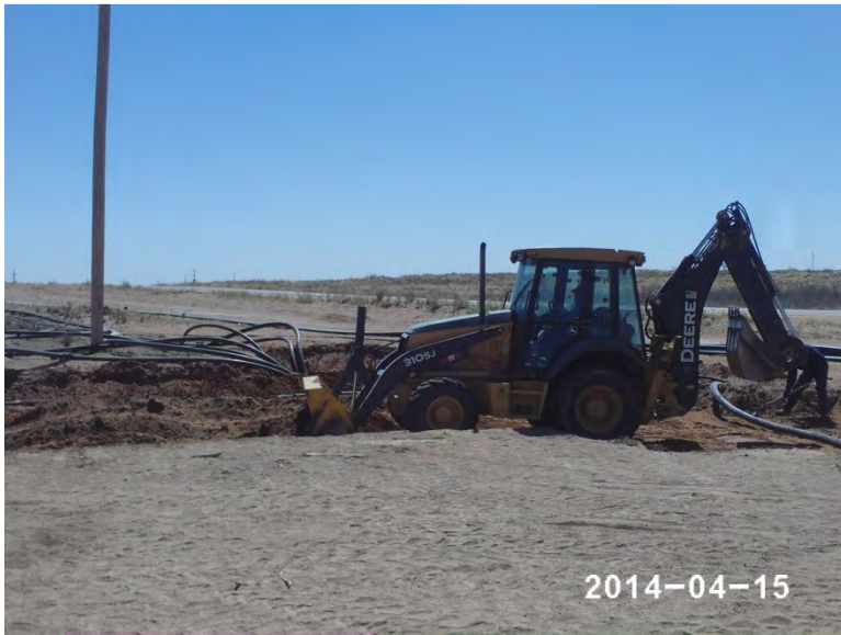
Scraping site down to 1.5 ft bgs, facing southwest 4/15/14
