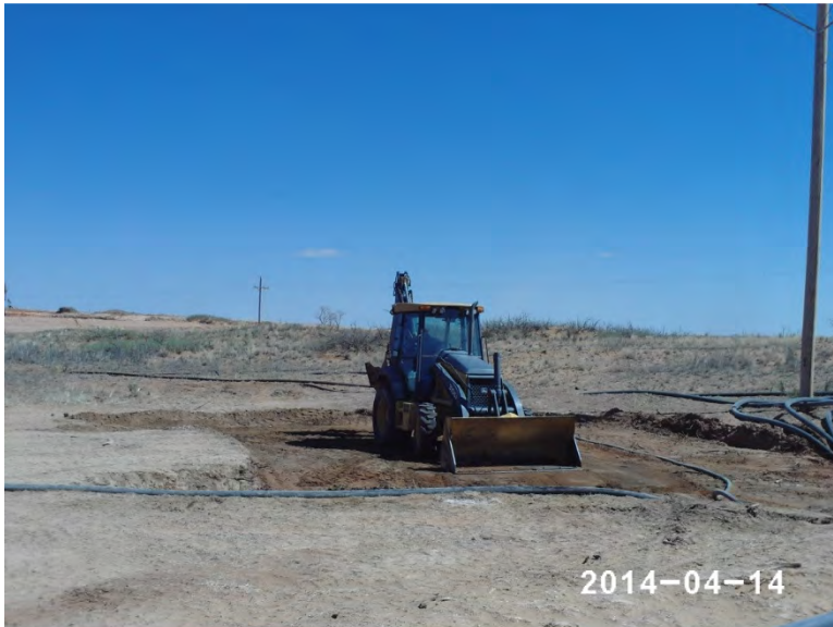
Scraping site down 1 ft bgs, facing east 4/14/14
