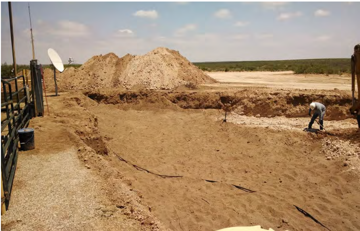
Indian Flats Bass Federal SWD – Excavation & Exposure of Existing Liner (Looking East-Southeast)
