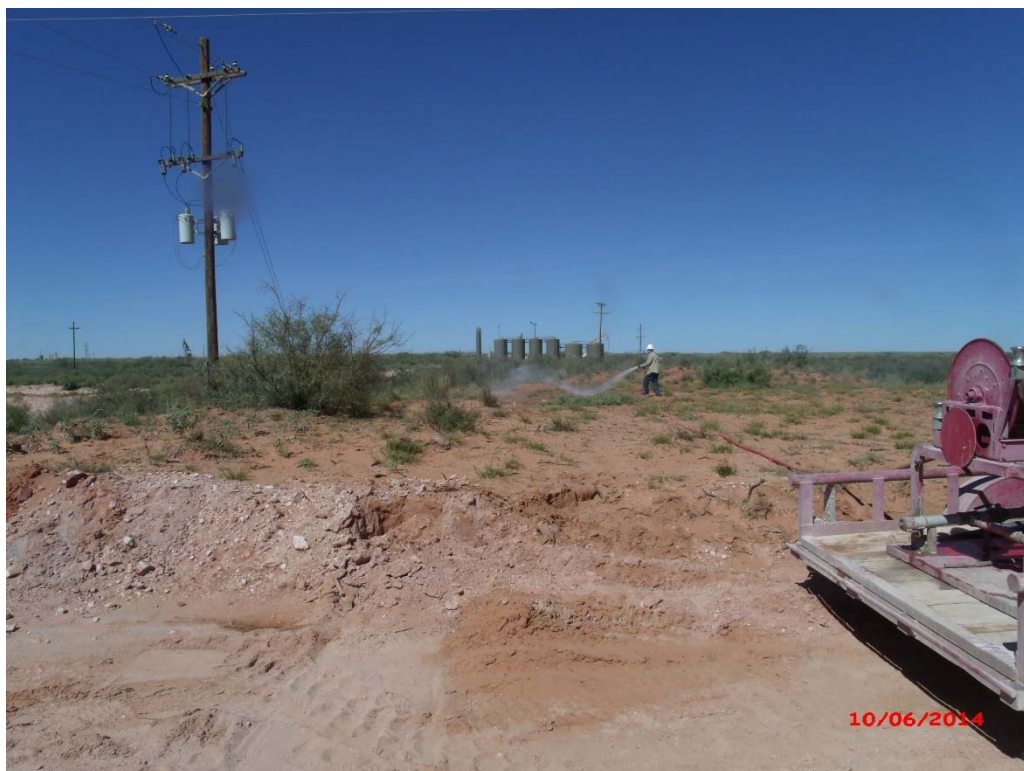
Photograph #2 – Application of Micro-Blaze
