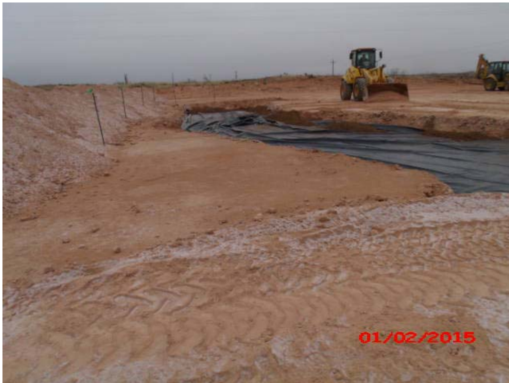
Photograph #11 – Liner installed
