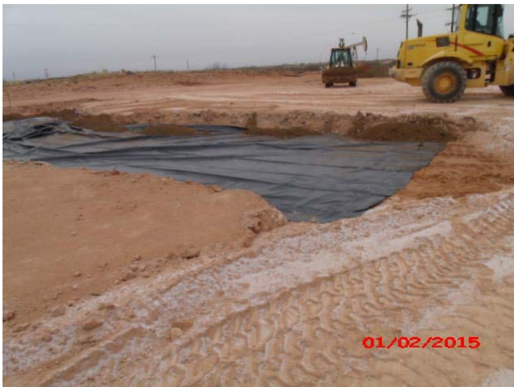
Photograph #12 – Liner installed
