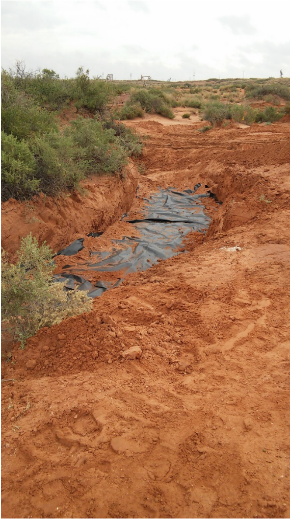
Spill area excavated with liner installation
