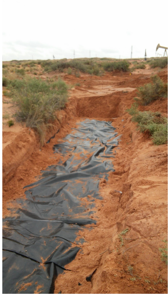
Spill area excavated with liner installation
