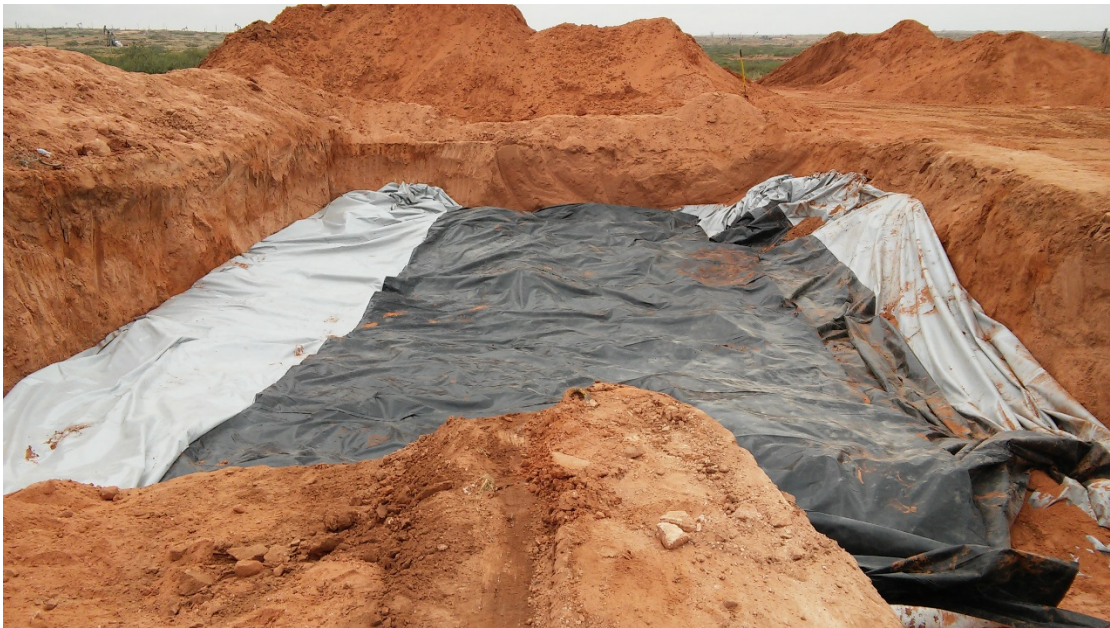
Pit area on Turner B 96 dug out and placed with liner
