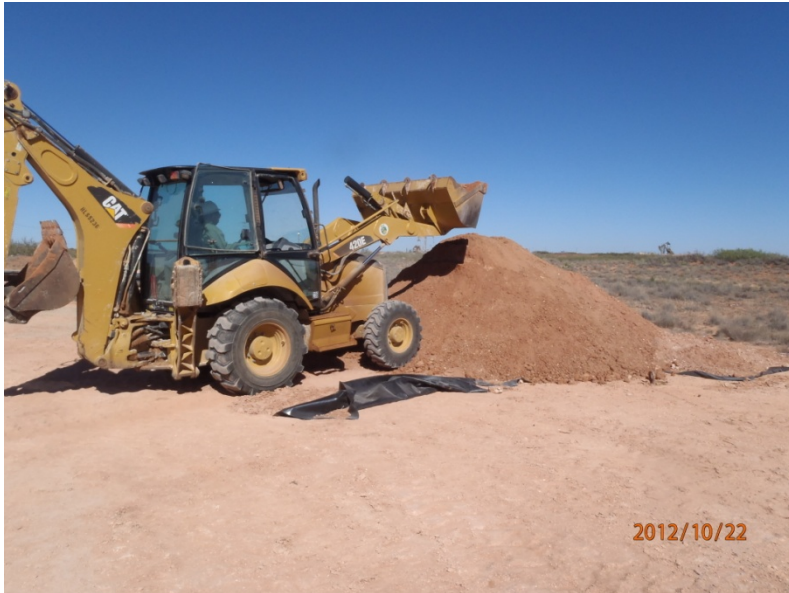
Stockpiling on plastic, facing east
