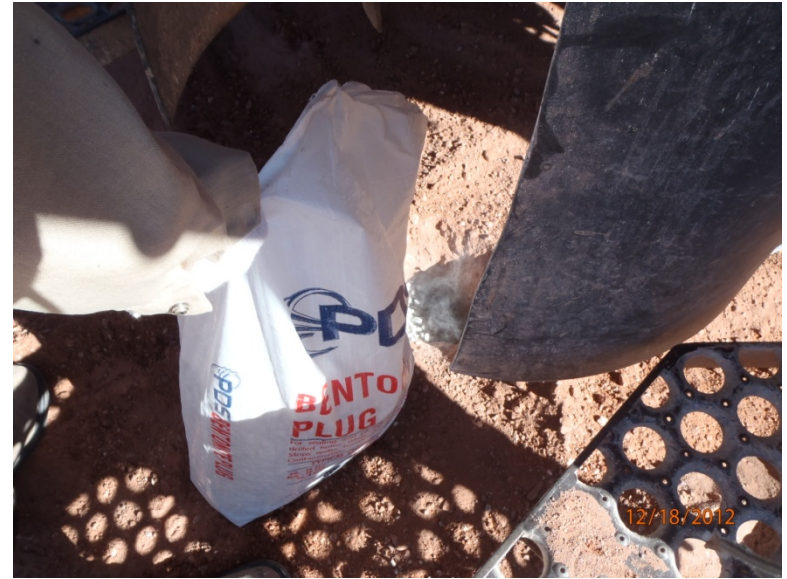
Plugging SB-1 in total with bentonite
