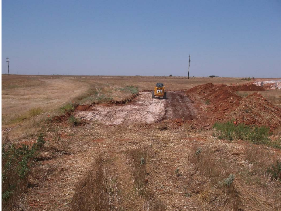
Photograph 5: Incorporating gypsum into base of the excavation
