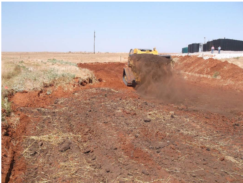
Photograph 4: Incorporating manure into base of the excavation
