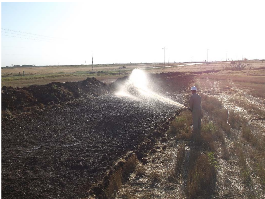
Photograph 6: Treating the base of the excavation with a MicroBind solution
