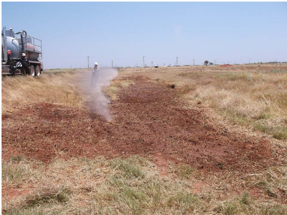
Photograph 2: Treating the tilled drainage way with a MicroBind solution
