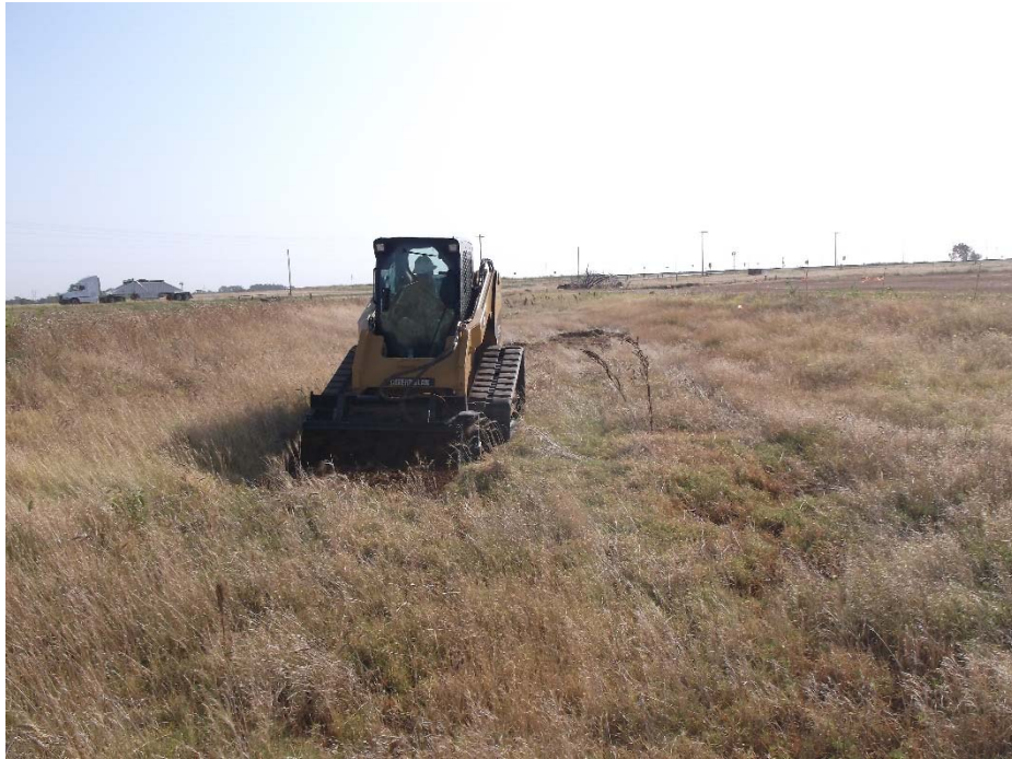
Photograph 1: Tilling drainage way
