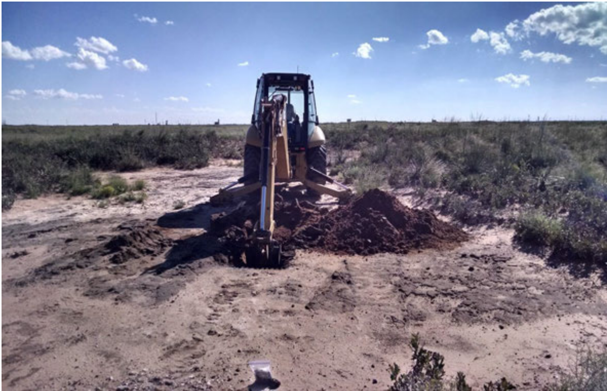
Former Maljamar Station – Advancement of Delineation Trench TT-10 (looking southwest)
