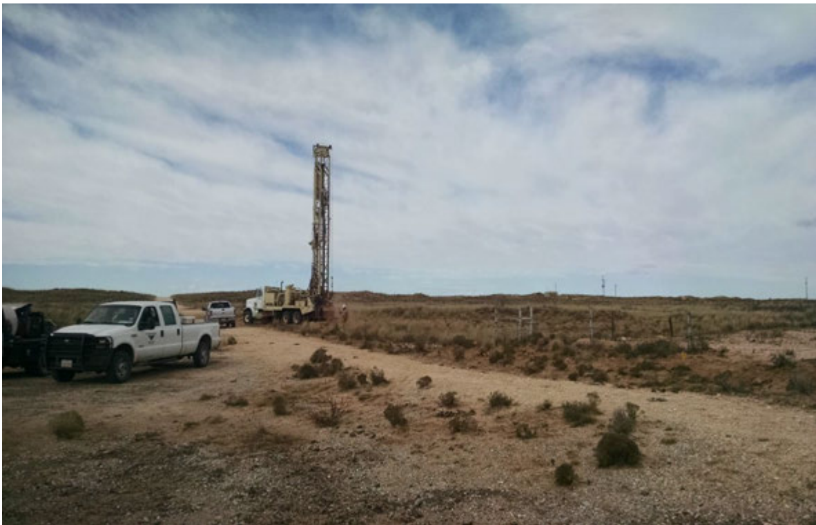
Former Maljamar Station – Advancement of Soil Boring SB-5 (looking northwest)
