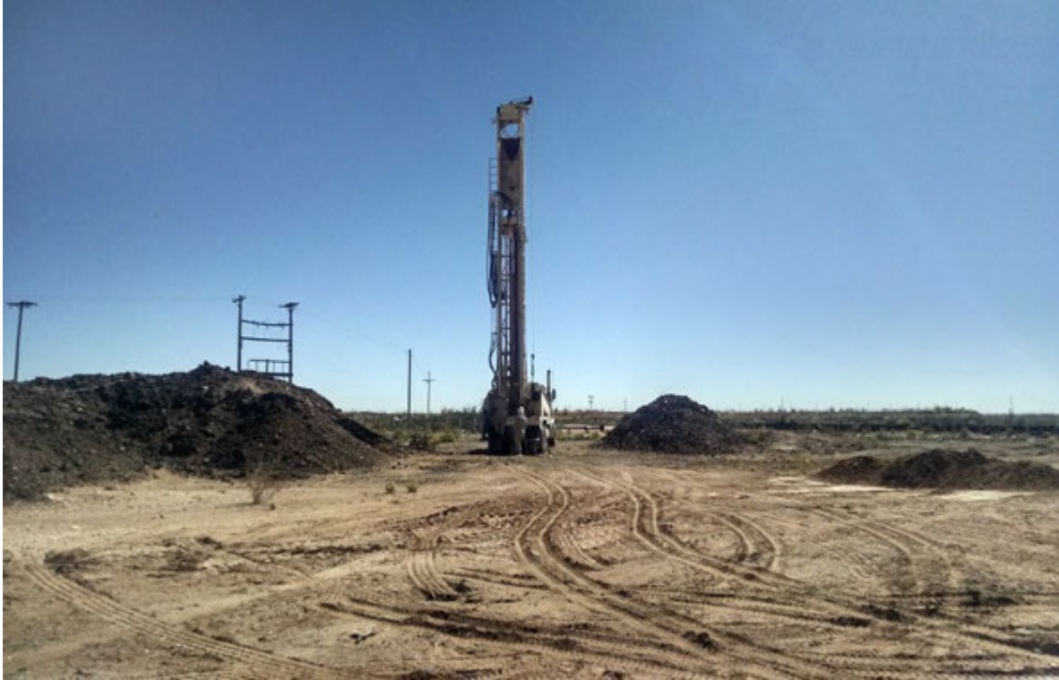
Former Maljamar Station – Advancement of Soil Boring SB-2 (looking south-southeast)
