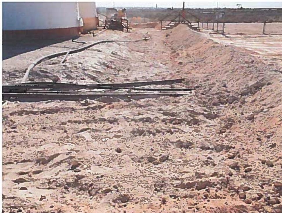
View South – Backfill of AH-1 Excavation.
