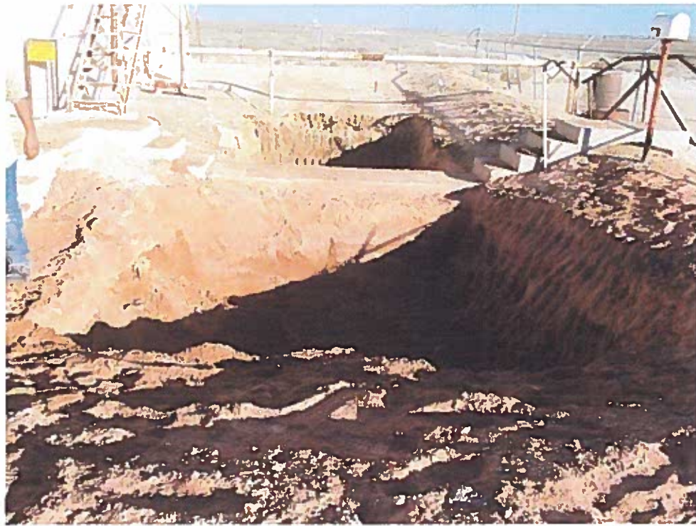
View East – Excavation of AH-6.
