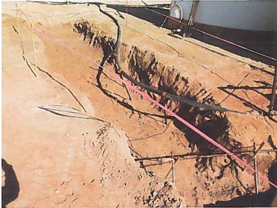
View North— Excavation of AH-1.
