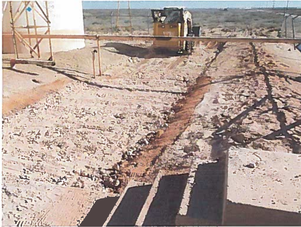
View East – Backfill of AH-5 and AH-6 excavations.
