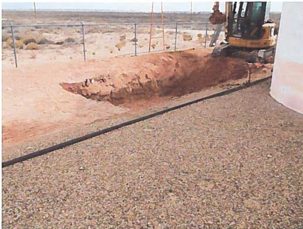
View Southeast – Excavation of AH-4.
