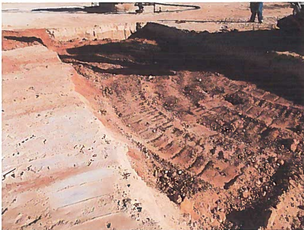
View Northeast – Clay Cap added to Excavation.
