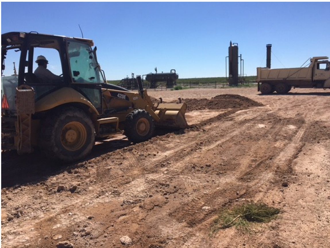
Excavation of the spill area via backhoe
