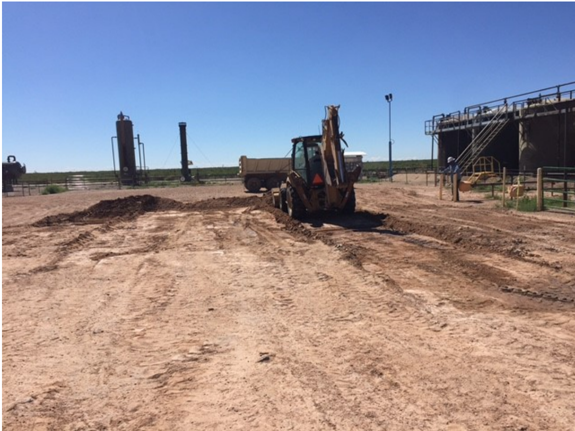
Excavation of the spill area via backhoe
