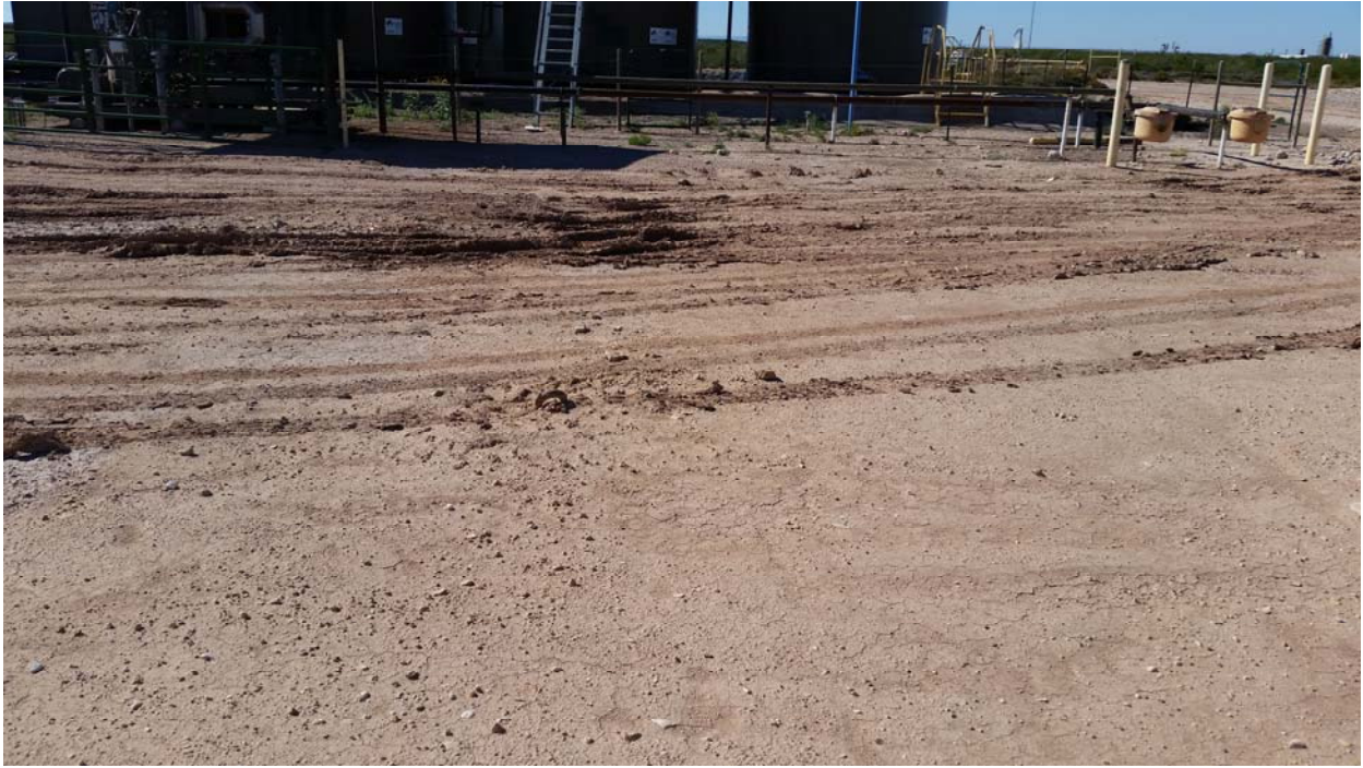
View of the backfilled area
