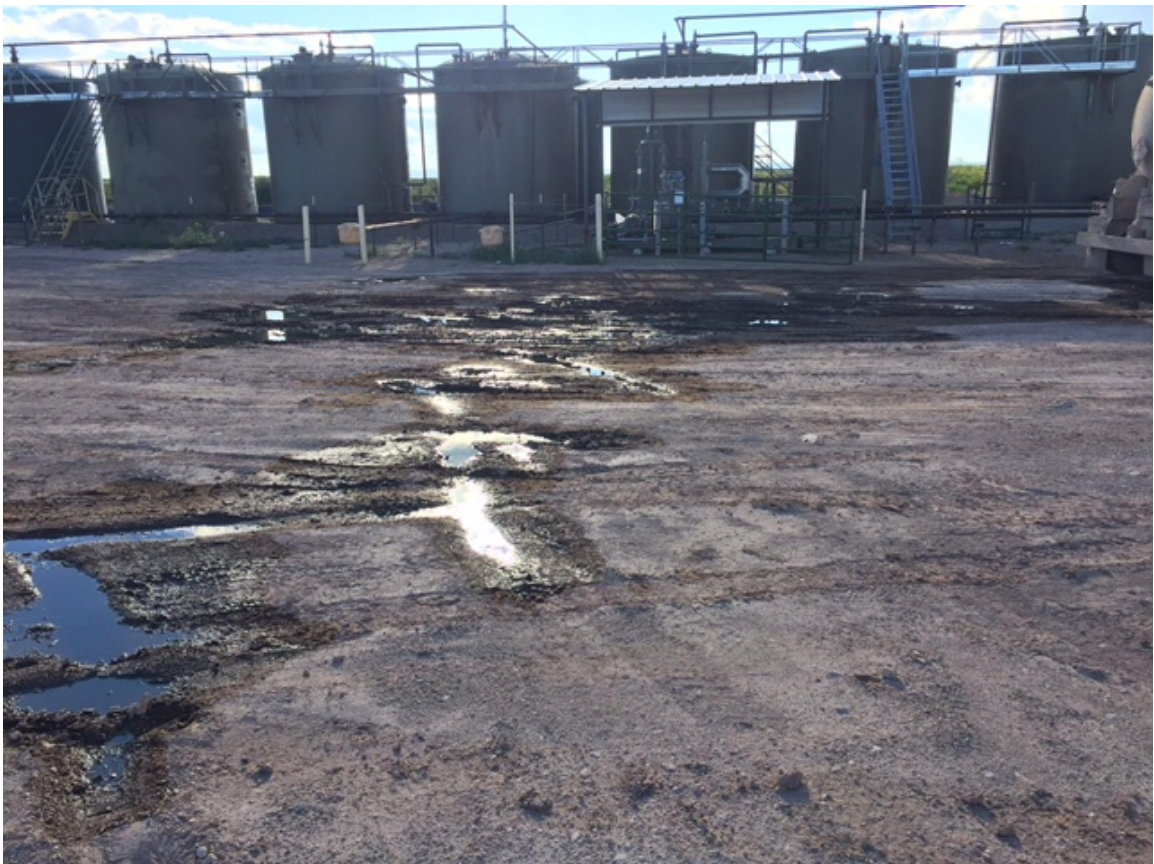
View of the crude spill area
