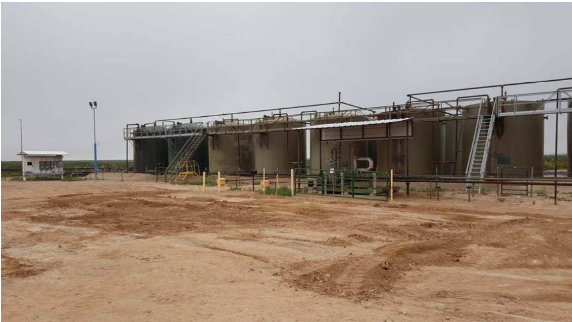
View of the excavated area
