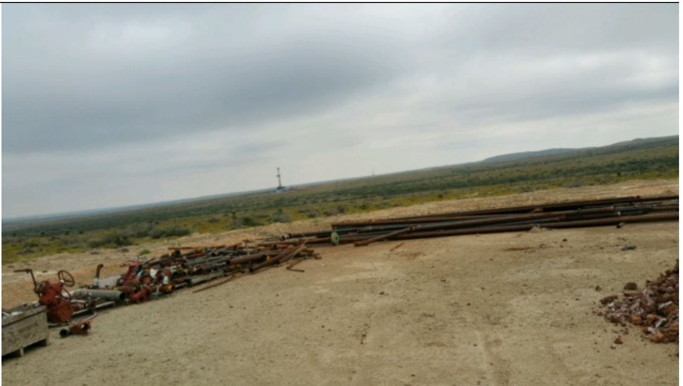
Photo 2: View of portion of the affected production pad, facing northeast.
