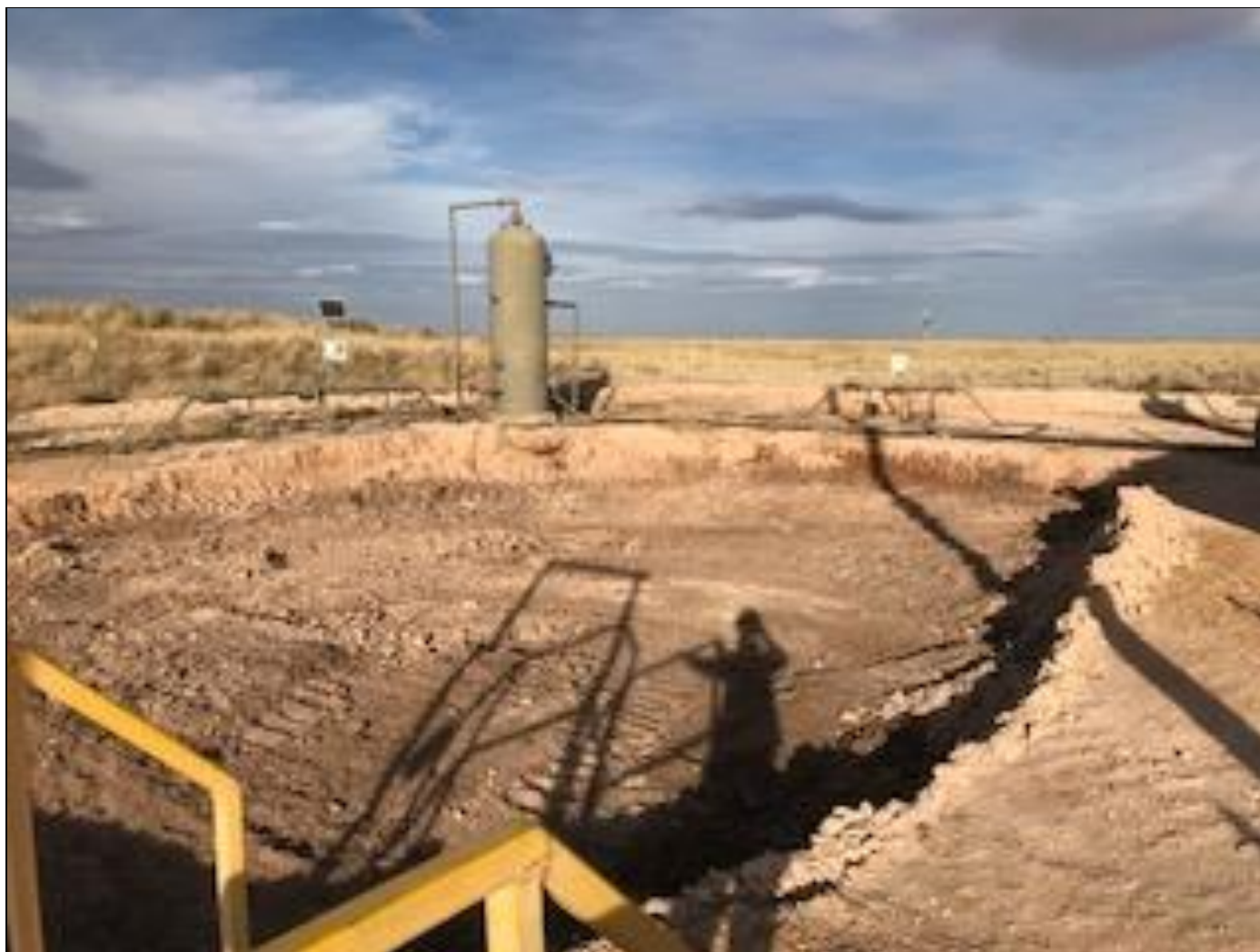
View of excavation facing northeast toward pasture.
