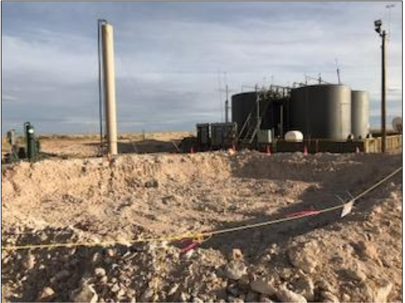
View of excavation facing south toward tank battery.
