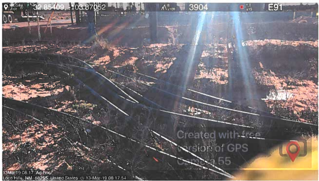
Photo of excavation
